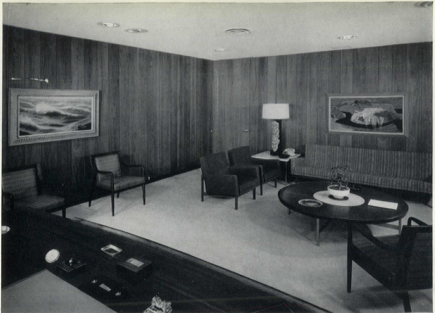
Weldwood® plain sliced 3/4" Architectural walnut , installed in a carefully mismatched plank style. Office of the president, Southland Life Insurance Company, Southland Center, Dallas. Arch: Welton Becket, FAIA & Assoc., Los Angeles. Inst: Adleta Show Case & Fixture Mfg. Co., Dallas.
