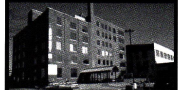
CIGAR FACTORY Architect: Joel Kranich Architect, P.C. HVAC: ClimaTech
