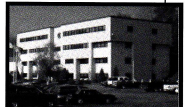
BLACKBOX DISTRIBUTION CENTER Architect: WTW Architects HVAC: ClimaTech
