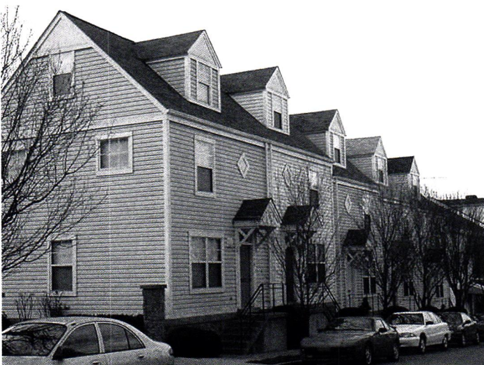
The active South Side Local Development Corporation has 72 units of housing to their credit with eight more underway. Design review is critical. "We're like design Nazis over here," says director Carey Harris.
