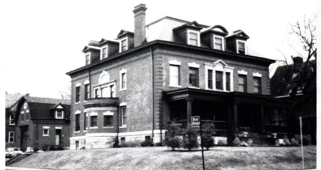
A project of Highland Park Community Development Corporation and Bloomfield Garfield Corporation, this $1.4 million restoration of an abandoned building on Stanton and Mellon is now an 11-unit apartment building. The group credits the Community Design Center of Pittsburgh as instrumental in assisting with the project. Architect: Korzeniwsky-Cullen.
