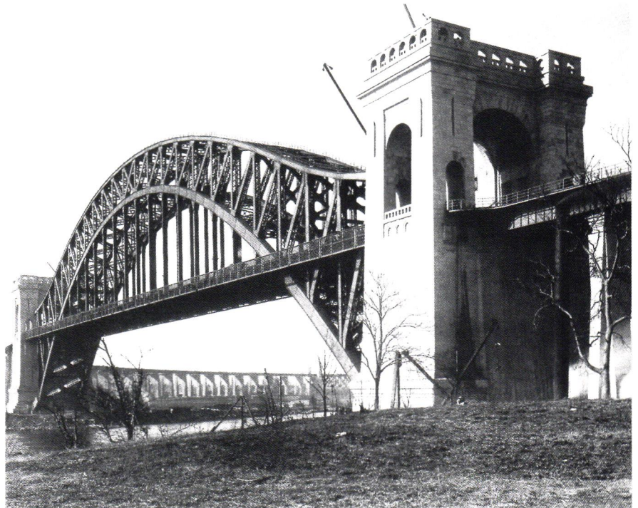
Hell Gate Bridge, New York, NY. At the time of its completion, Hell Gate was the longest steel arch bridge in the world. Hornbostel was the first architect to collaborate with engineers on bridge design.
