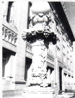
Detail of lamp and terra cotta ornament, City Hall, Oakland, California. Kidney observes that from competition entry to execution the ornament went from classical to almost Art Nouveau.
