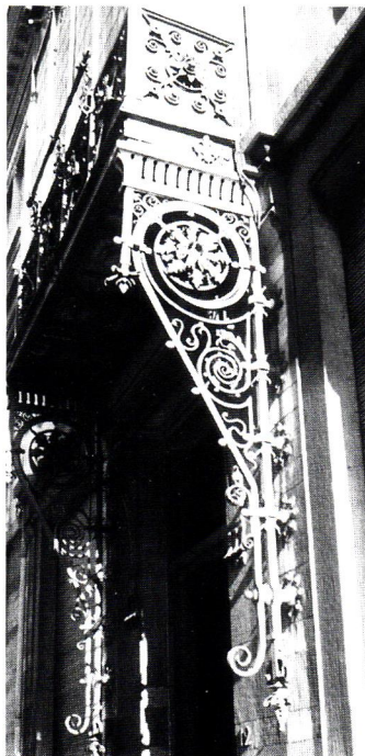
A sunroom in Brussels, Belgium (circa 1900) Slit and drifted holes, collars and decorative bolts are used in its construction.
