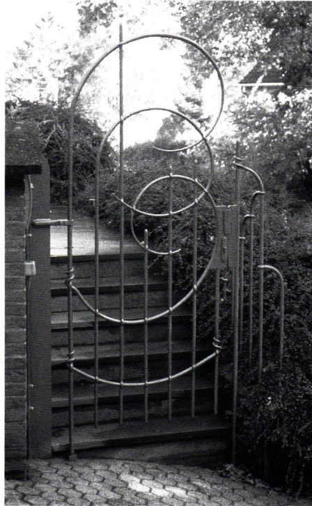
A gate in Eupen, Belgium. There are 25 angled slit and drifted holes used in its construction.
