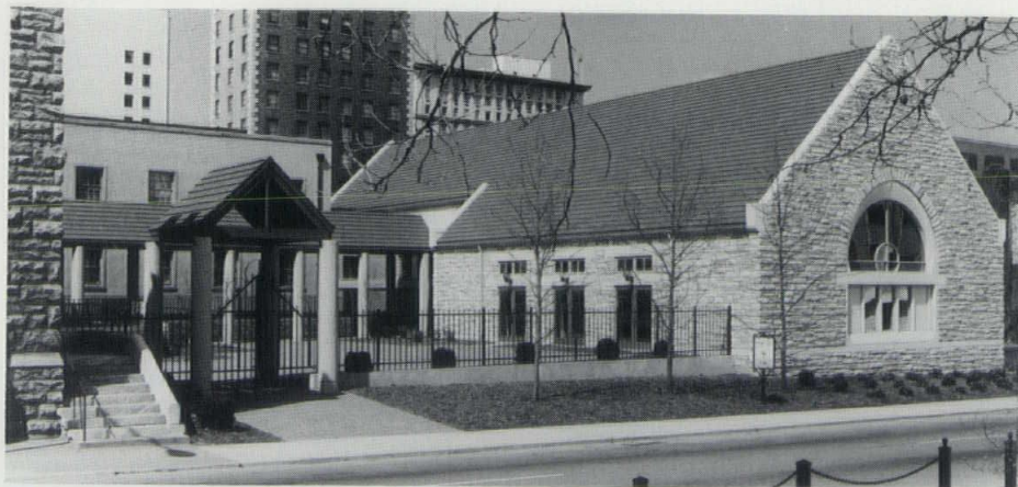
The renovation of St. John's Episcopal Church, across the state in Knoxville, garnered a second award for McCarty, Bullock, Holsaple, who also received a TSA Design Award of Excellence for this fine work. Stone masonry was used to blend in with the existing building, with the material being of reduced scale to meet availability and budget requirements.
