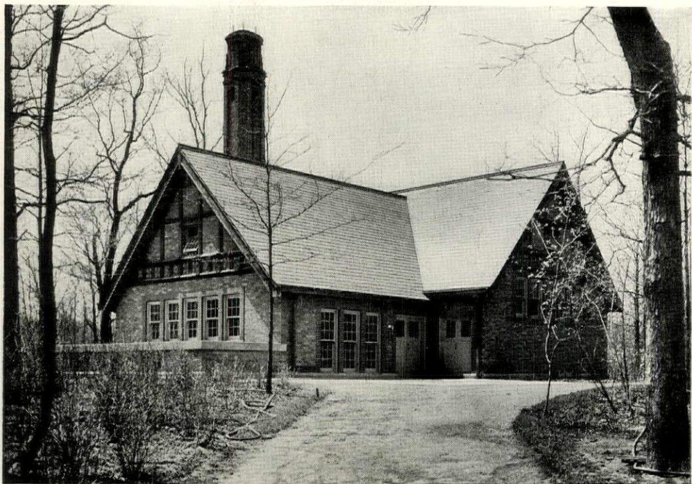
POWER HOUSE—ESTATE OF MRS. CYRUS H. McCORMICK, LAKE FOREST, ILL. Perkins, Fellows & Hamilton, Architects.
