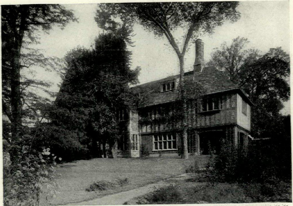
FIG. M. FROM THE SOUTHEAST—RESIDENCE OF ALLAN S. LEHMAN, ESQ., TARRYTOWN, N. Y. John Russell Pope, Architect.
