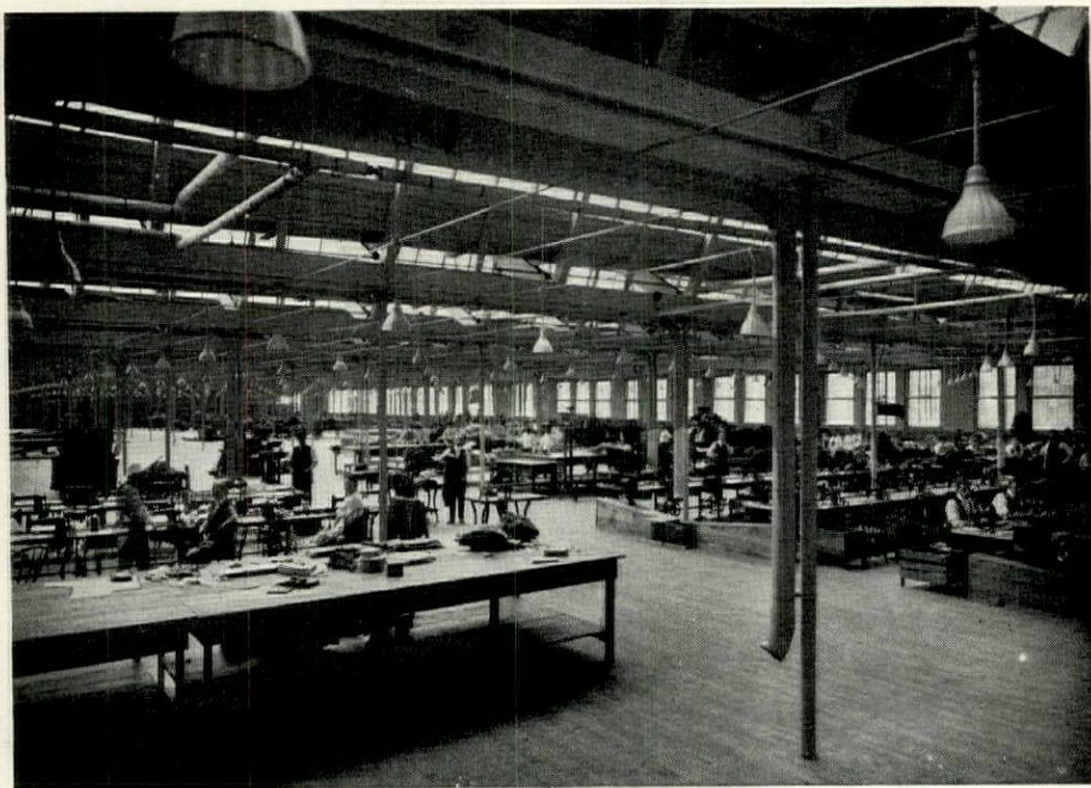
INTERIOR VIEW—ROSENWALD & WEIL BUILDING, CHICAGO. Alfred S. Alschuler, Architect.
