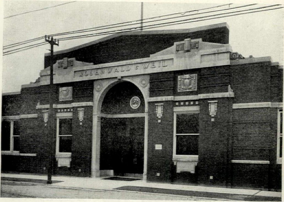
ENTRANCE DETAIL—ROSENWALD & WEIL BUILDING, CHICAGO. Alfred S. Alschuler, Architect.
