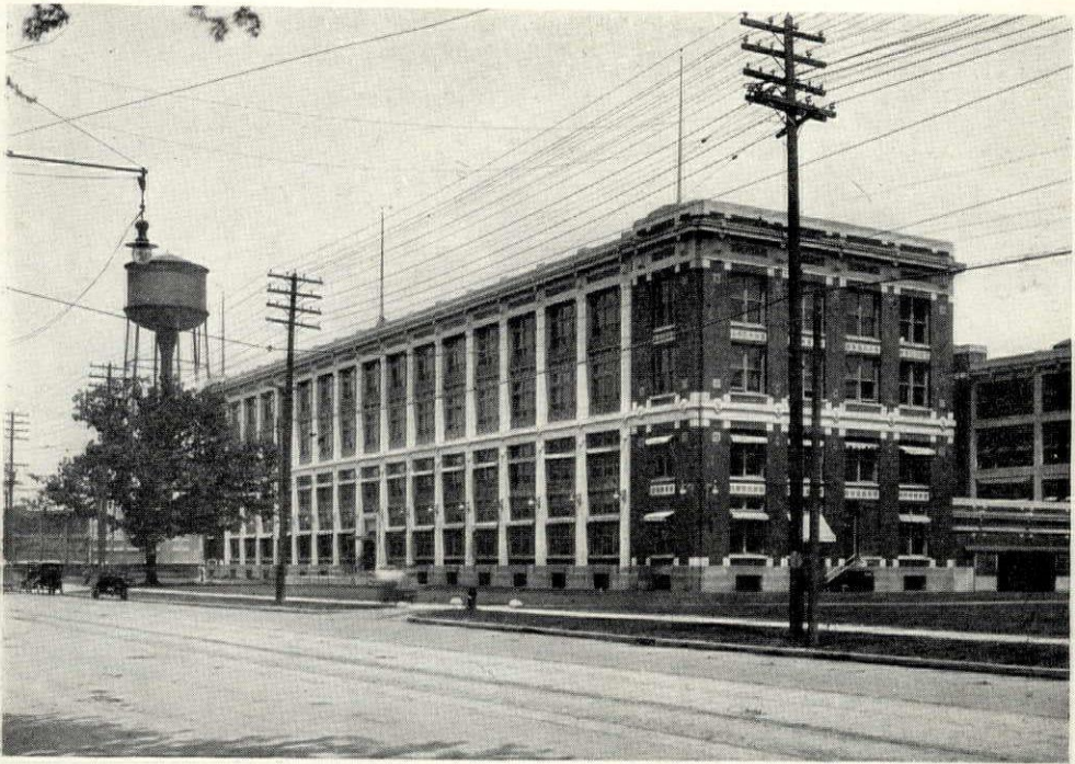
FORD ADMINISTRATION BUILDING, DETROIT, MICH. Albert Kahn, Architect.
