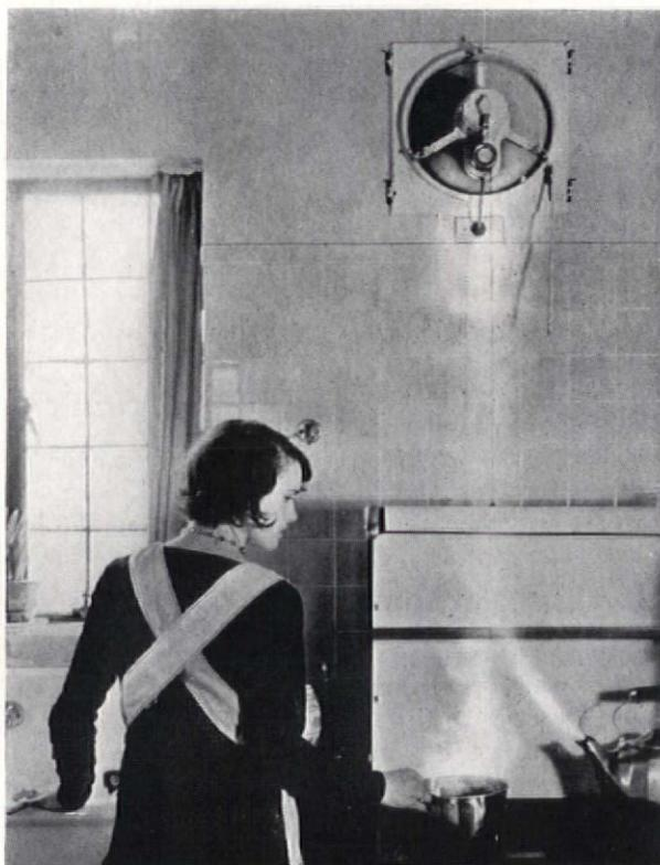
Typical propeller type fan installation for kitchen. American Blower Co.
