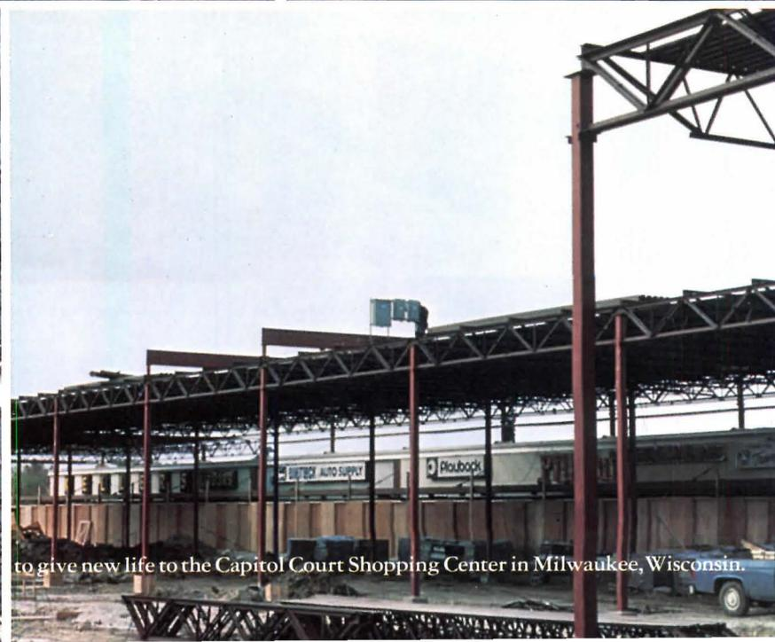
Vulcraft joists and special 116' joist girders were fabricated to give new life to the Capitol Court Shopping Center in Milwaukee, Wisconsin.
