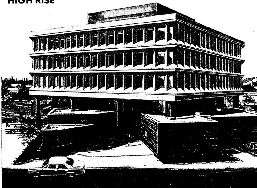
**1** The permanence and appearance of pre-cast concrete at one-eighth the weight. Window wall unit was glazed and insulated in the factory offering substantial cost savings at the job site. Insulation was installed within the panel without any loss of floor space. Architect: Simpson, Usher, Jones, Inc., Anchorage, Alaska. Manufacturer: Olympian Stone, Redmond, Washington.
