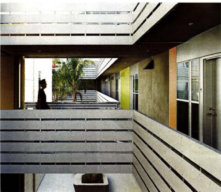
MATERIAL MATTERS Fiber-cement siding, perforated aluminum-zinc coated sheet-steel panels, and integral-pigment stucco are durable and easy to maintain, suiting the complex's modest operating budget.
