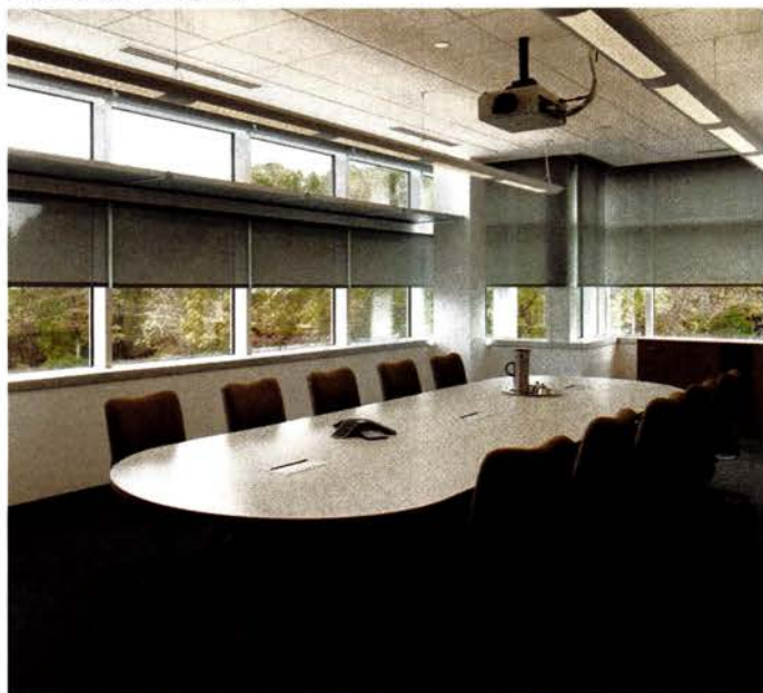
Left: Solar screen fabric helps to prevent glare and preserve views to the outdoors, while the automated shading system controls the position of the fabric on the window. Right: Siting and façade orientation each play a large role in determining what type of daylight is available at a window.
