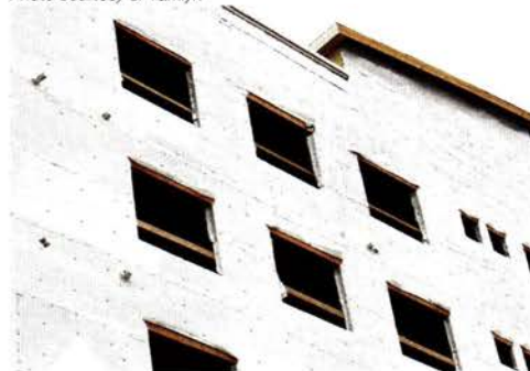
Continuous water-resistive barriers (WRBs) are required by code and provide improved construction performance.
