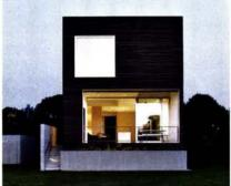
The dark exterior of the 2,200-square-foot house is clad in custom-milled slats of cypress. Each 11/2"by-3" slat has been charred, brushed, and oiled (far left). The east facade serves as the entry and faces the pool and separate garage (top, left). An elevated deck for outdoor dining is tucked below the main bedroom and includes an open-air skylight (left). Large cutouts in the ceiling flood the ground-floor public space with natural light as it overlooks Quonochontaug Pond
