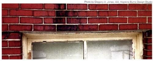
Lack of flashing and weeps has allowed water to collect on the top of the lintel, causing rust. Rust jacking has lifted the masonry above by approximately 3/8 inch, and deflected the lintel downward in the center where there is nothing to resist the rust's expansive forces.
