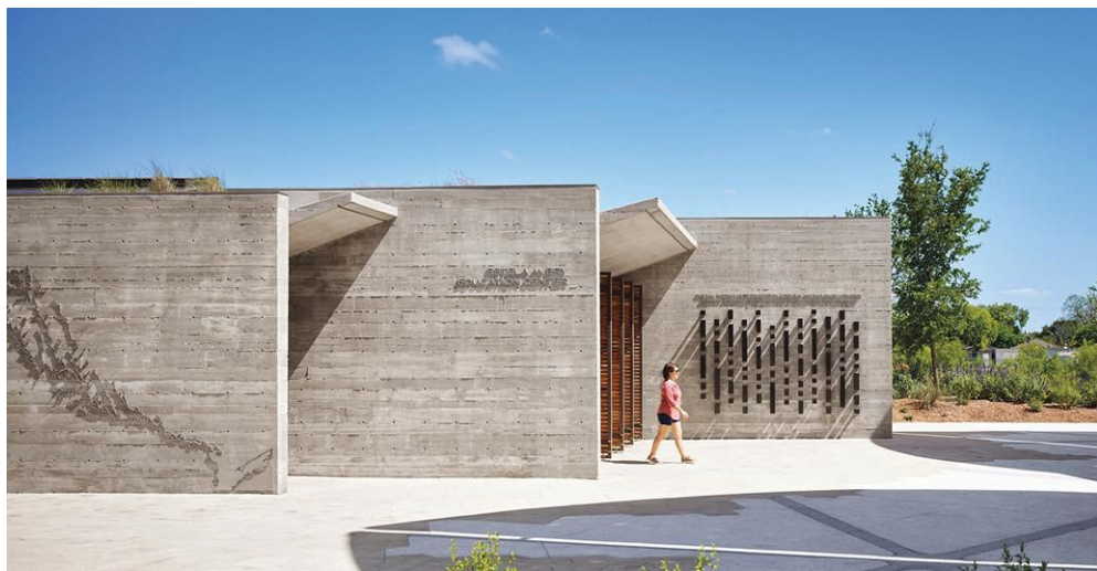
Twenty-two separate concrete "petals," pairs of which are joined by pins at the top, form the main pavilion of Confluence Park (top). Sliding wood-slat doors open one side of the classroom to the outdoors (above).
