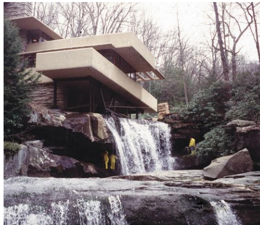
Silman completed the renovations of Frank Lloyd Wright's Fallingwater (1937) in Bear Run, PA, in 2002. The process required the firm to shore up the main-floor cantilever as well as the waterfall's rocky ledge.
