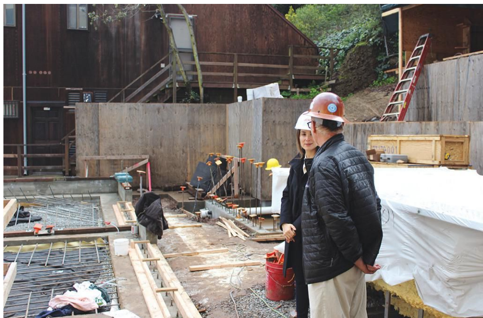
Jensen Architects on-site in San Francisco
