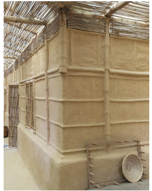
The main factory buildings surround a protected courtyard and are nestled into a remote, hilly region (left). Walls are made of brick and covered in lime (above). Hand-laid stone pathways provide circulation through the stepped site (bottom, left).
