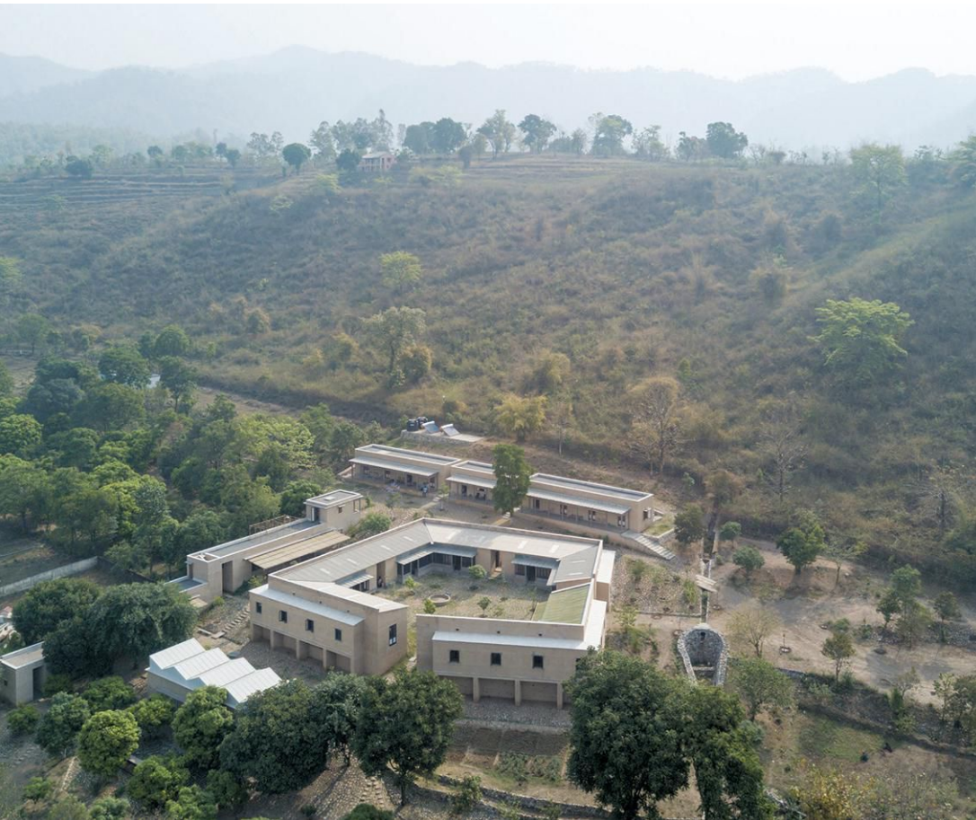
The main factory buildings surround a protected courtyard and are nestled into a remote, hilly region (left). Walls are made of brick and covered in lime (above). Hand-laid stone pathways provide circulation through the stepped site (bottom, left).
