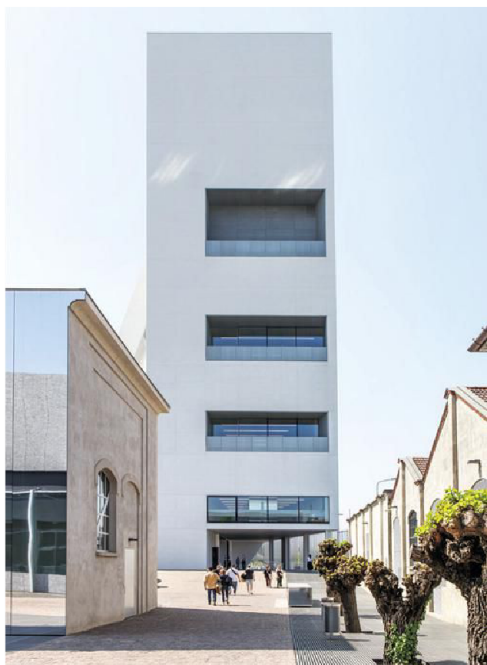
As visitors walk toward the northwest corner of the Prada Foundation complex, they encounter the east facade of the Tower (above). Also visible is the "tube," the structural element on the south side, which encloses cables that help anchor the cantilevers on the north facade (image, below).
