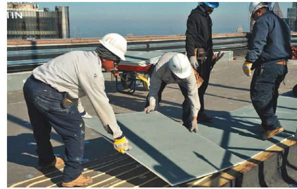
Glass mat gypsum cover boards are composed of a fiberglass mat with a gypsum core, combining the benefits of gypsum products with rigid, water-resistant fiberglass.
