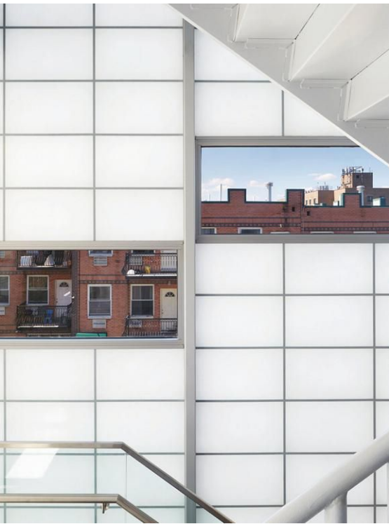
New York Psychotherapy and Counseling Center (NYPCC) Brooklyn, NY | Bromley Caldari Architects PC
