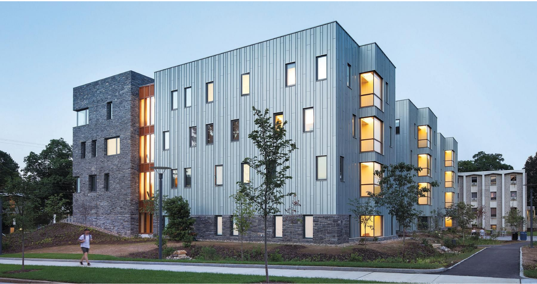
STONE FACED From the main campus road, the residence hall formally expresses itself as part of the Dickinson campus with its limestone cladding (top). Mahogany cladding visually links the two facades; a high-performance landscape wraps around the building's perimeter (above).
