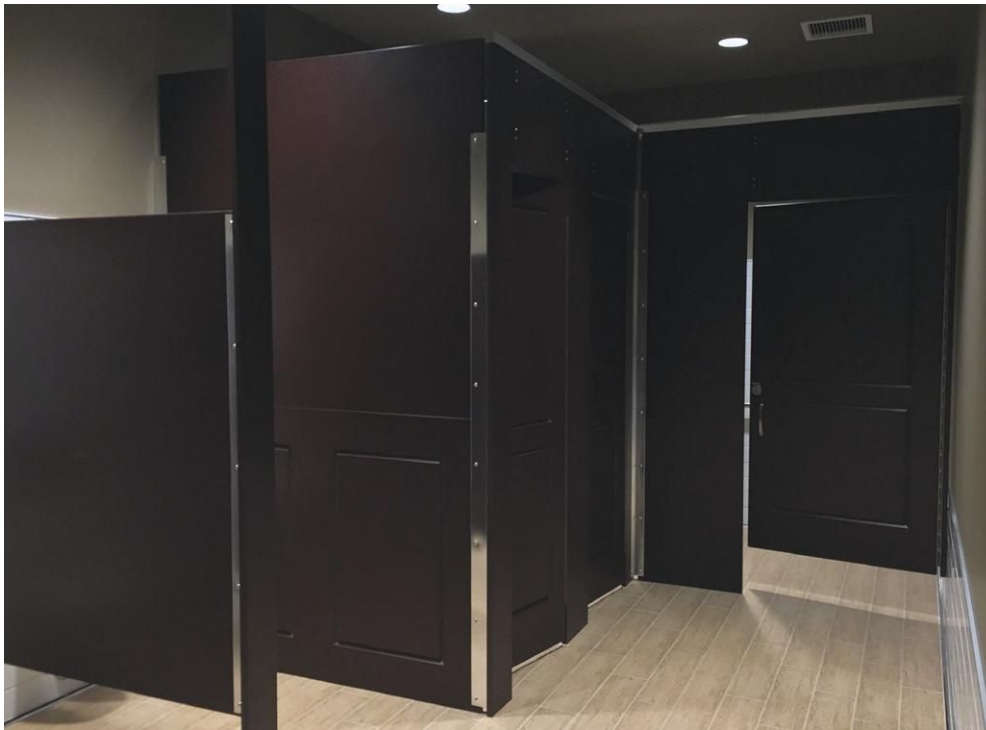
In the headquarters of the Sacramento Regional Builders' Exchange (SRBX), the restroom partitions are made from solid HDPE and feature shoeless pilasters, which deliver a cleaner aesthetic that is also easier to clean.
