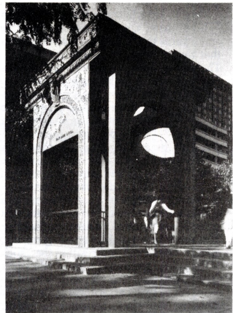
Orbanco Building Gazebo, Portland. SOM, Architects.
