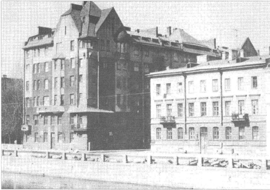
Apartment House, No. 159 Fontanka Quay
