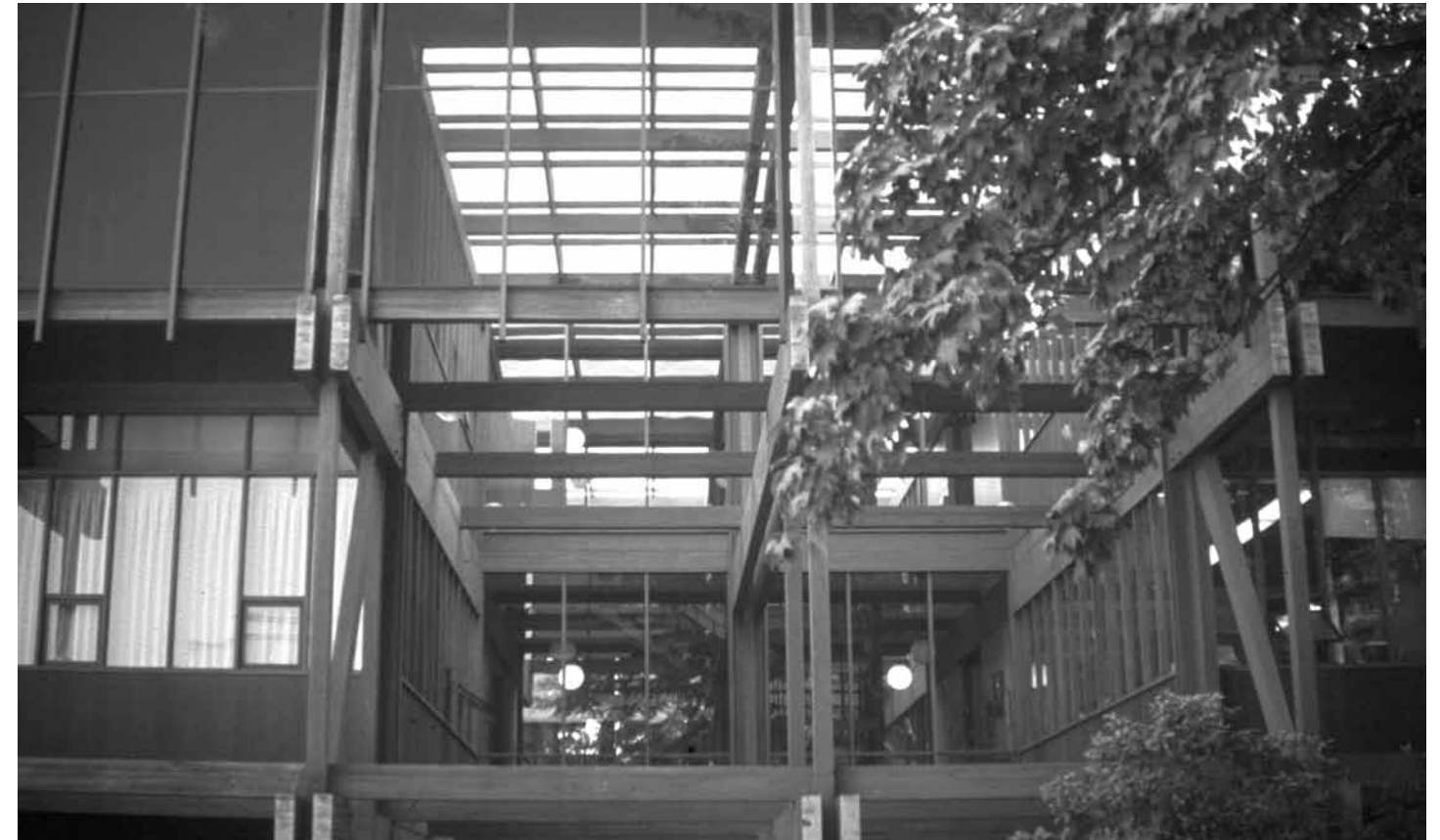
The skylit, light-filled atrium occupies two bays and provides for primary vertical circulation by means of the stairs partly visible through the glazing. Image from the Visual Resources Collection, College of Built Environments, University of Washington.
