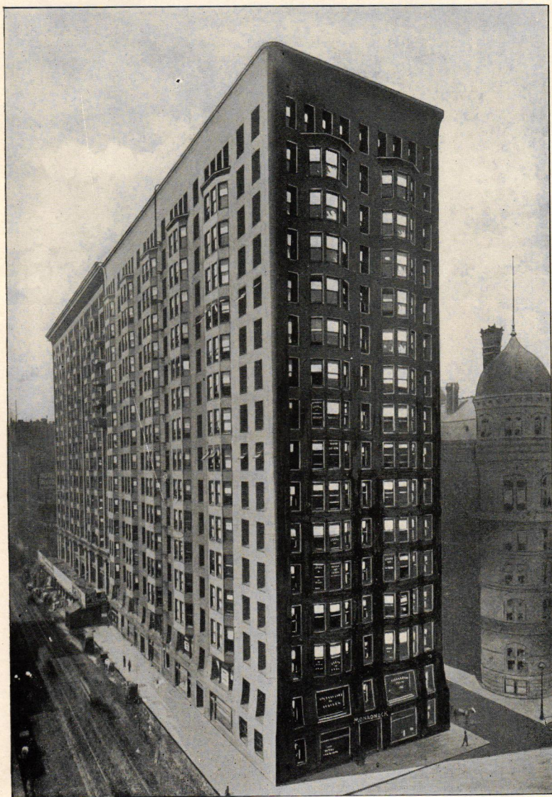
THE MONADNOCK BUILDING, CHICAGO.
