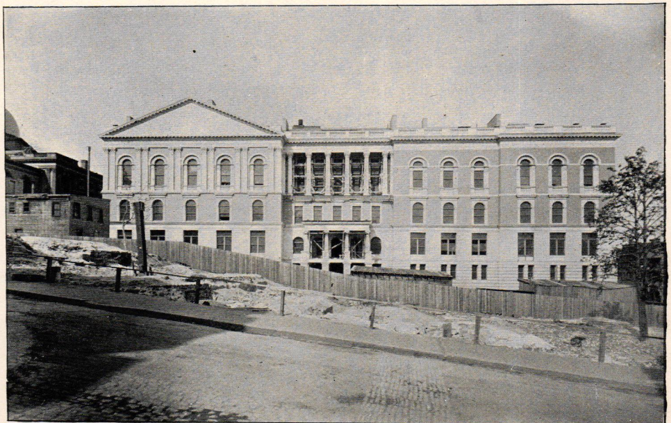
EASTERN FAÇADE OF ADDITION TO MASSACHUSETTS STATE HOUSE.
