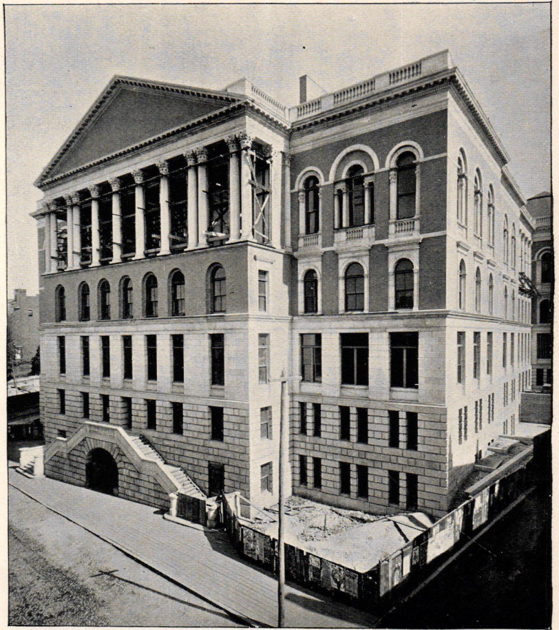
NORTHERN FAÇADE OF ADDITION TO MASSACHUSETTS STATE HOUSE.
