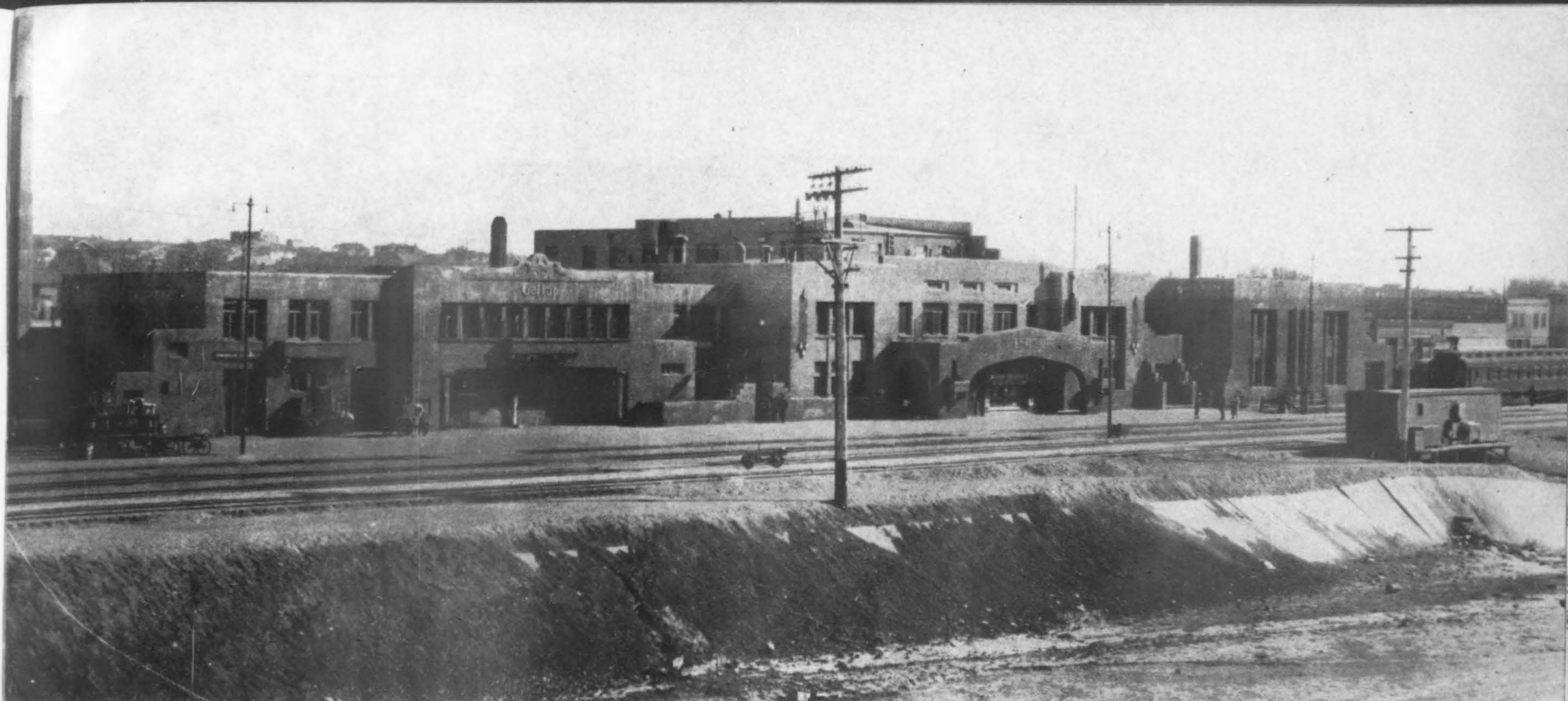
The El Navajo Hotel at Gallup entails the most vigorous modern statement. In the building one discovers horizontal and vertical grouping of windows, "cubistic" handling of walls and projecting balconies, and three tasseled pair of lights attached to the main block of the building, all of which were design motifs which had become the vocabulary of the early modern movements in European and American architecture.
