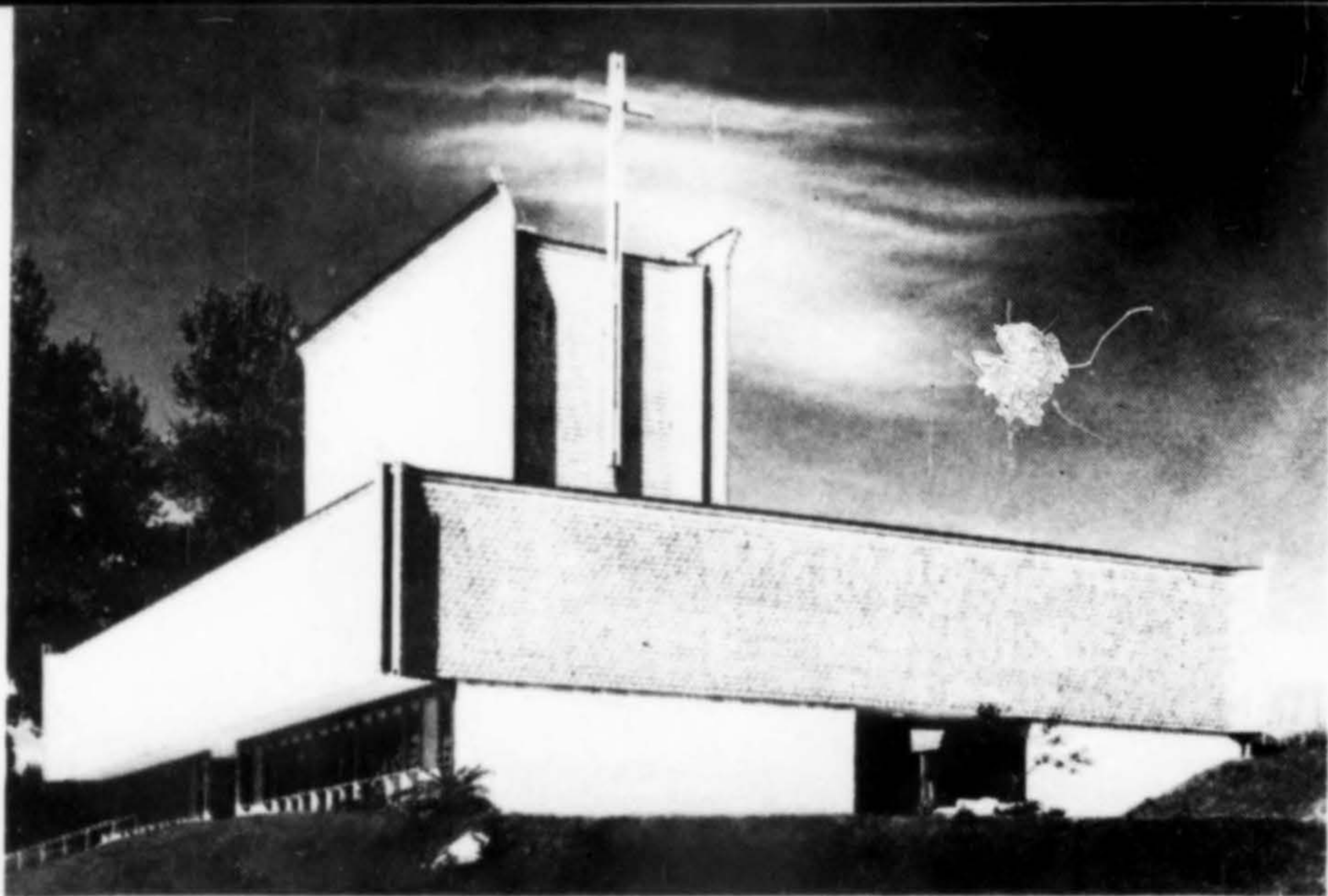
JAPANESE PRESBYTERIAN CHURCH , Seattle. Architects: Kirk, Wallace, McKinley, AIA, & Associates. "Their solution is deceiving in its simplicity, born of a highly creative imagination which saw very clearly the problems and levels of design consideration involved. The design expresses in its materials the context of region, neighborhood, and site, while reflecting in form the ethnic overtones of its occupants, without compromising the solution by direct use of traditional idioms."
