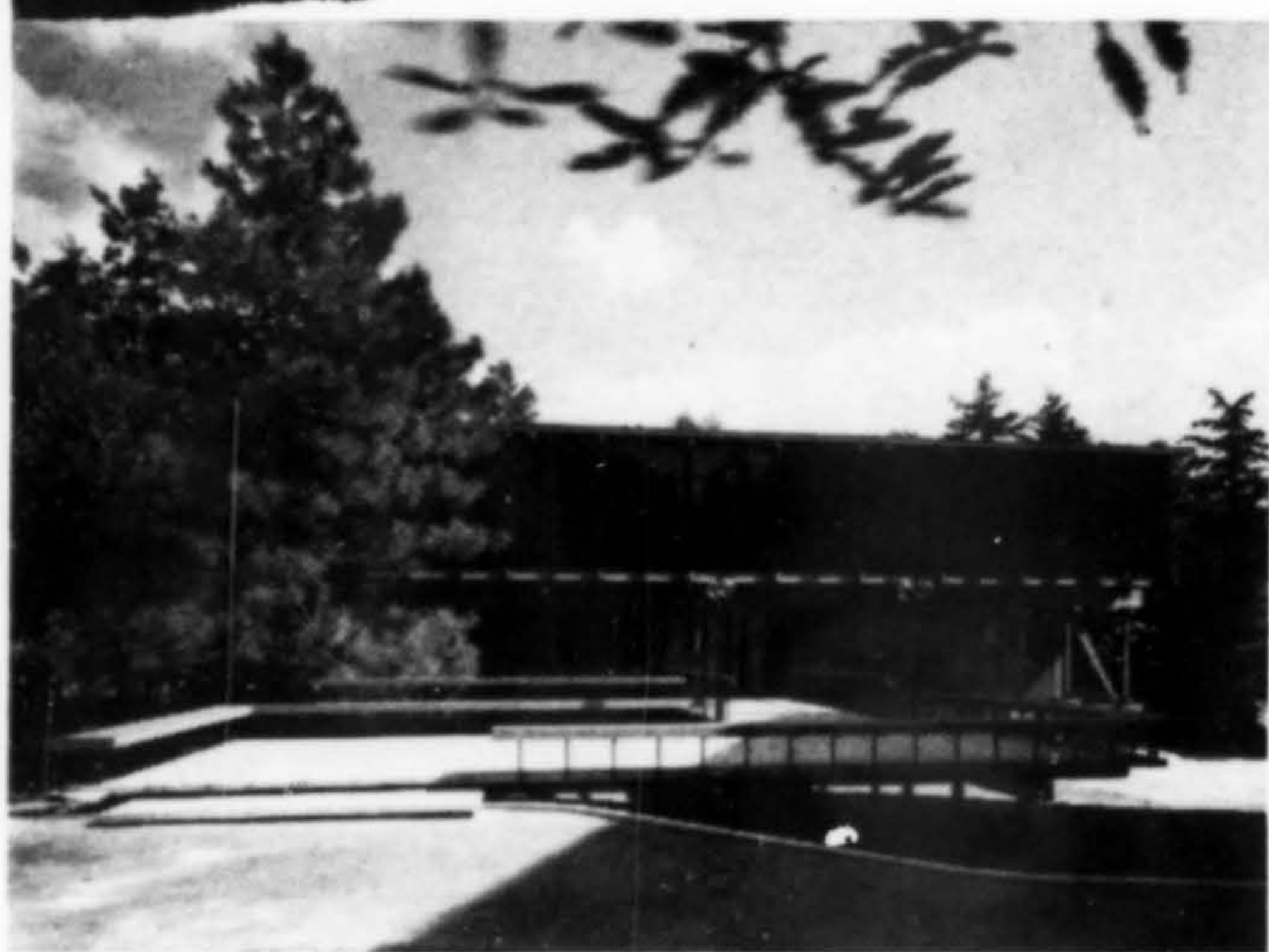
HUGO WINKENWERDER FOREST SCIENCES LABORATORY , University of Washington. Architects: Grant, Copeland and Chervenak and Associates. "It synthesizes these elements of site, materials, and program without compromise; making of these elements one of the most beautiful expressions of the wood style to emerge in recent years. Especially admirable is the way the building is located within its environment. It sits very agreeably with its neighbors of various styles by means of deft handling of existing trees as transitional elements."
