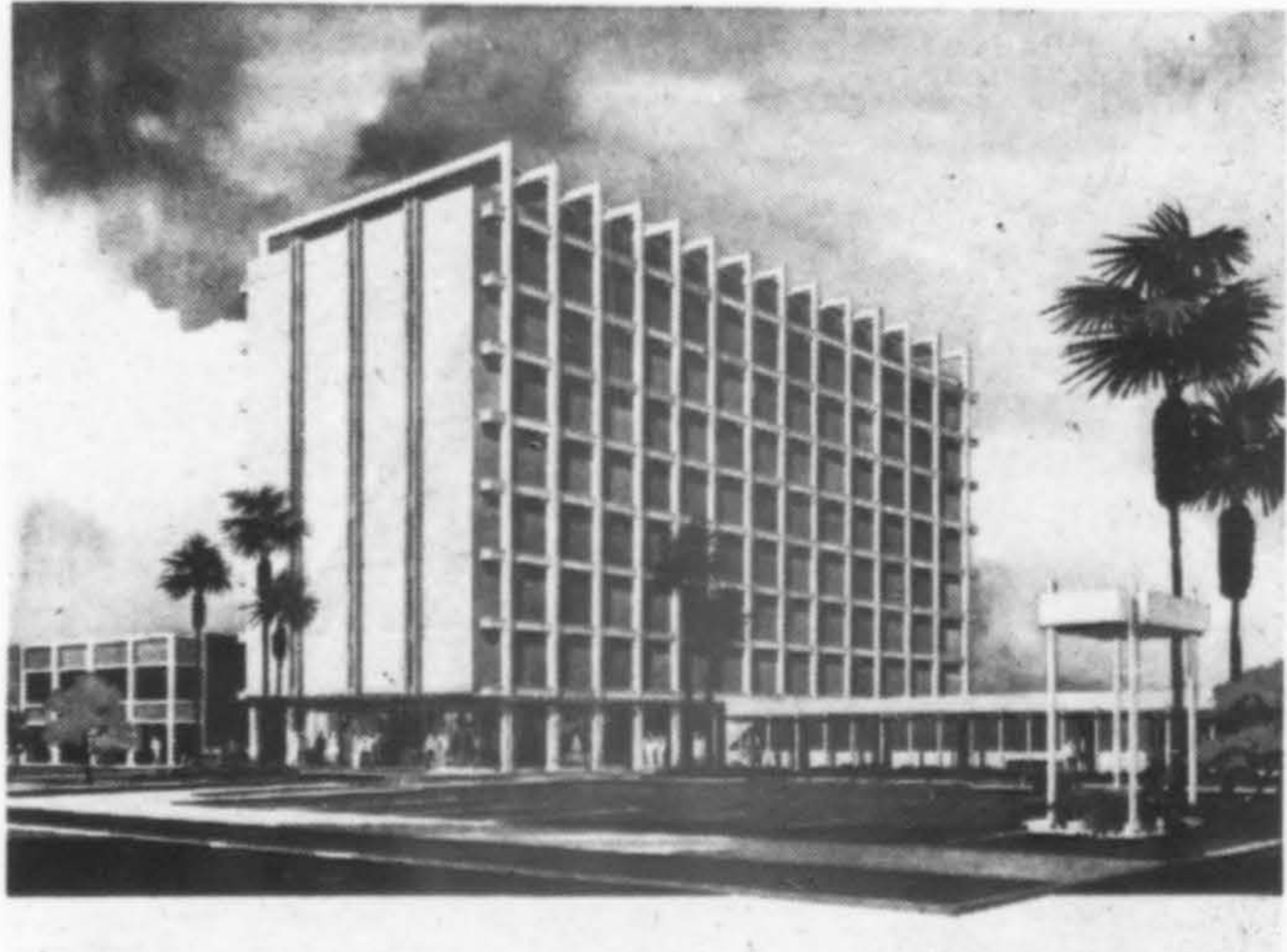
O'MALLEY BUILDING , Phoenix, a $2 million project is scheduled for completion, September 1965. A porcelain enameled steel tube canopy around first floor area gives a horizontal accent and a beginning for the building's base. Building frame is set two and one-half feet in front of exterior walls, providing protection for exterior walls from sun. East and west walls are predominantly void of glass, are textured with exposed, colored concrete. All glass will be solar bronze. Entrance doors are nine foot high, hand carved wood. Landscaped plaza surrounds building. Architects: Weaver and Drover, Phoenix; Walter Riley, structural engineer.
