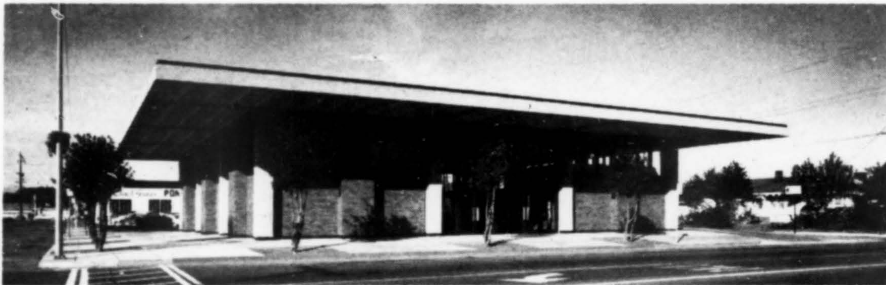
NATIONAL BANK OF WASHINGTON , Auburn branch. Architects: Liddle & Jones. Honor Award. "A handsome building, handled in a skillful manner . . . imparts a sense of dignity and purpose. It sets a high standard for the requirements of the urban design of the commercial neighborhood where it is found."
