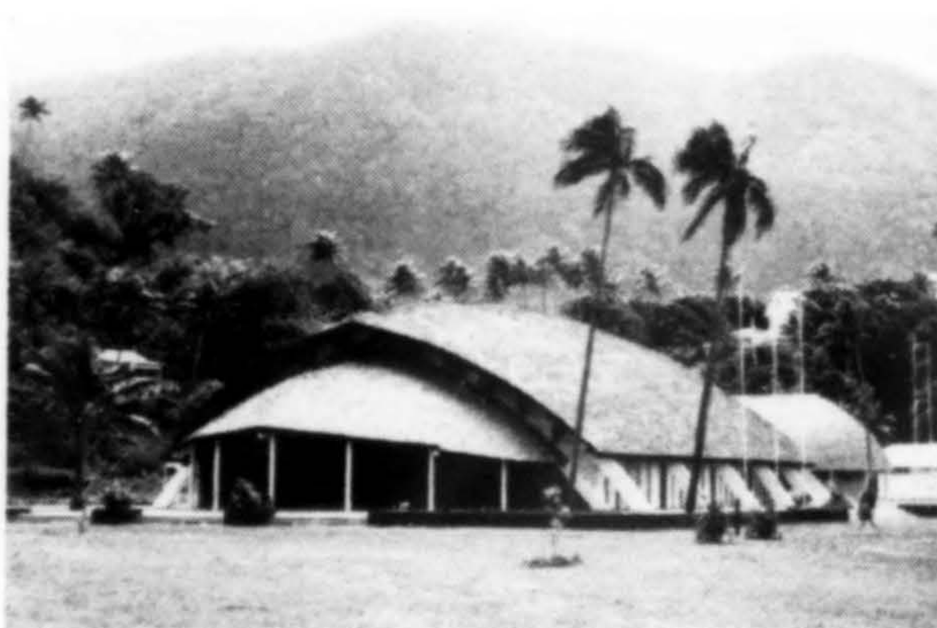
CIVIC AUDITORIUM , American Samoa. Architects: Wimberley, Whisenand, Allison & Tong. Captures the essence of the traditional "fale" or longhouse of Samoa.
