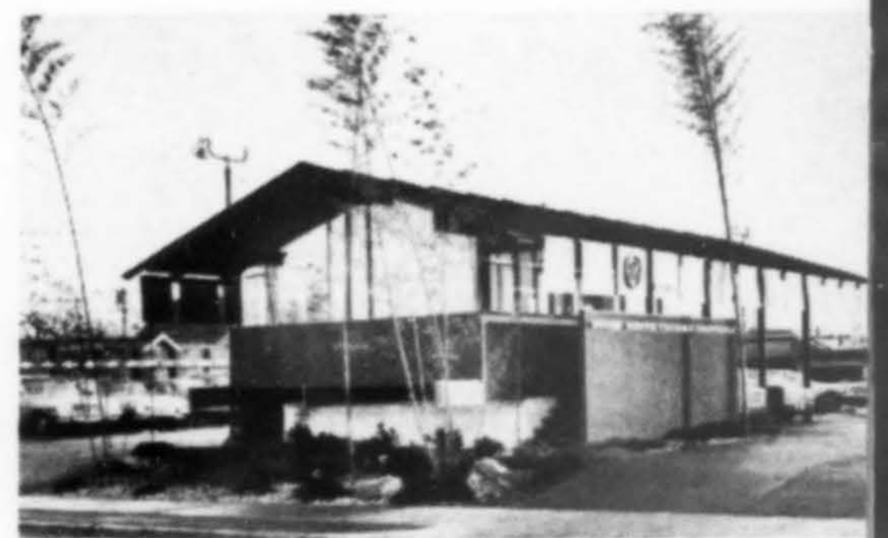
SOUTH TACOMA CHEVROLET MOTOR MALL . Architect: William Hocking. Award of Merit. "The handling of the needs of a used car emporium, here for the first time, may provide an example that may alleviate the ugly problems of our arterial automobile row areas. The architects and the clients are to be commended for a thoughtful and successful solution to a problem."
