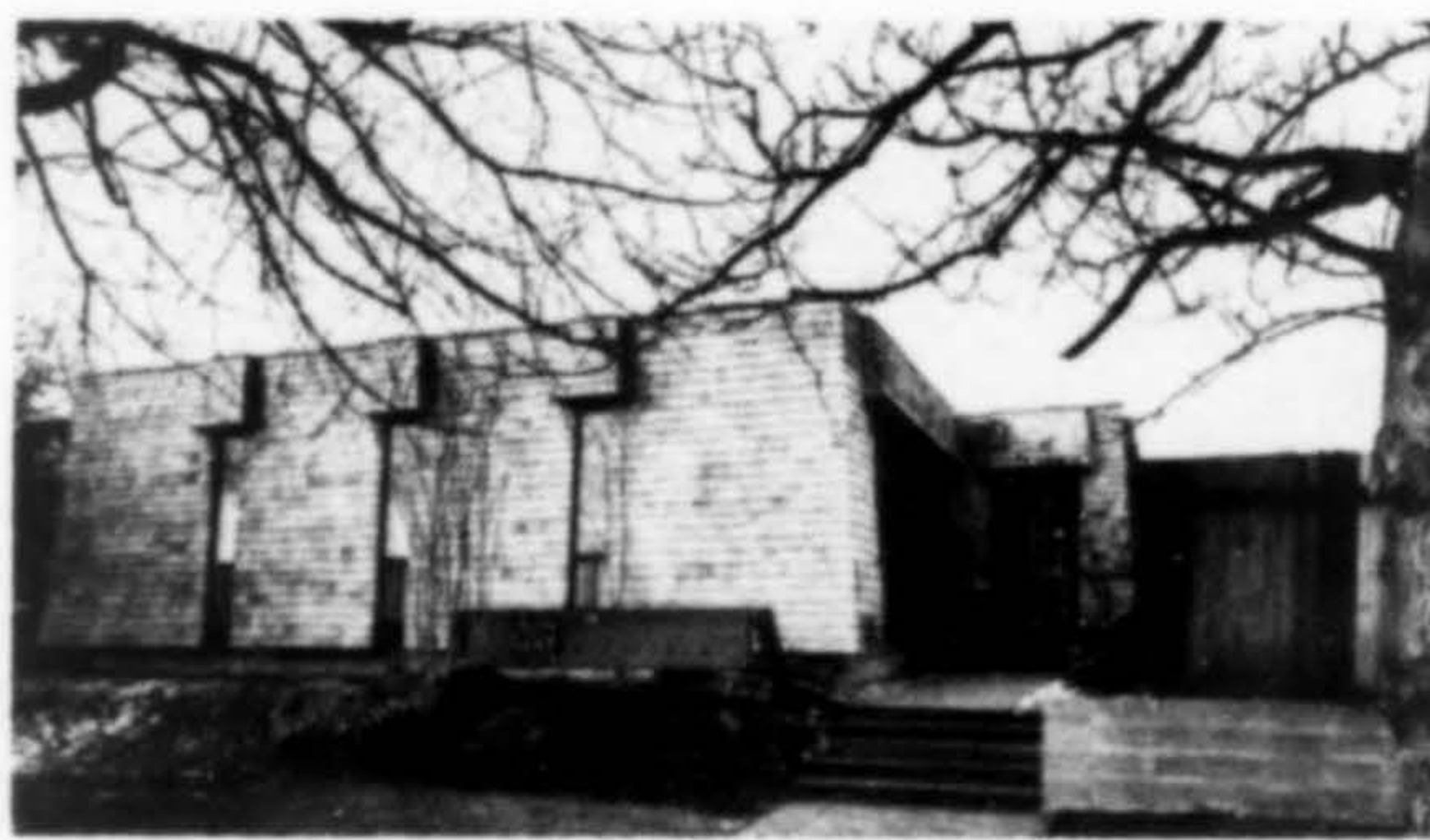
CECCANTI'S RESTAURANT . Architect: William Hocking. Award of Merit. "A fine solution for perceptive clients who have made a contribution to the growing needs of Tacoma for a fine set of places in which to dine. The bar seems especially successful and is an appropriate and skillfully designed room . . . commends particularly the excellent graphics of the sign at the entrance to the site. The exterior character of the building and the interior design add up to an architectural success."
