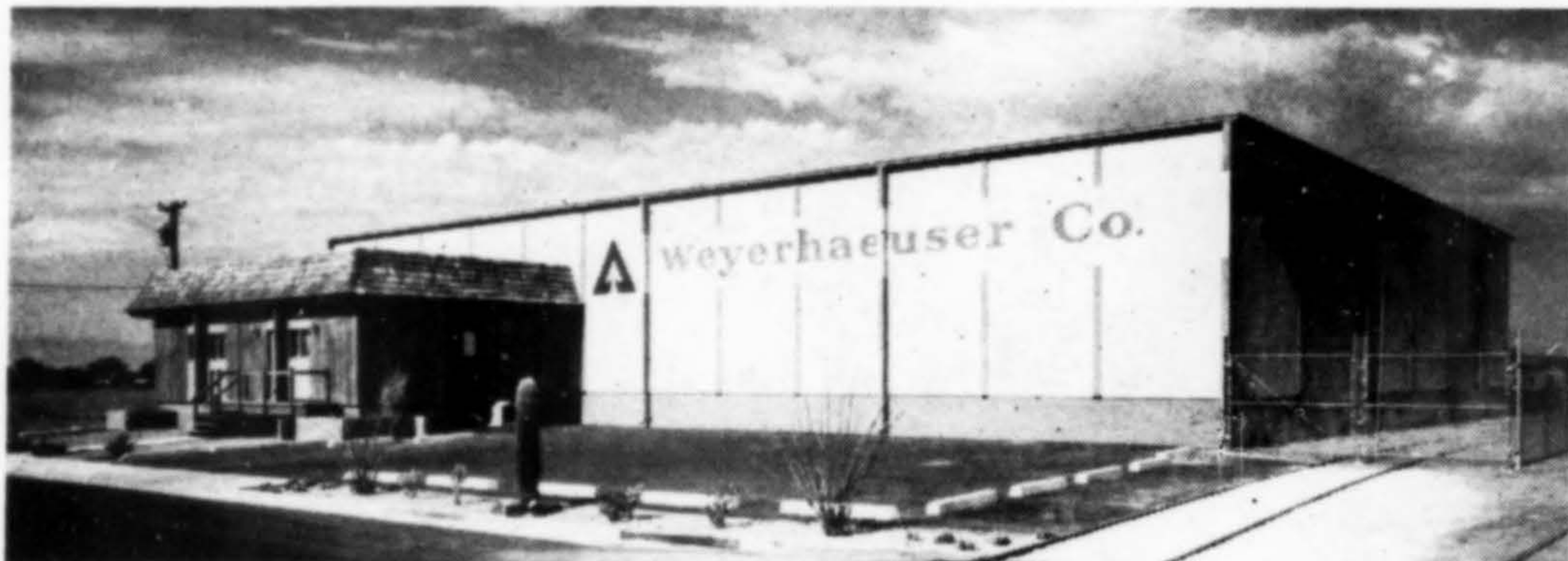
WEYERHAEUSER'S new facility in Phoenix, Arizona, predominately incorporates the firm's own building products: wall panels built on the floor and tilted into place, similar to tilt-up concrete work. Laminated wood beams supported by laminated wood columns formed outside members of the adjoining panels. Lateral loads are resisted by plywood roof, a non-functional expression which has become something of a Weyerhaeuser trademark. Harry Youngkin was architect.
