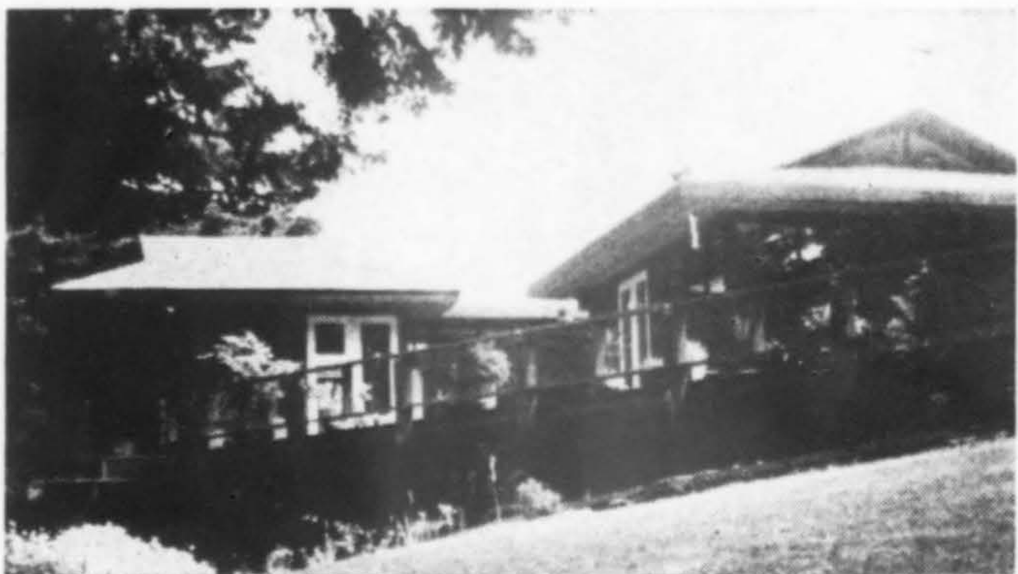
RESIDENCE of DR. and MRS. E. BURNS LEE , Arcata, California. Architect: William M. Van Fleet. "A good definition of plan use. Good use is made of the site and garage. This house represents an achievement of character at a reasonable cost."
