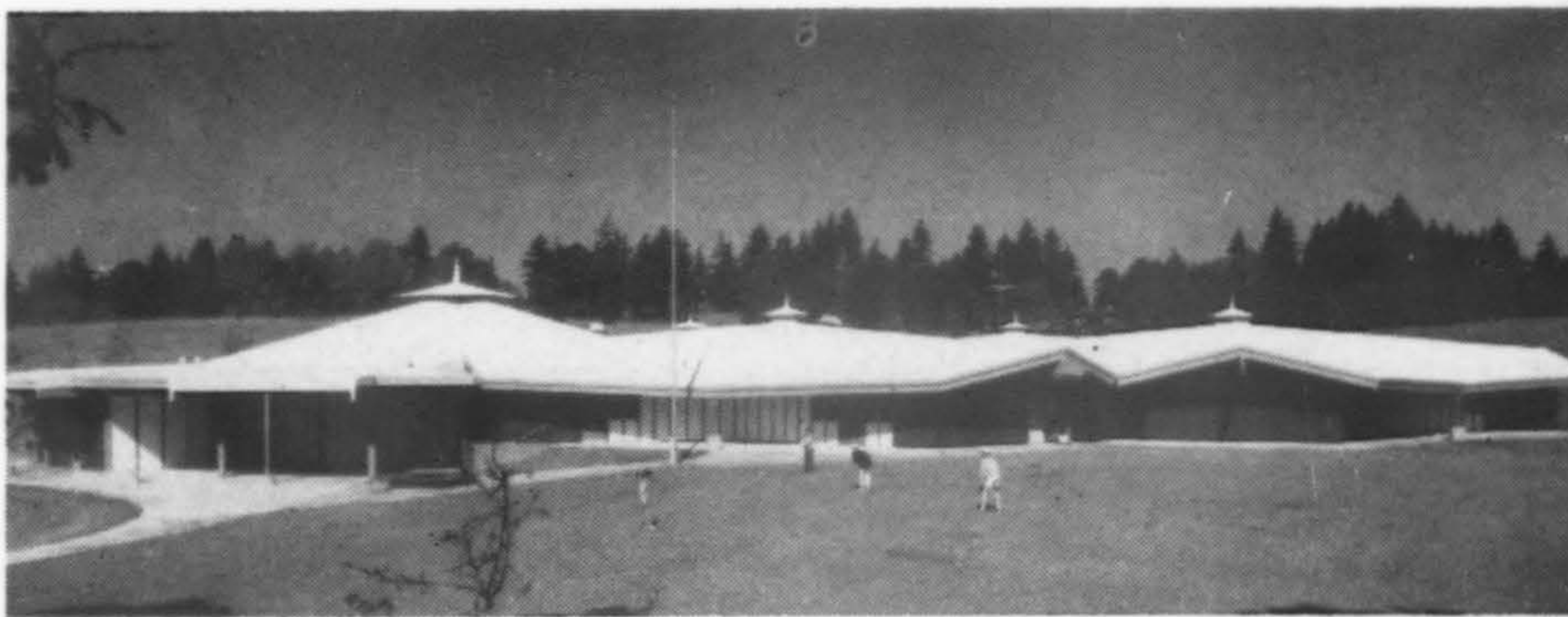
CREST DRIVE ELEMENTARY SCHOOL , Eugene, Oregon, received an Award of Merit in the American Association of School Administrators exhibit at Atlantic City in February. Architects: Stearns, Mention and Morris, Eugene.
