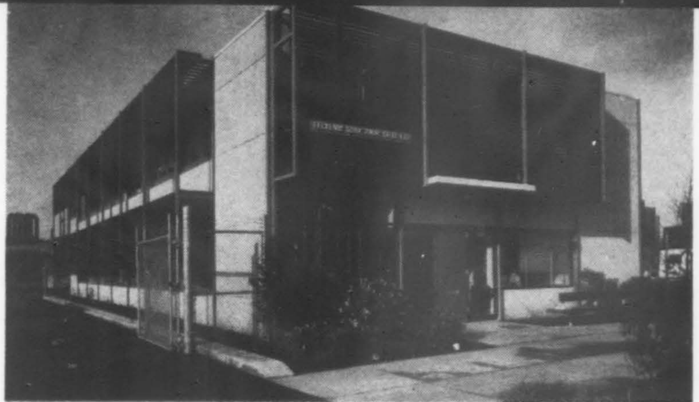
LECKENBY STRUCTURAL STEEL COMPANY opened new offices at 2745 - 11th Avenue S.W. on Seattle's Harbor Island earlier this year. Architect: Durham, Anderson & Freed; Herbert U. Taylor Co., general contractor.
