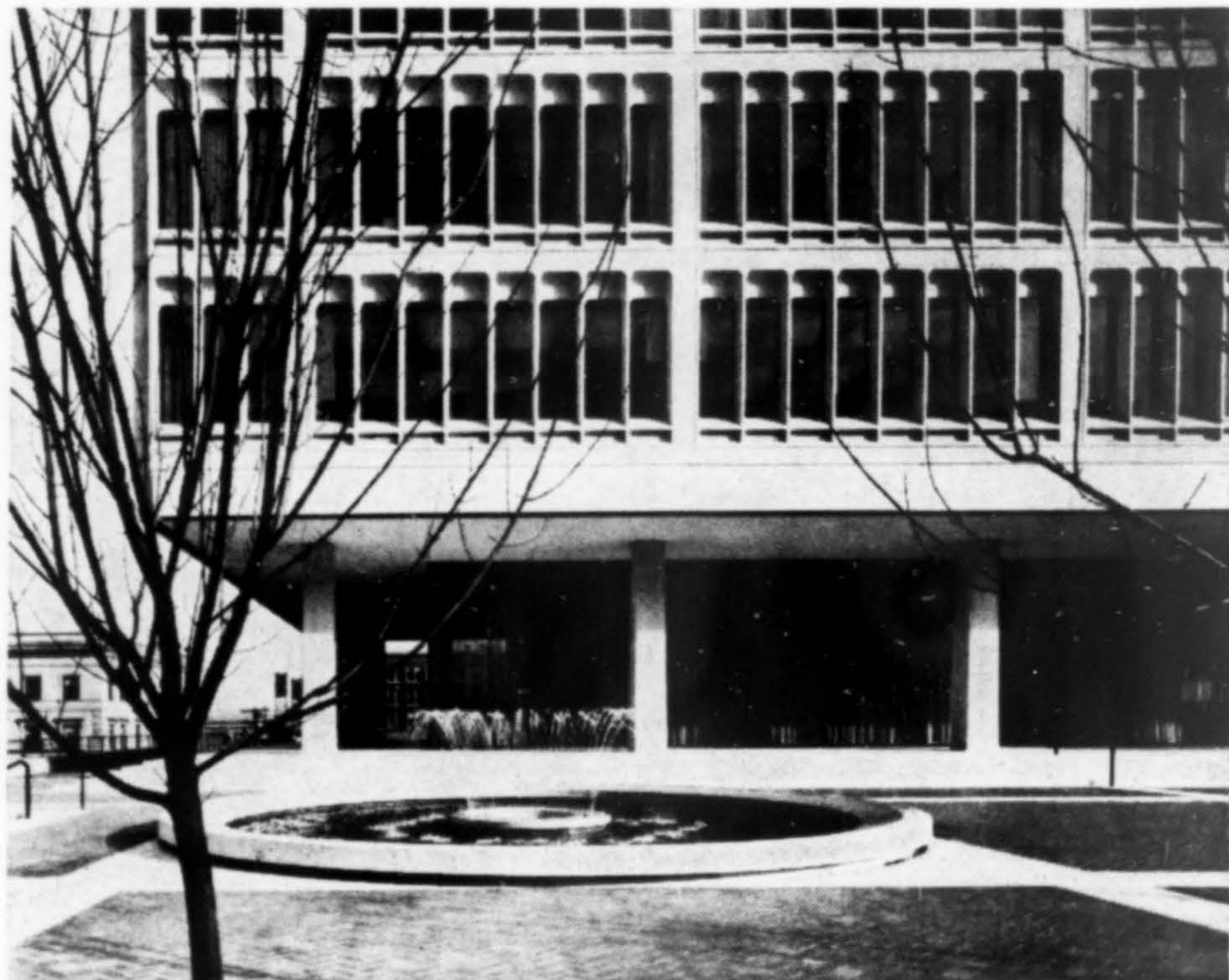
EQUITABLE SAVINGS & LOAN ASSOCIATION Building. Honor award. Architects: Wolff/Zimmer & Associates in association with Pietro Belluschi, FAIA. "The building comes at a time when faceted gems fronted by plazas have become a national cliché . . . the serious attention to refinement of detail and proportion throughout this building should be instructive to those who might too easily follow . . ."
