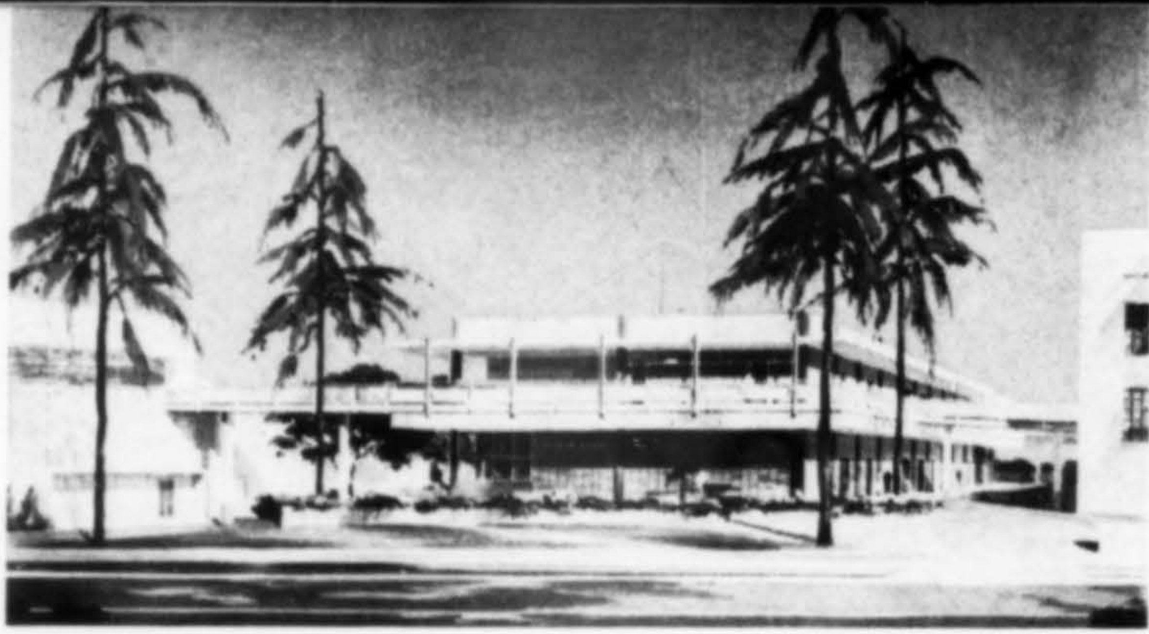
TECHNOLOGY BUILDING at Pasadena City College, Pasadena, is scheduled for completion in August. Building is planned as a modular frame in three rows of columns supporting concrete joists and cantilevered balconies and roof structures. Cost: $900,000. Architects: Allison & Ribble, Los Angeles; Ropp & Ropp, structural engineers.
