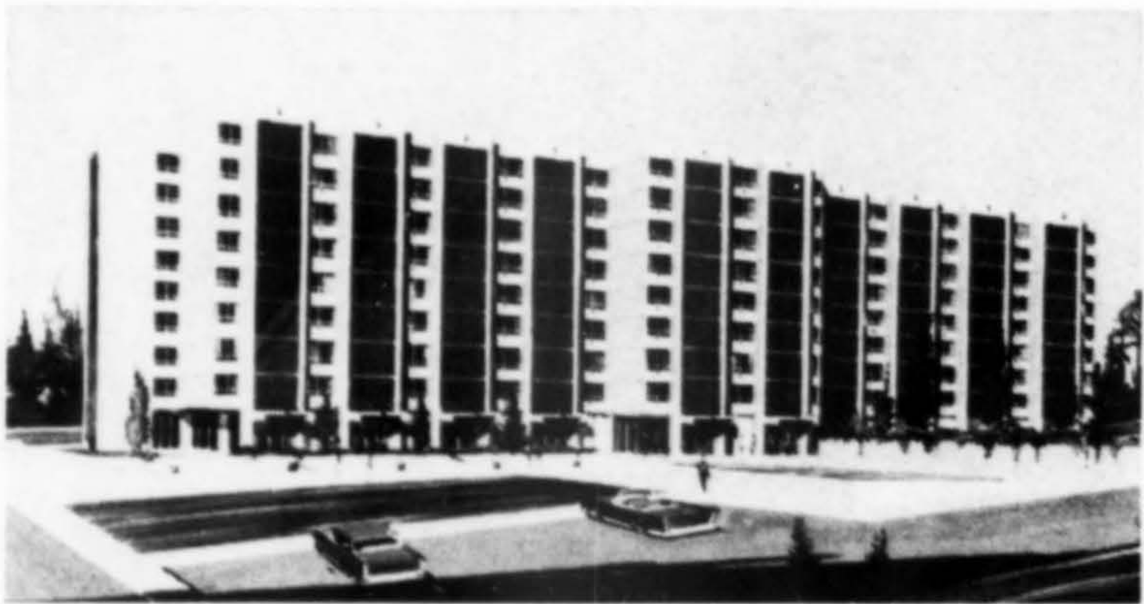
MEN'S HIGH RISE Dormitory, Arizona State College, Flagstaff, will have nine stories. Channel shaped prefabricated concrete column and wall units permit heat piping to be installed as construction progresses. Exterior: exposed aggregate. Cost: $1.6 million. Architects: Guirey, Srnka & Arnold; Foltz, Hamlyn & Adam, structural engineers; Johannessen & Girard, mechanical; Manhattan-Dickmann Construction Co., contractor.
