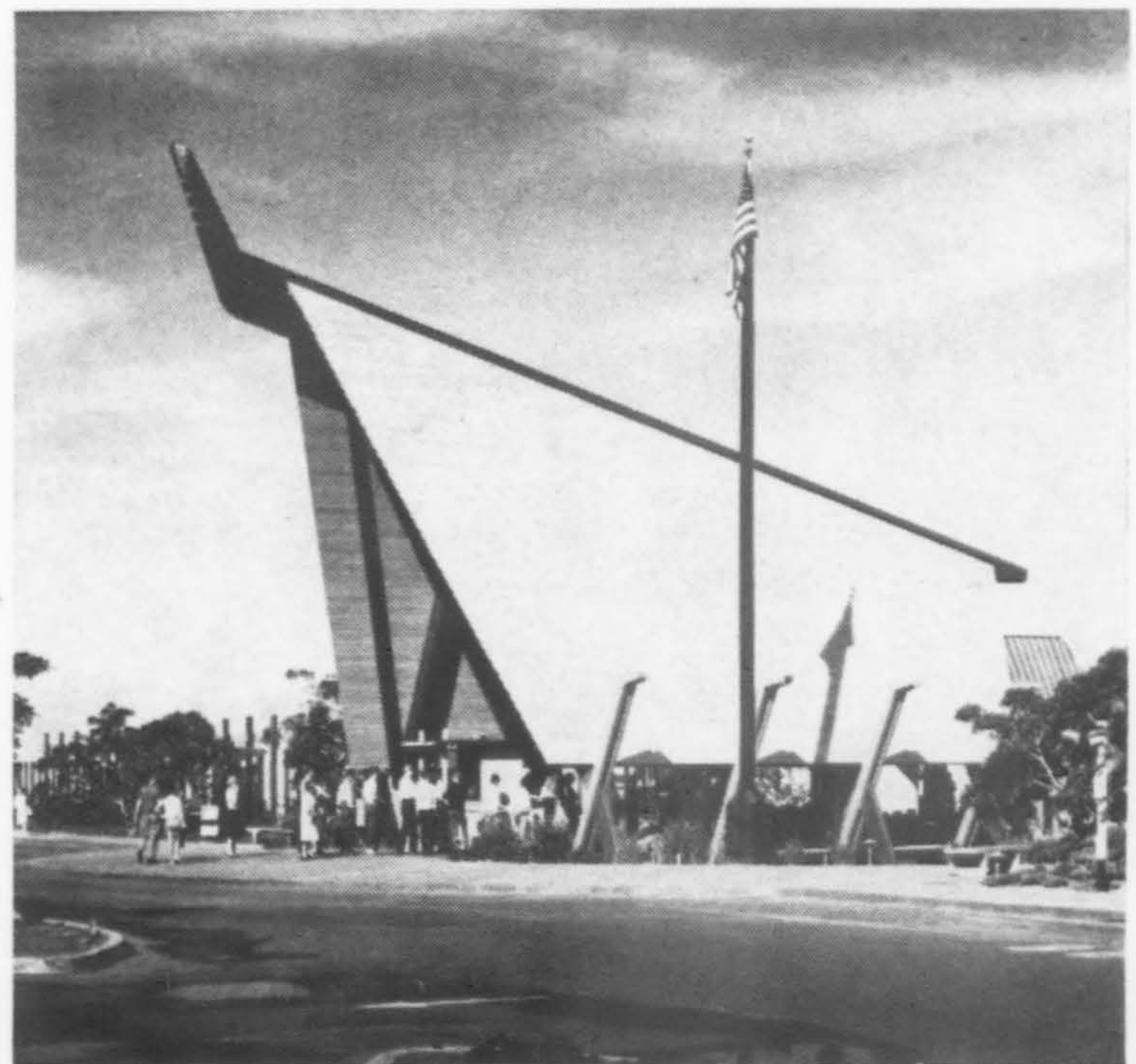
2. ENTRANCE STRUCTURE 50 FT. HIGH PULLS VISITORS.
