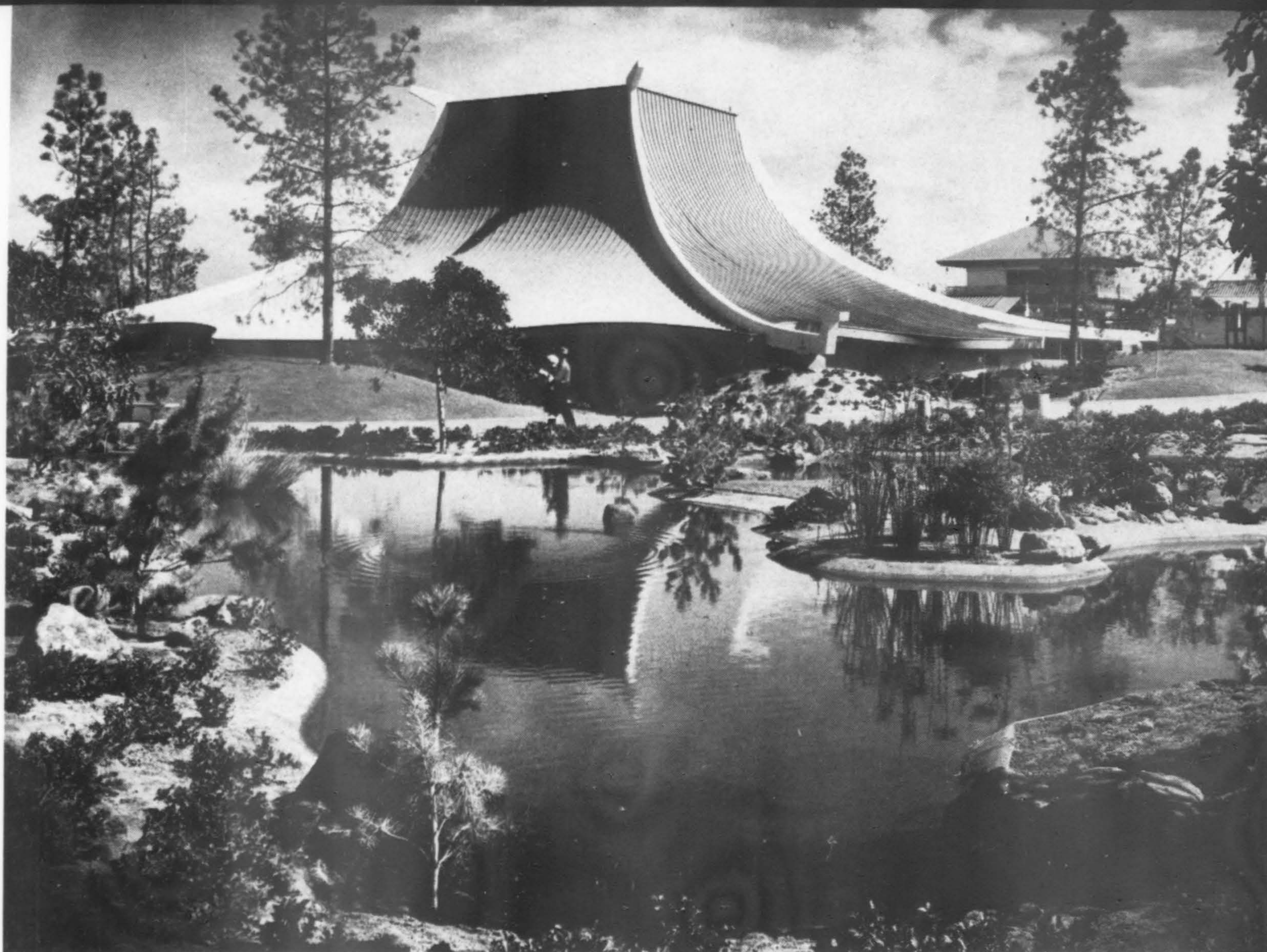
5. UNDERWATER THEATRE ACCOMMODATES 800 PEOPLE WITH NO SPECTATOR MORE THAN 45 FT. FROM A PERFORMANCE. FOUR EXPOSED LAMINATED BEAMS SPRING FROM CONCRETE BUTTRESSES, SUPPORT MECHANICAL EQUIPMENT ABOVE 150,000-GAL. TANK.
