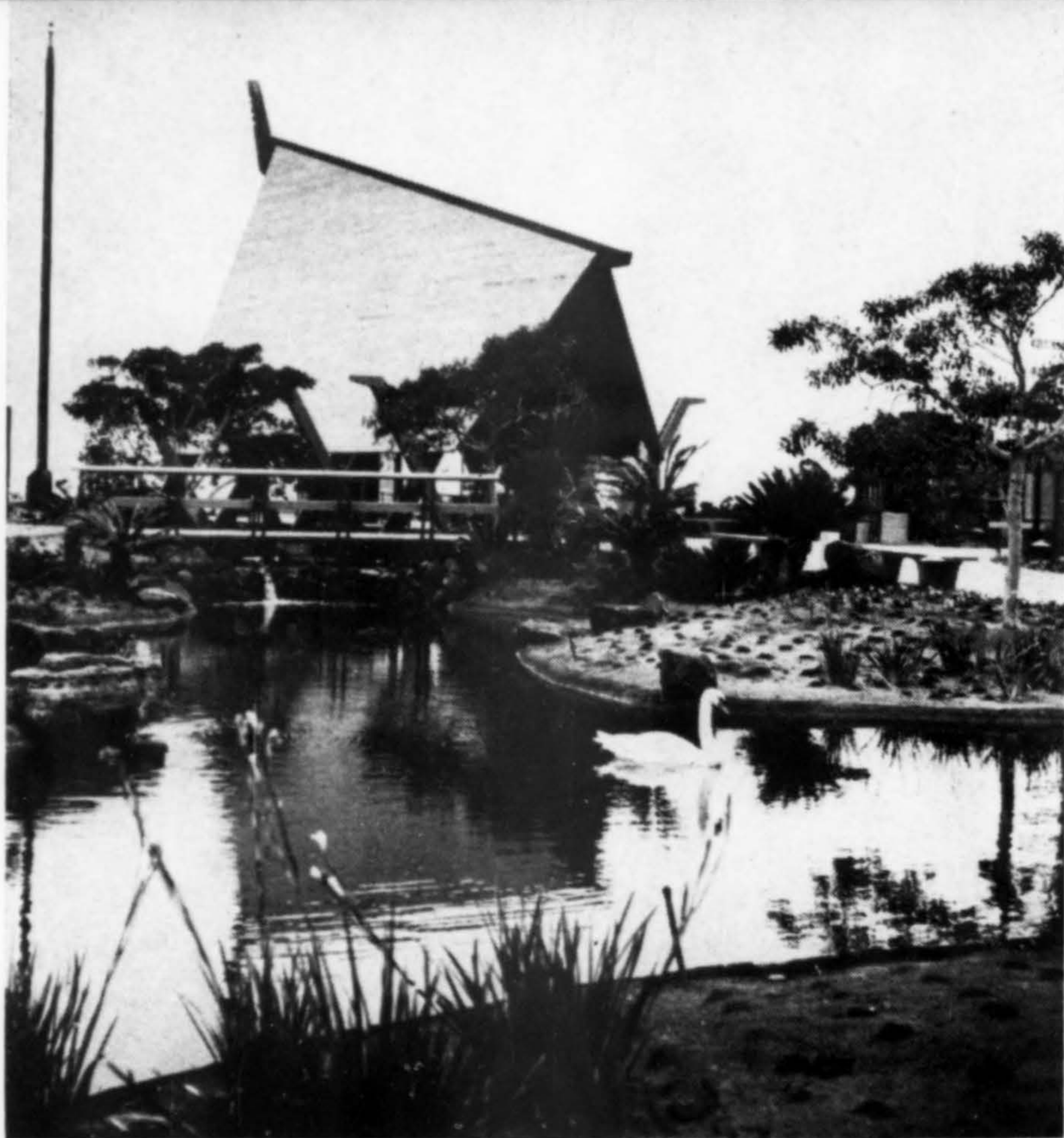
2. CHARM OF LANDSCAPING BEGINS WITH POOLS AT ENTRY STRUCTURE.
