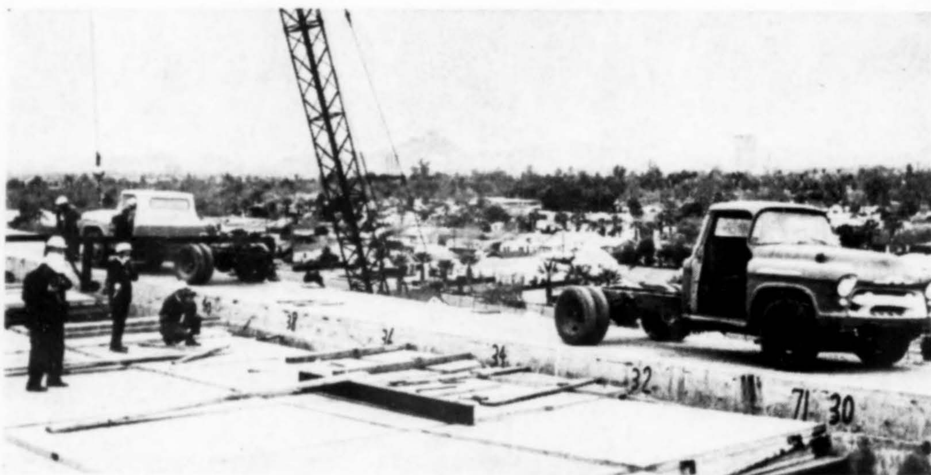
Four trucks atop compression ring carry hydraulic tensioning jacks.
