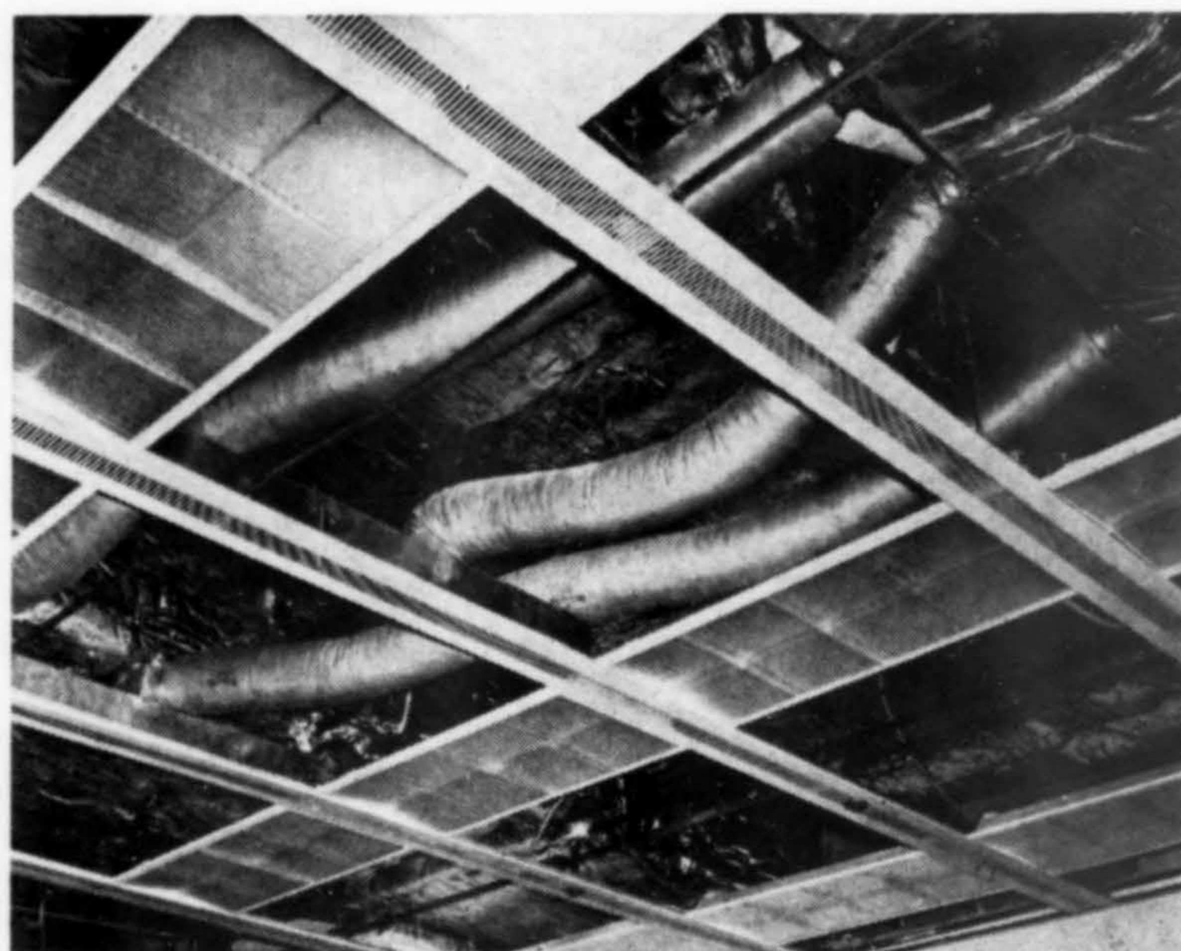
Flexible duct hooks to connections without fittings.
