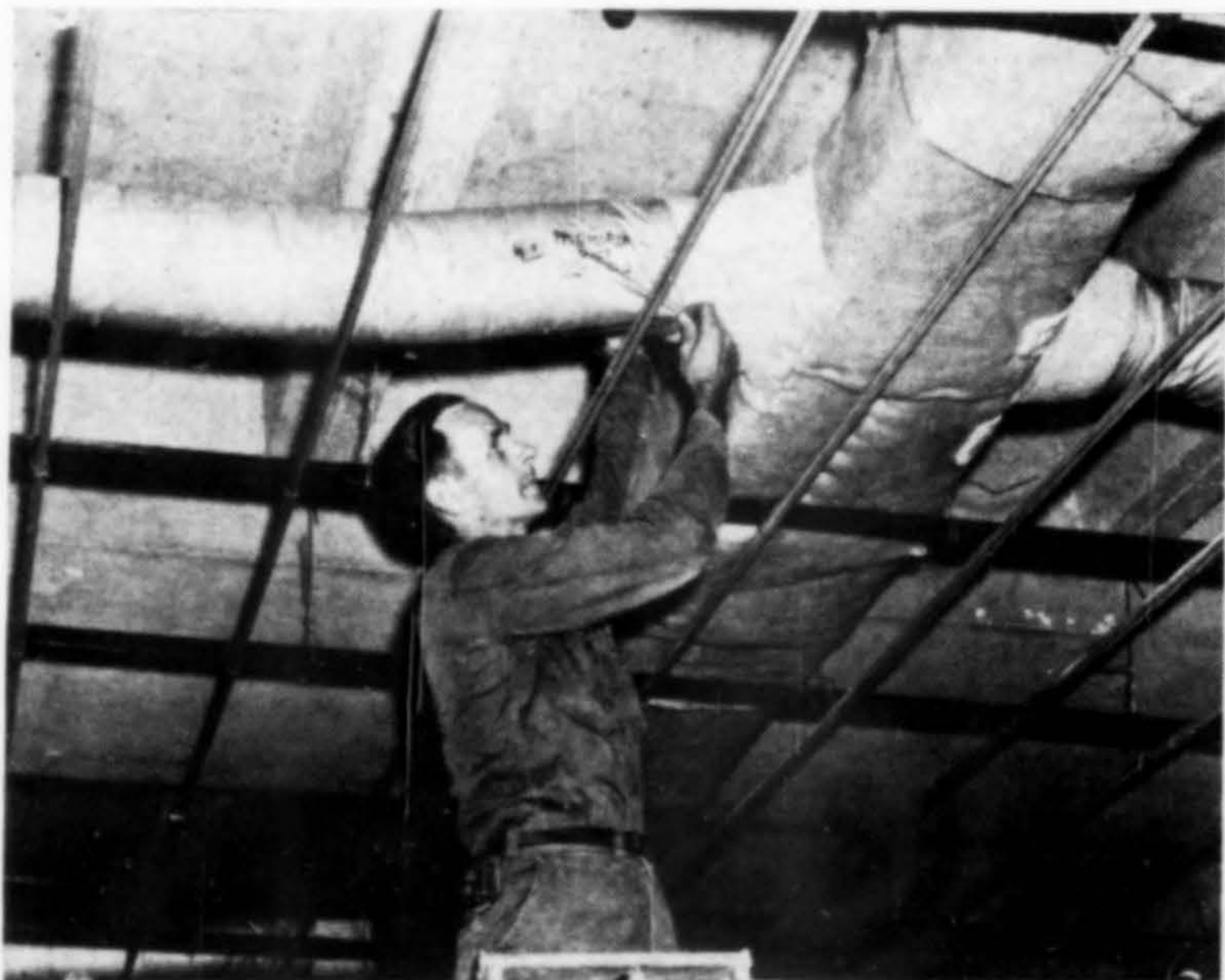
Lightweight duct is cut to fit with knife, taped into place.
