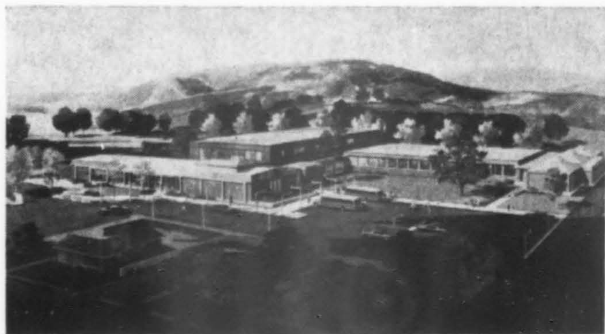
LABORATORIES AND MULTI-PURPOSE ROOM additions, Belt Public School, Belt, Montana. Space will be provided for music department, stage, cafeteria, student commons and related facilities. Fixed science laboratory will be flanked by two lecture rooms. Walls are face brick and exposed concrete frame, laminated wood roof framing. Architects: Hoiland-Zucconi, Great Falls.
