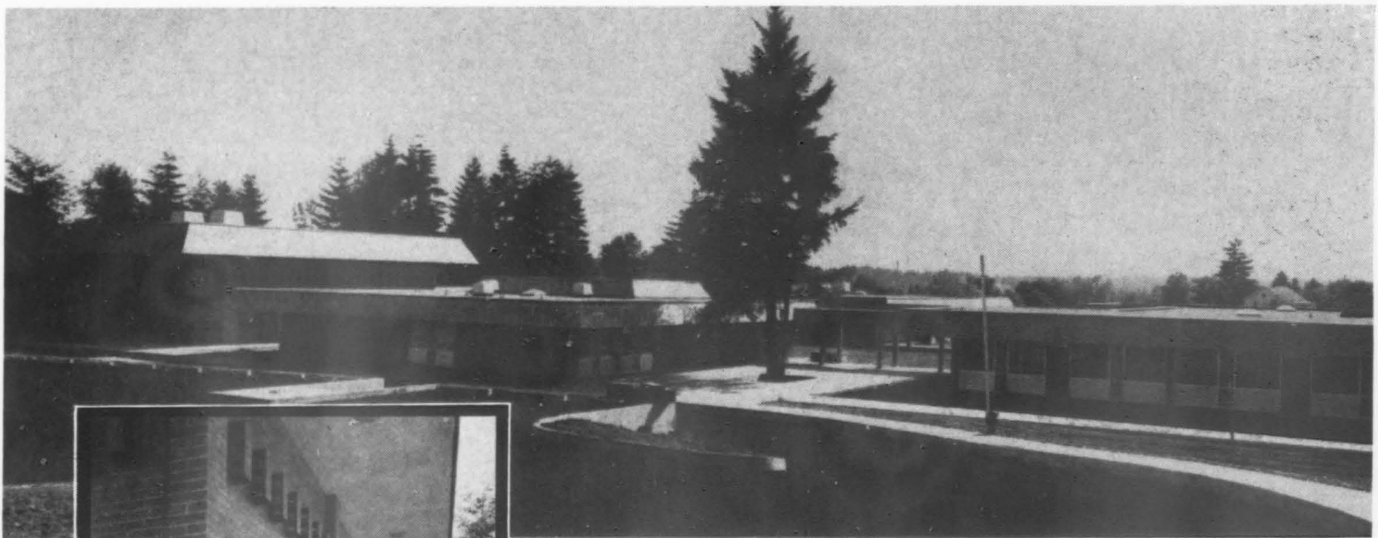
Alderwood Elementary School—Edmonds School Dist. #15
