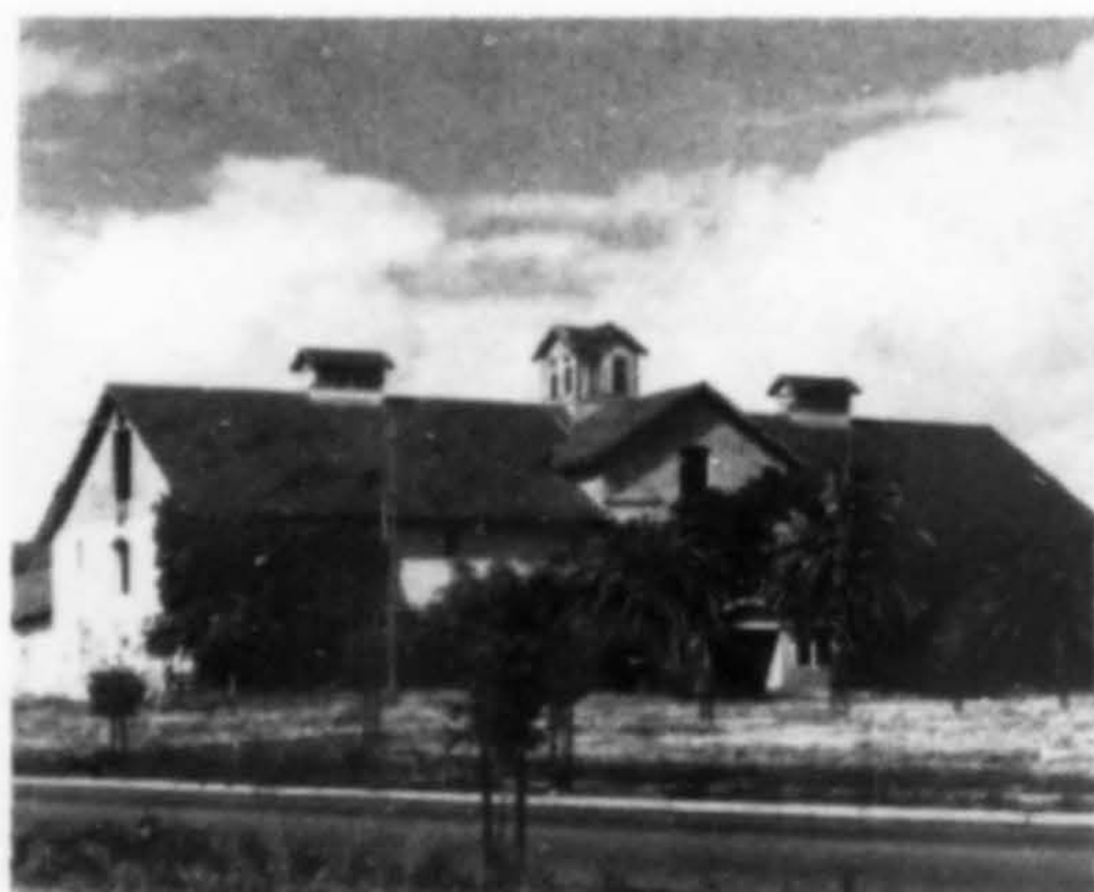
Old parking area before refinishing. Old stucco covers brick walls.
