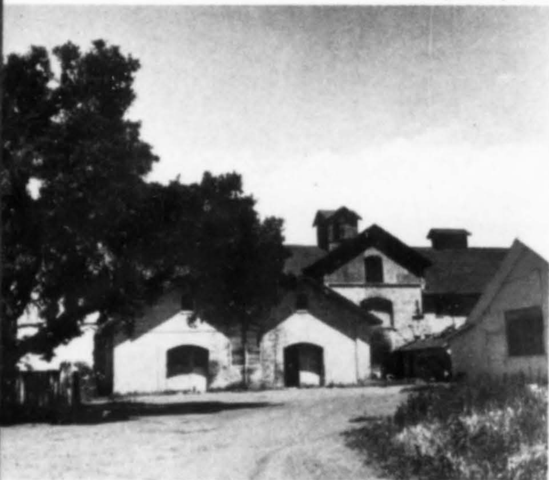
Street elevation of the old winery. At top, present street elevation after renovation. Entrance to portico is at center.
