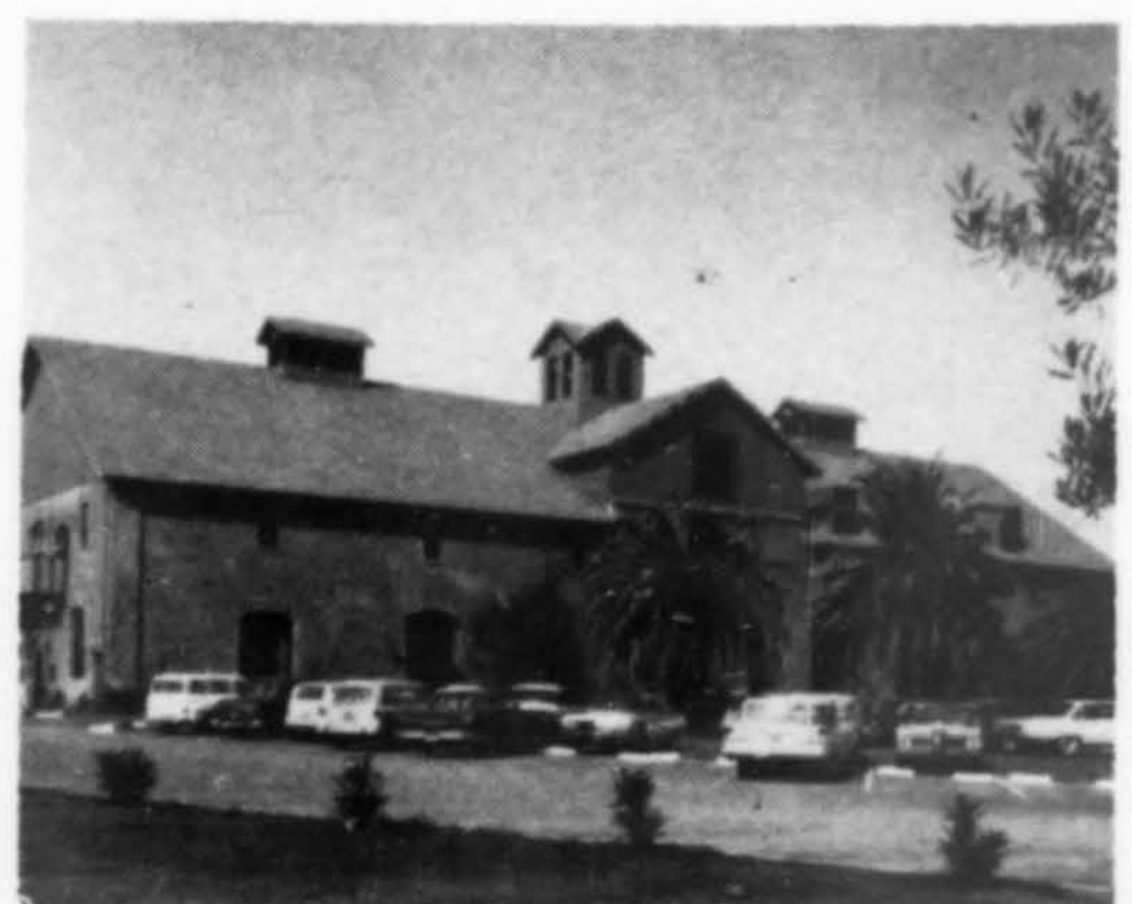
Present parking area. Note the clean lines of old winery have been retained.
