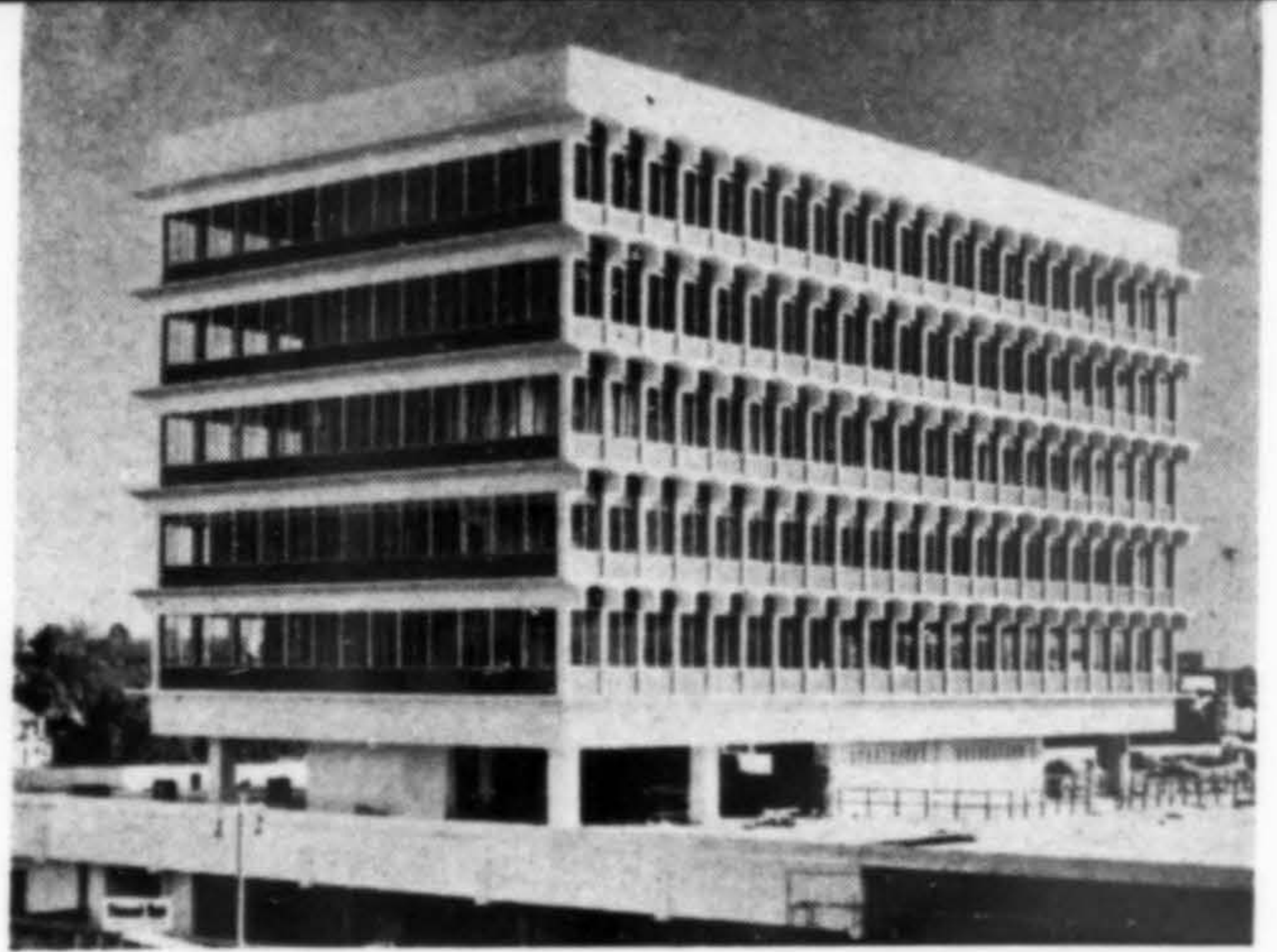
MacARTHUR-BROADWAY OFFICE BUILDING , Oakland, California. Architect: Irving D. Shapiro & Associates. Structural engineers: T. Y. Lin, Yang & Associates.
