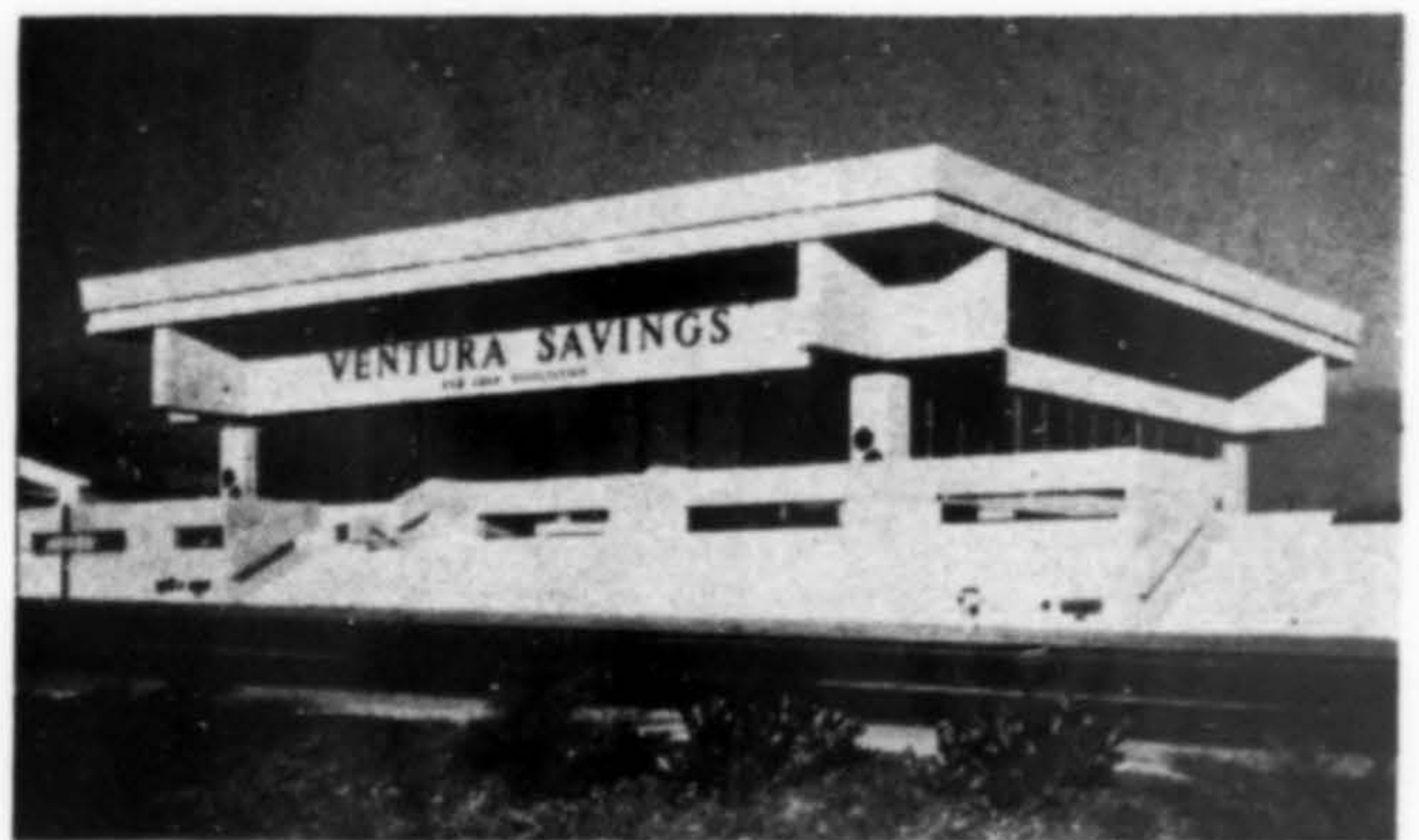
VENTURA SAVINGS & LOAN ASSOCIATION BUILDING , Buena Vista, California. Architects: William L. Pereira, FAIA, & Associates. Structural engineers: Woodward Tom Associates.
