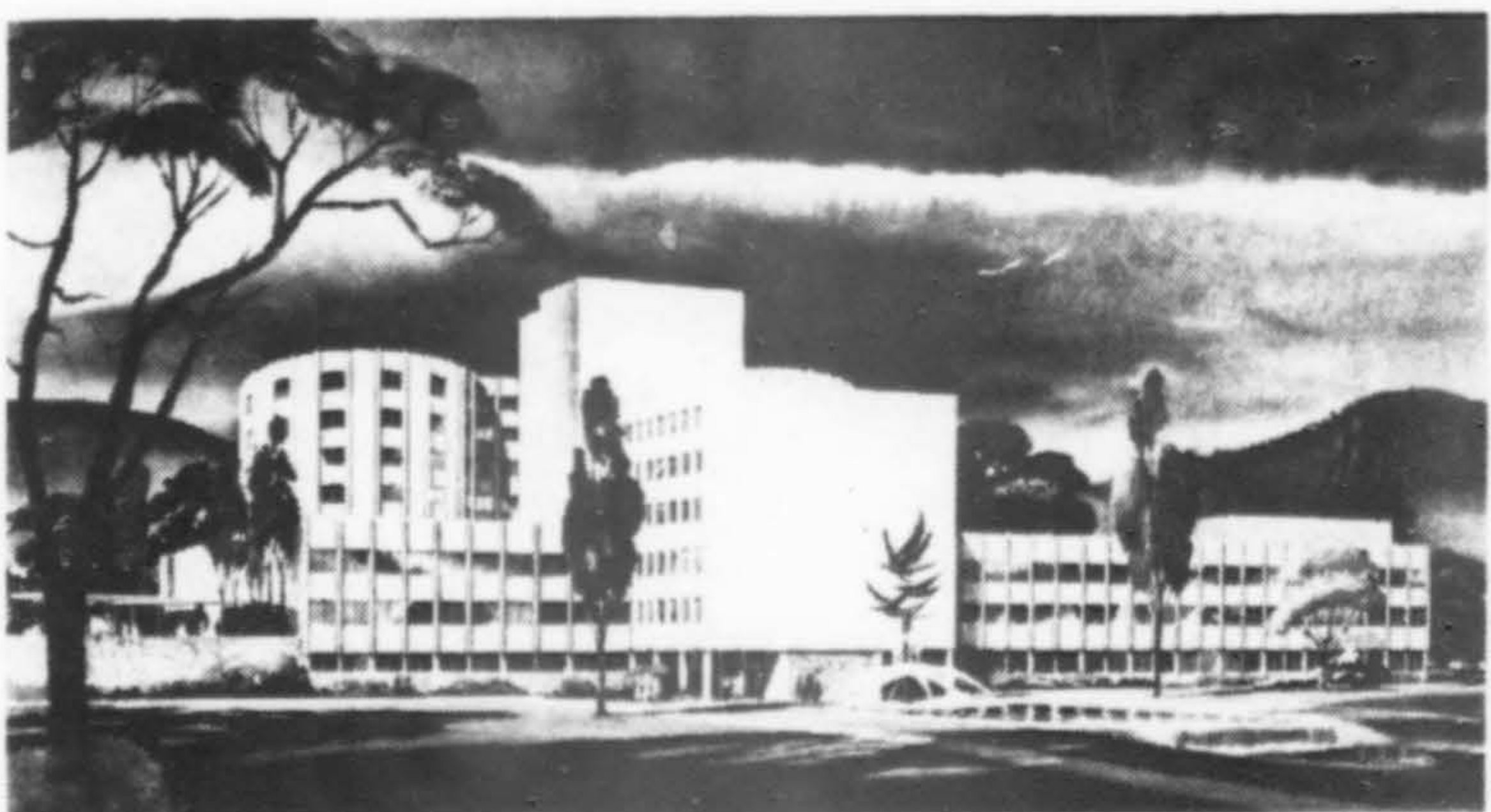
MEDICAL CENTER , Loma Linda University, Loma Linda, California, includes in first phase, facilities for teaching, medical research, out-patient clinic, 360-bed hospital (ultimately 500 bed). Four floors of rectangular design are surmounted by three circular towers connected by a service stem. Expansion plans call for two additional floors, three wings. Completion, CPM planned: spring of 1967. Estimated cost: $17.8 million. Architects: Heitschmidt & Thompson; L. C. Havstad-Del E. Webb Corp., contractors.
