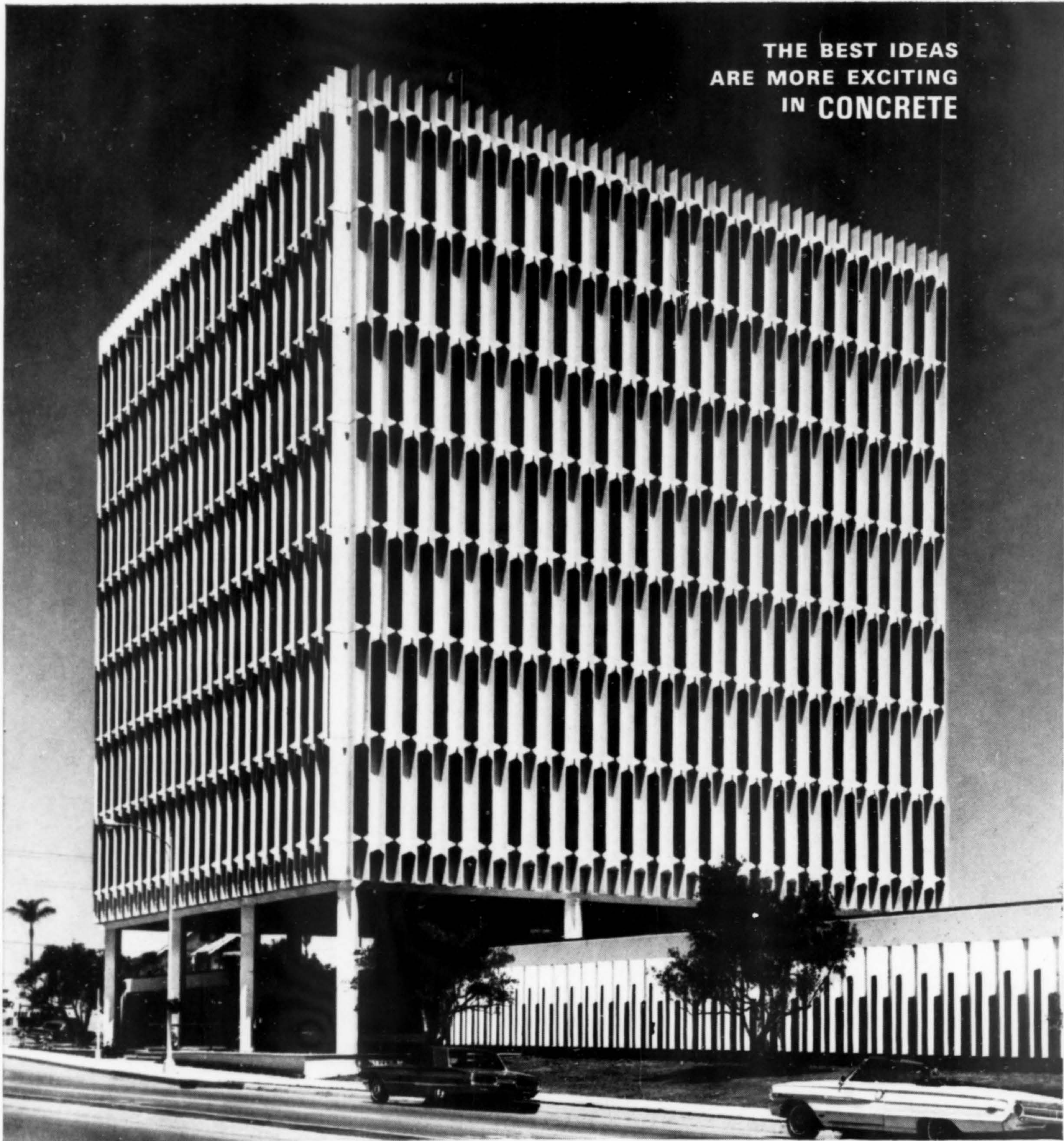
Owner: The Whitson Company, San Diego, Calif. Architect: Deems-Martin, Associates, San Diego, Calif. Structural Engineer: A. J. Blaylock and Associates, San Diego, Calif. Contractor: Peter Kiewit Sons Company, Arcadia, Calif.
