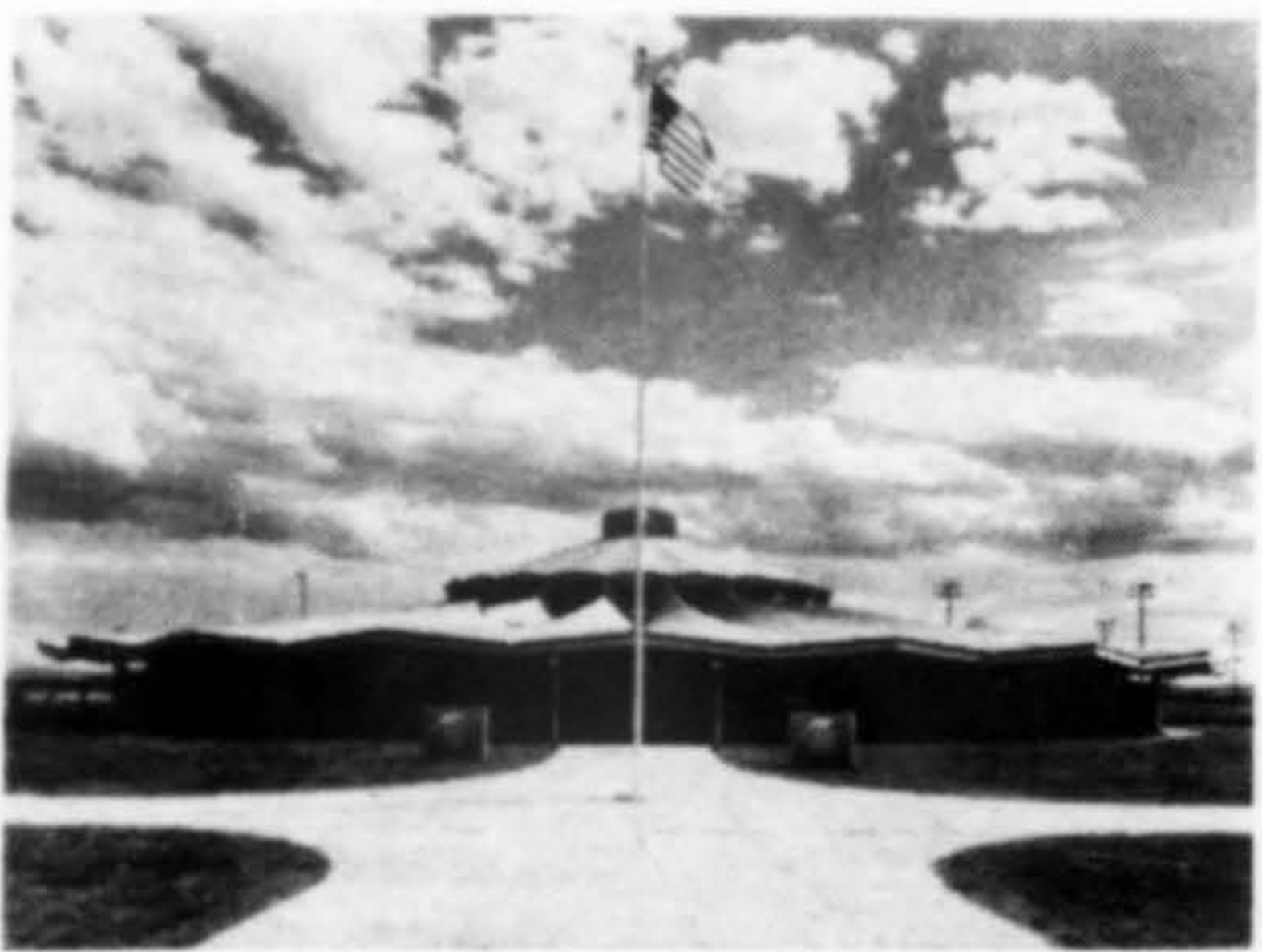
CARROUSEL PRIMARY SCHOOL , Ellsworth Air Force Base, South Dakota. Award of Merit. Gass-Gay, architects.
