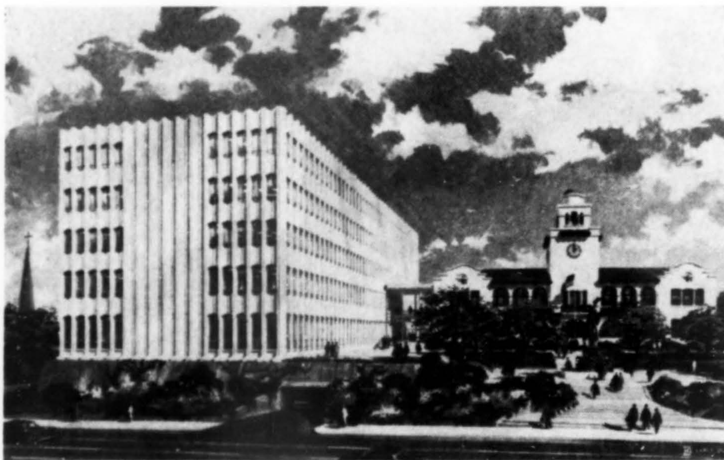
SNOHOMISH COUNTY COURTHOUSE , Everett, Wash., will be steel frame with cast stone exterior, providing space for Superior and Justice Courts, sheriff's department, jail and other county offices. Gross area of 110,000 sq. ft. and underground garage for 25 cars. Jails are mechanically ventilated, other areas air conditioned. Cost: $3,616,000. Architects: Harmon, Pray & Detrich, Seattle.
