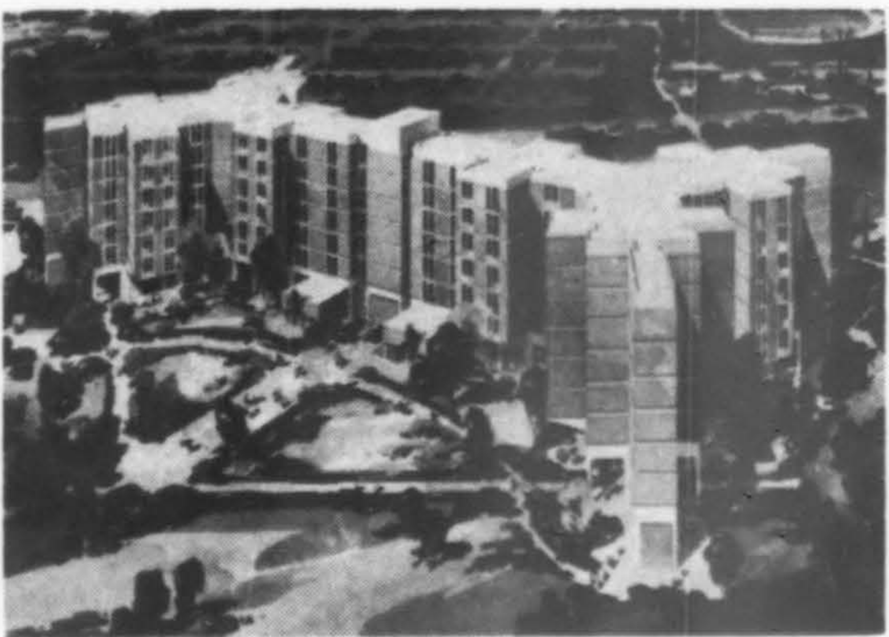
RESIDENCE HALL , San Fernando Valley State College, Northridge, California, is first unit in a planned complex of eight residence halls. The seven-story reinforced concrete and masonry building will have face brick exterior, house 306 men and 306 women. Cost: $3 million. Architects: Allison & Ribbe, Los Angeles.
