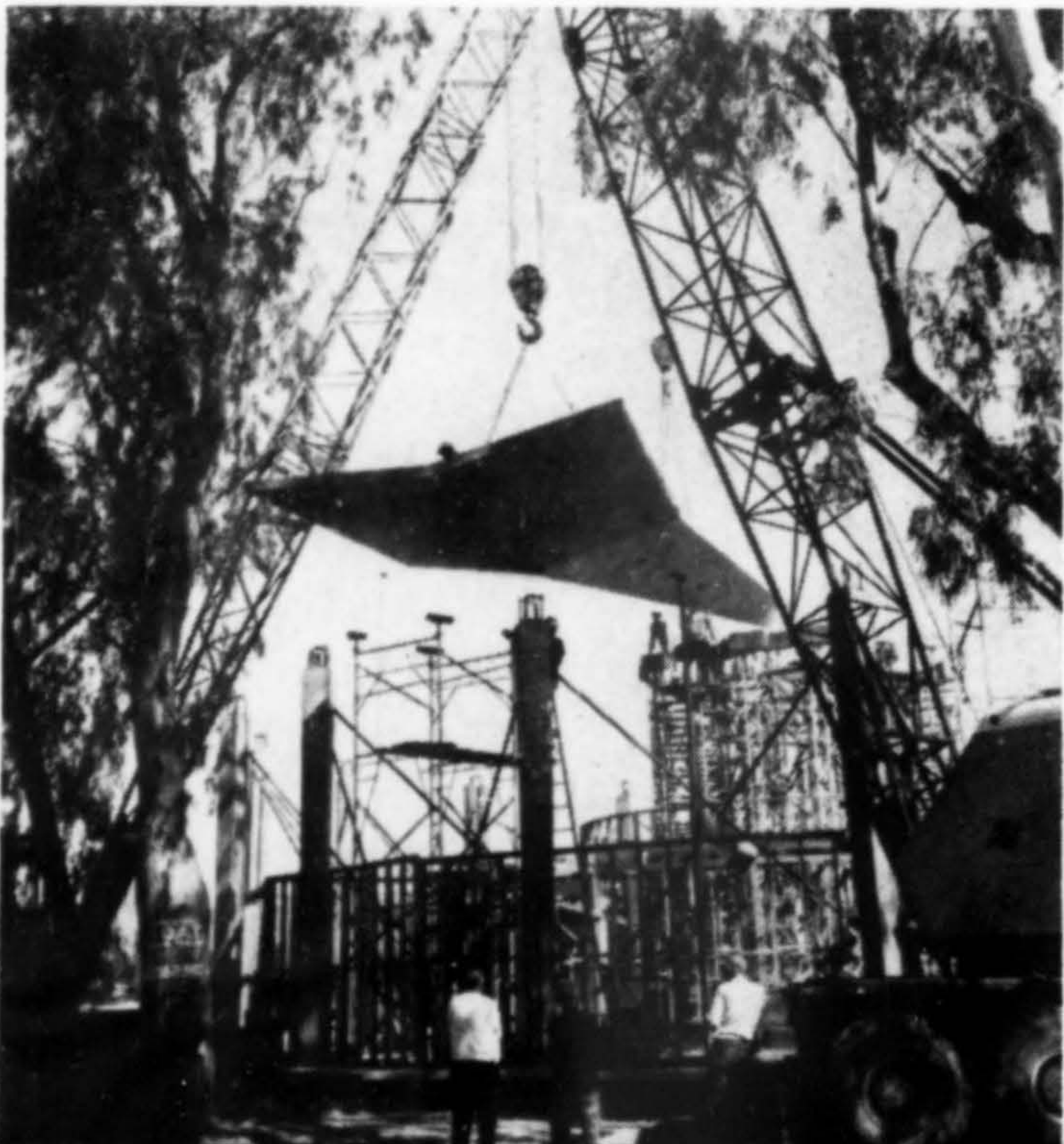
Two cranes were used in placing the segments on the columns and center shoring. A tolerance of only 8-in. was allowed between segments. After units were placed, they were welded at the tension ring and at shear plates.
