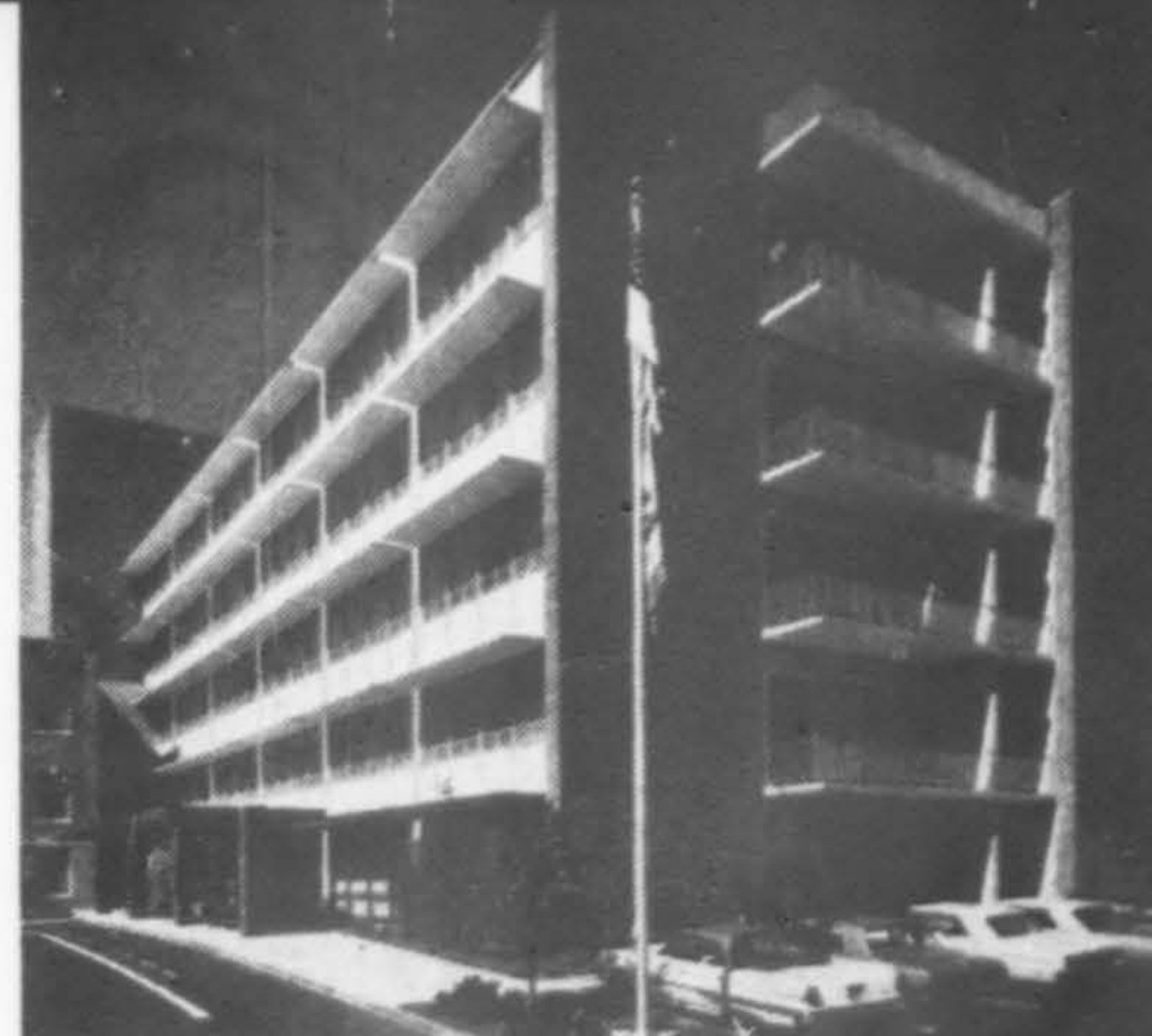
THE TOWER of Oakland's Merritt Hospital won for San Francisco architects, Stone, Marraccini & Patterson, a 1965 Masonry Honor Award. MacDonald, Young & Nelson were general contractors. Karl H. Riek photo.
