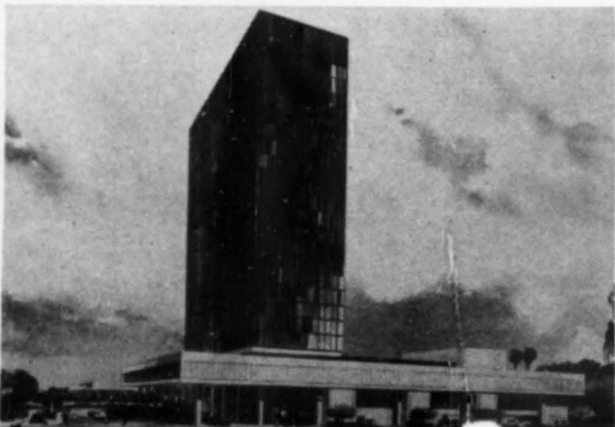
THEATER-OFFICE BUILDING , Los Angeles, will include a 2600-seat proscenium theater, to be called the Cole Porter Theater, a 24-story office building, bank, two restaurants, parking for 1300 cars on three levels beneath the complex and in an adjoining parking structure. Estimated cost: $24 million. Architects: Welton Becket & Associates.
