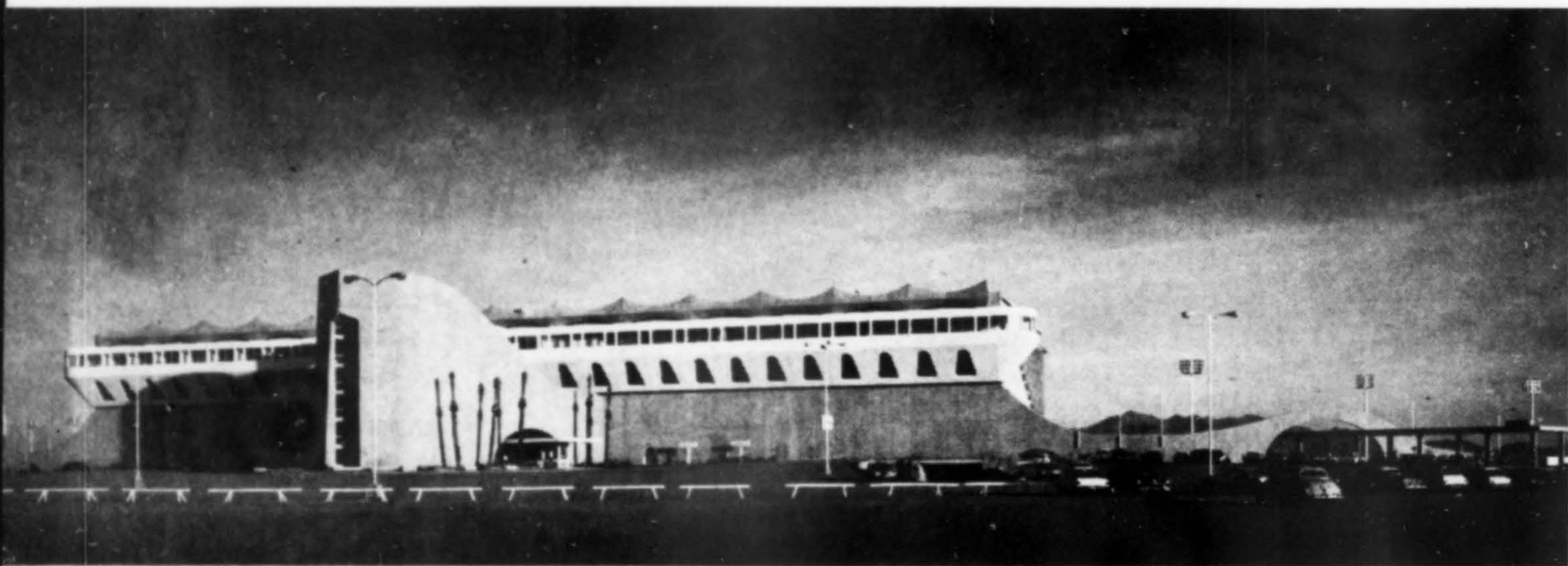
All grandstand seats have full view of the track. Concrete columns, which support the roof structure, are designed as slim as building codes allow to permit less line-of-sight obstruction.
