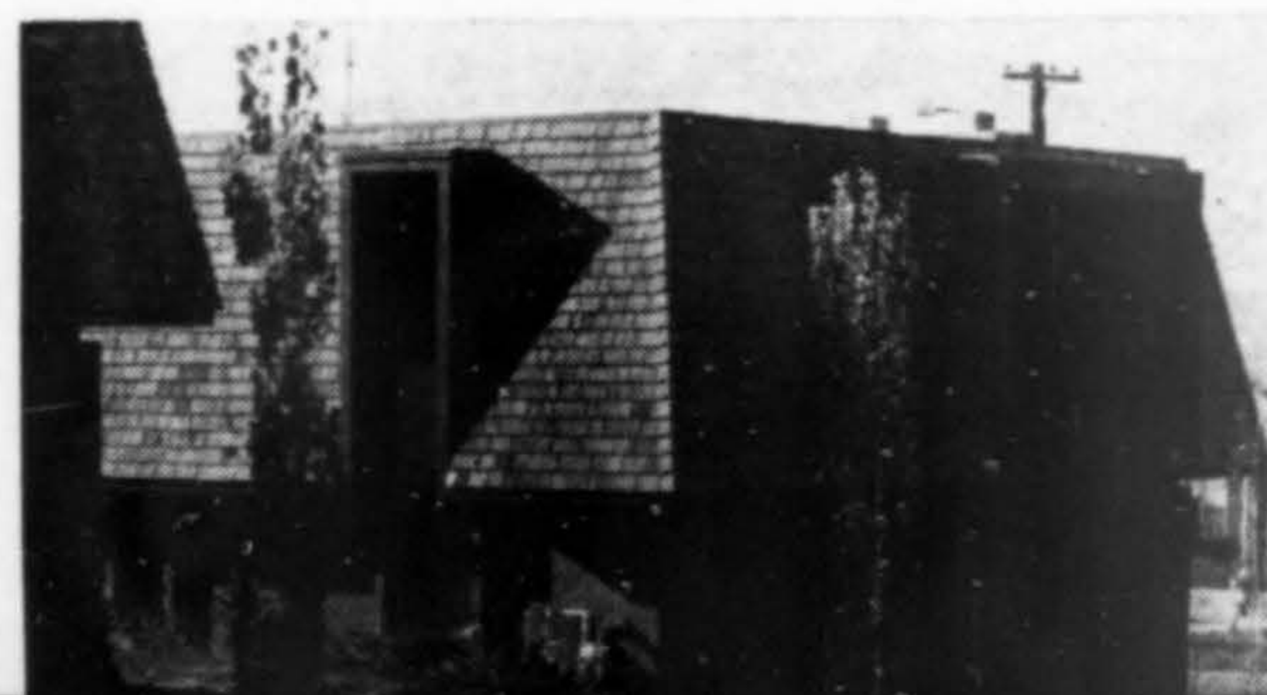
LOGAN AVENUE TOWNHOUSES, Salt Lake City, Glen Ashton Lloyd, architect.
