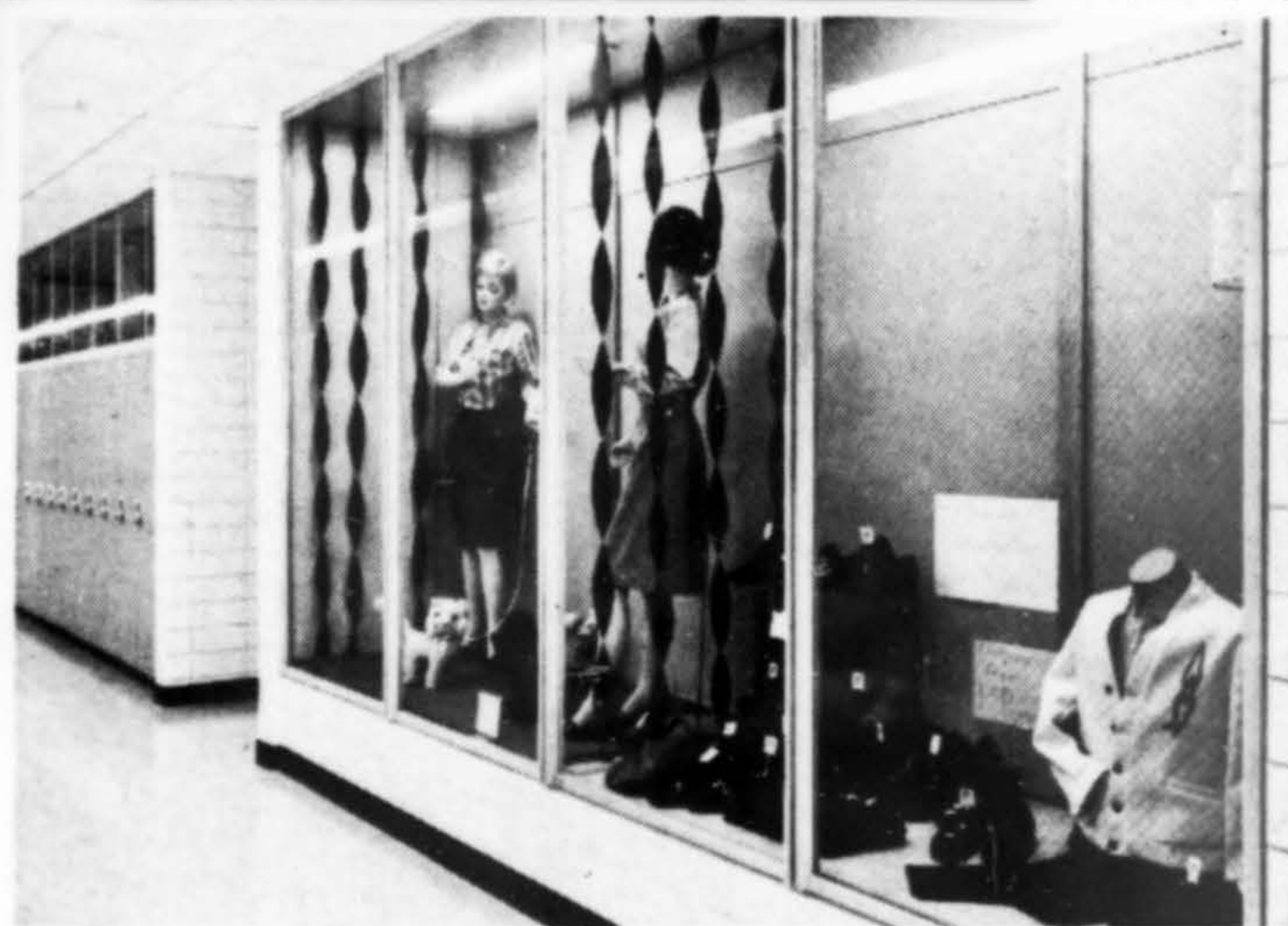
(above) Wire glass provides a safeguard against human impact in heavily trafficked corridors.
