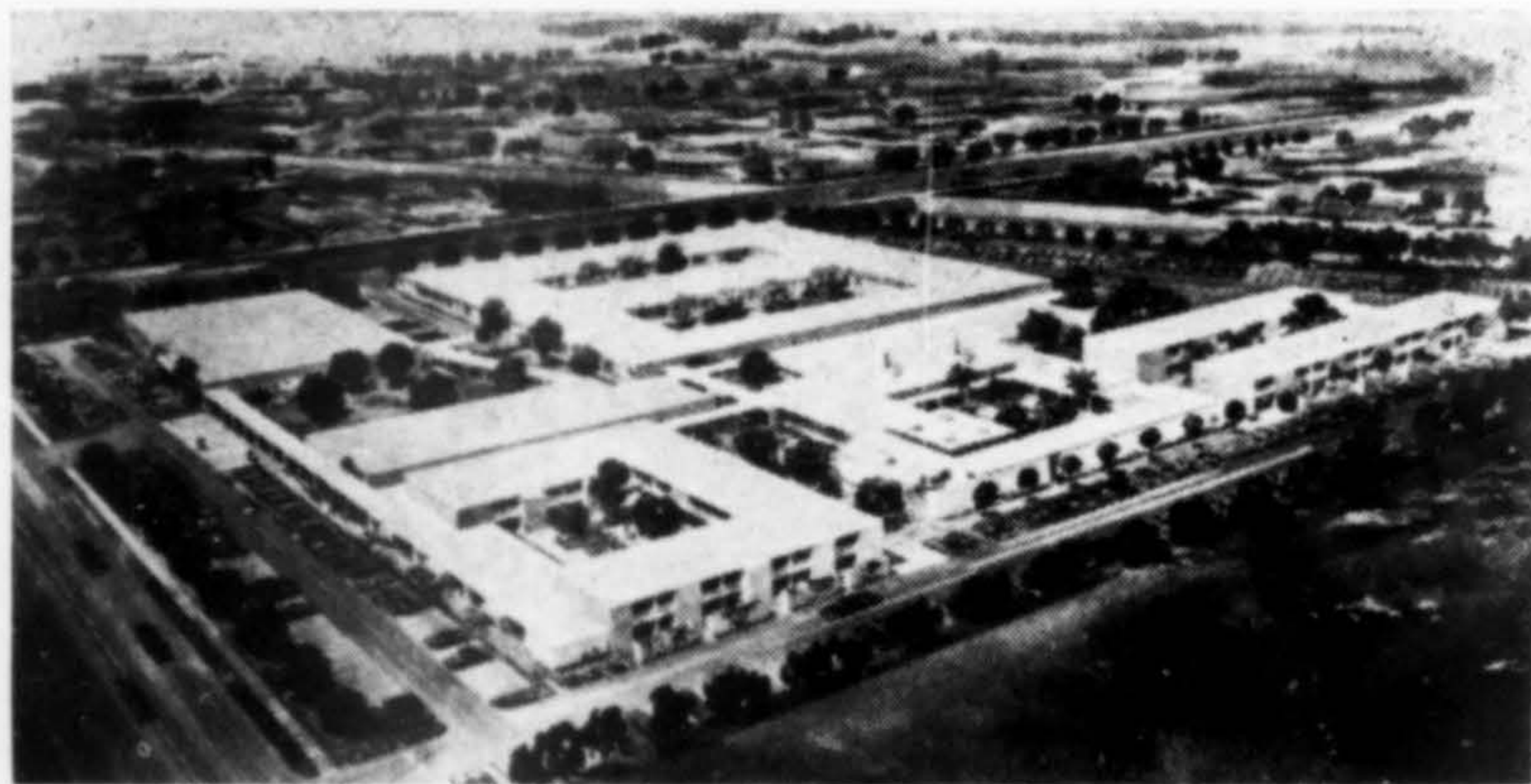
LOS ANGELES JEWISH HOME for the Aged, San Fernando Valley branch, is presently under construction. A total nine-acre project emphasizes a non-institutional concept of a series of buildings with balconies and courtyards, connected by promenades. Buildings will be reinforced concrete. Complex cost: $1 million. Architects: Mayer & Kanner, Matthew Lapota & Associates. Contractor: McIsaac & Menke.
