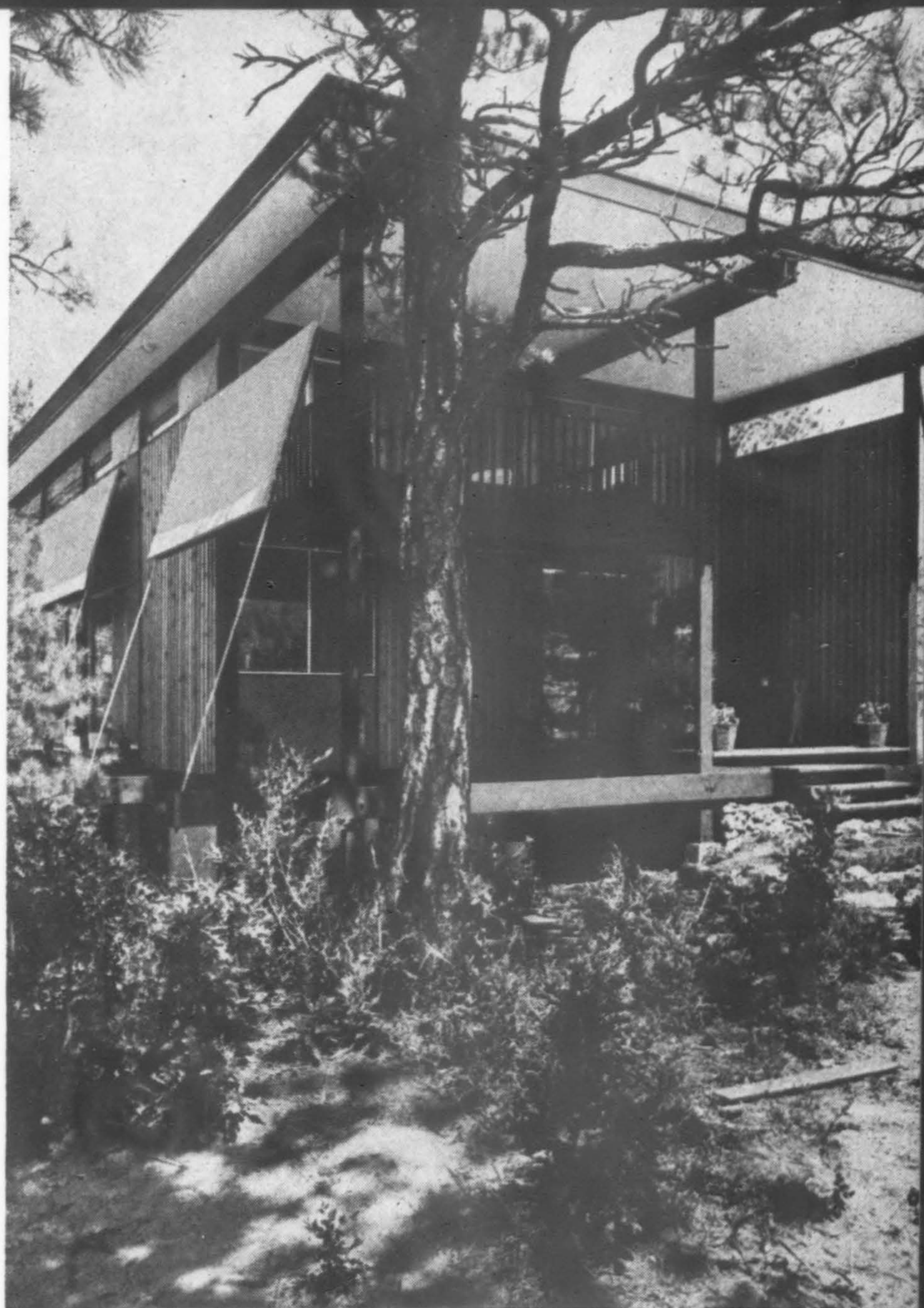
The large moving panels are a step toward an "architecture of motion" which began with the hinged shutter and the shoji and, with more reliable and sophisticated techniques, will go on to include larger movable components. This movability will increase not only functional performance of building but make possible flexible space effects as well.
