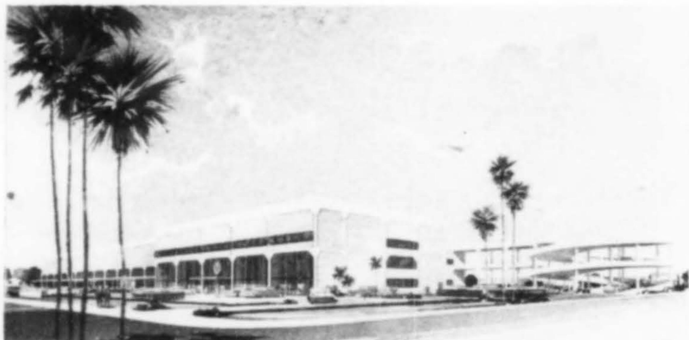
LOS ANGELES WORLDWAY POSTAL CENTER , Cargo City, Los Angeles International Airport, will be located on 7.3 acres adjacent to major arterial highway connections. The two-story reinforced concrete structure will have 386,000 sq. ft. of space with ceiling heights averaging 22-ft. A spiral concrete ramp provides access to employee parking at roof level. Architect-engineer; Daniel, Mann, Johnson & Mendenhall.
