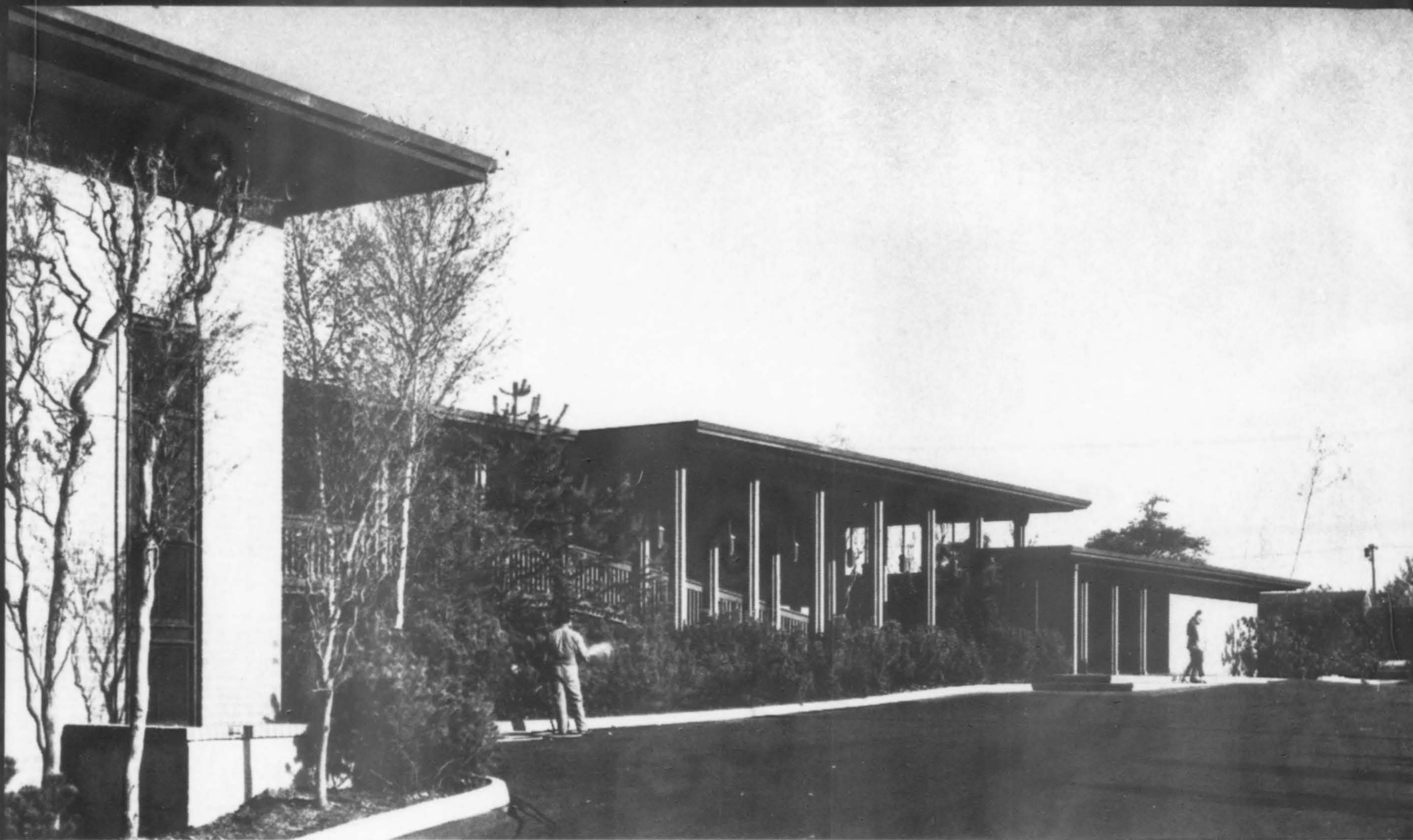
A special earth-toned color was developed for the masonry units which stage a quiet, complimentary background for extensive use of stained woods (both inside and out), native plant materials and exposed aggregate concrete paving. Grillwork shields the heat pump.
