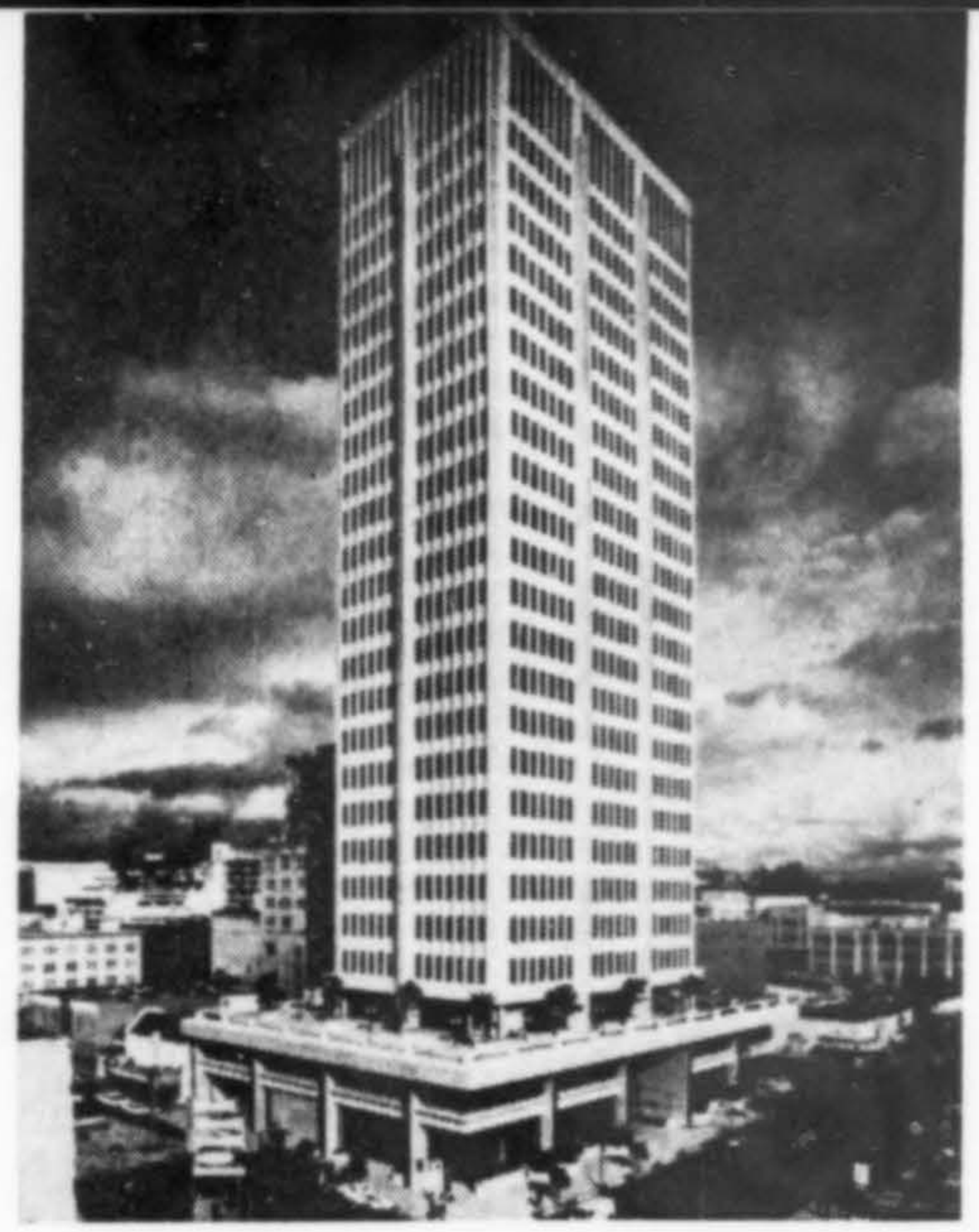
TUCKER, SADLER AND BENNETT, San Diego architectural firm, have been awarded top honors in the category of high-rise structures in the annual contest sponsored by the Prestressed Concrete Institute. The citation was for the 25-story First National Bank Building in San Diego.
