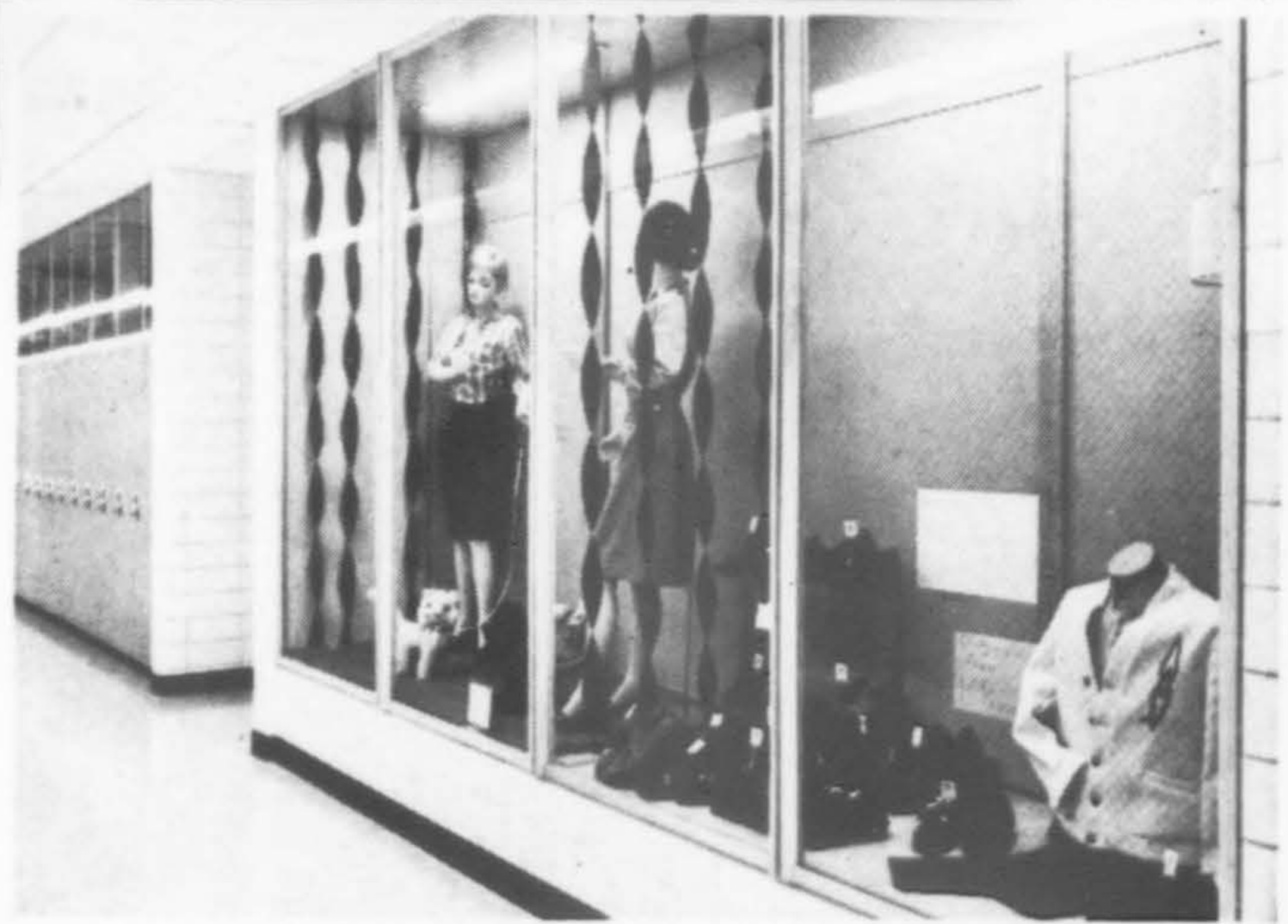
(above) Wire glass provides a safeguard against human impact in heavily trafficked corridors.
