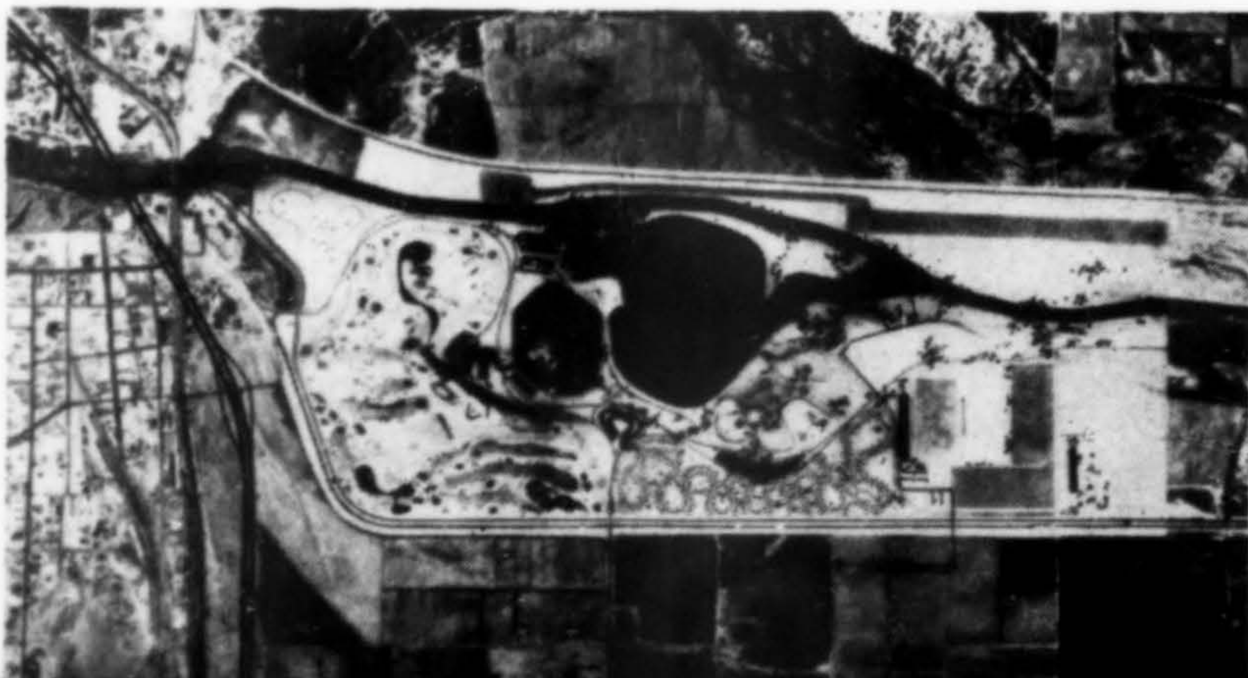
Downtown Yuma on the far left. Dark areas in center are proposed lakes.
