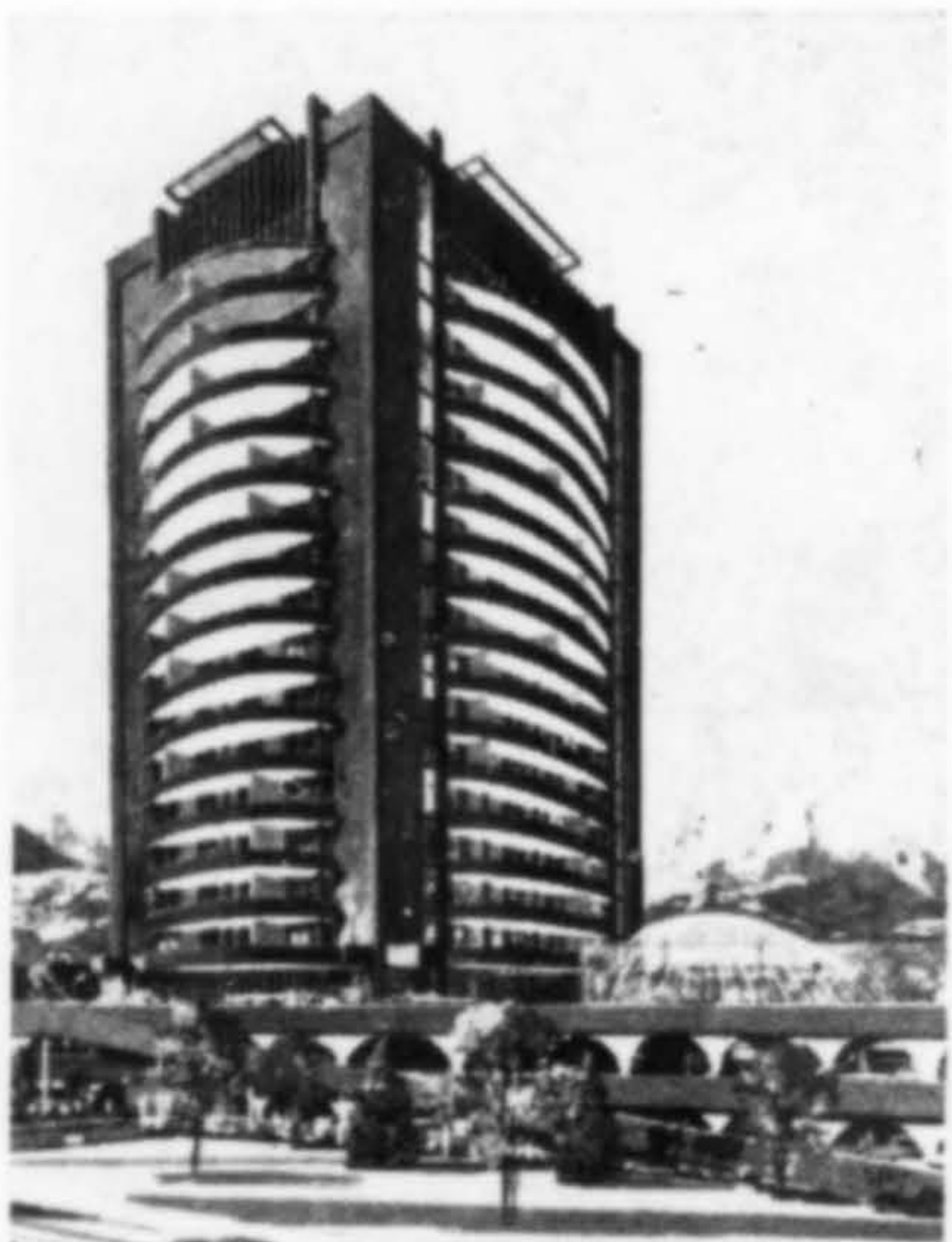
PARK TOWERS condominium, Colorado Springs, Colorado, will range from two to five bedrooms, have two-story penthouse suites. The 21-story structure will provide covered parking in two levels at the third floor. Every unit will be a corner apartment with two balconies. Cost: $4 million. Architect: Austin R. Siegfried; J. L. Williams & Co., contractor.
