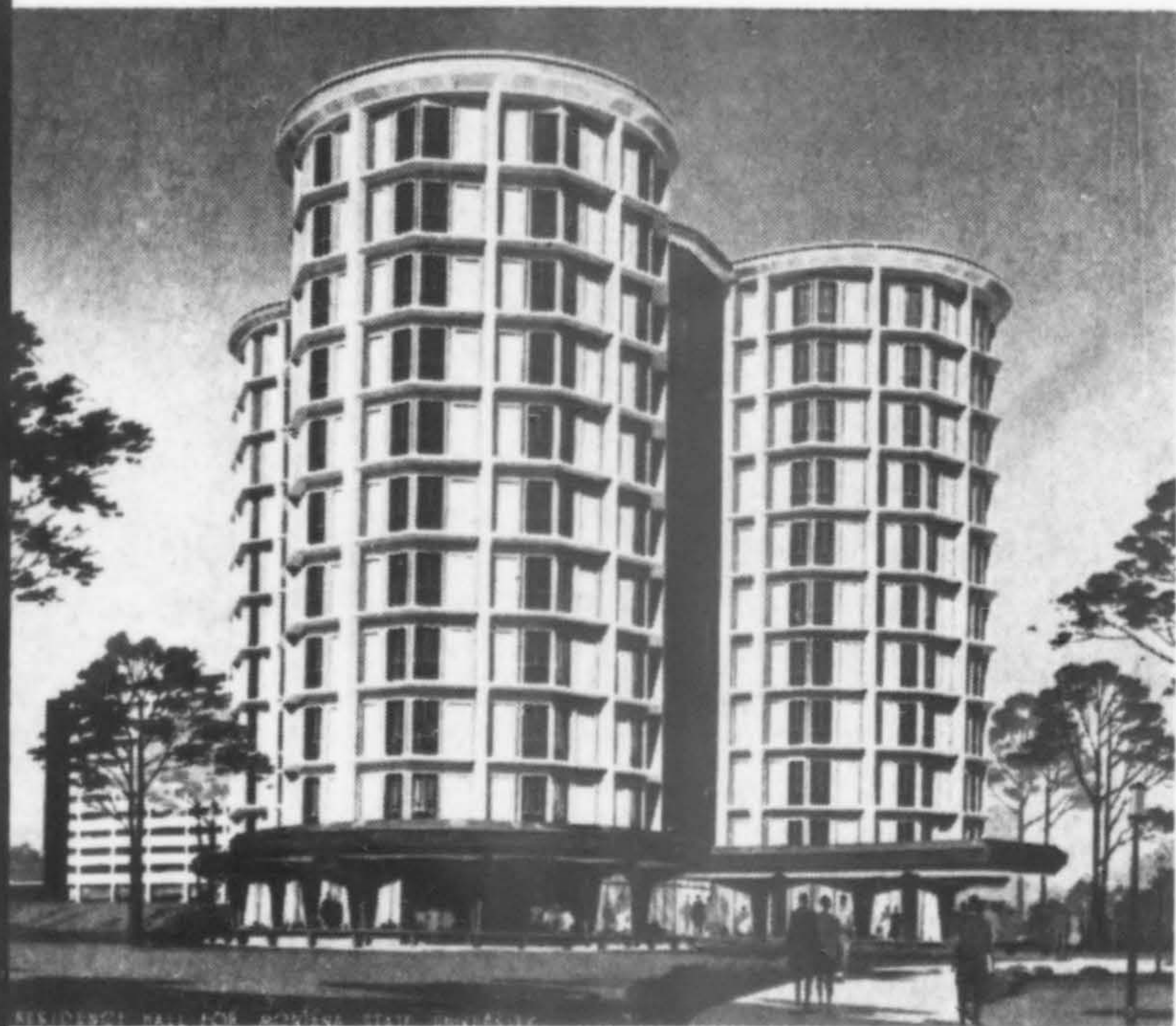
RESIDENCE HALL COMPLEX , Montana State University, Bozeman, Montana, was designed on basis of 450 students per unit. The 10 floors have each been sub-divided with 15 students in each living unit, tied together by a central core, housing elevators, lavatories, laundry, seminar room and the head resident. The building is primarily flat slab construction on steel columns. Cost: $2,000,000. Architects: Oswald Berg, Jr. & Associates.
