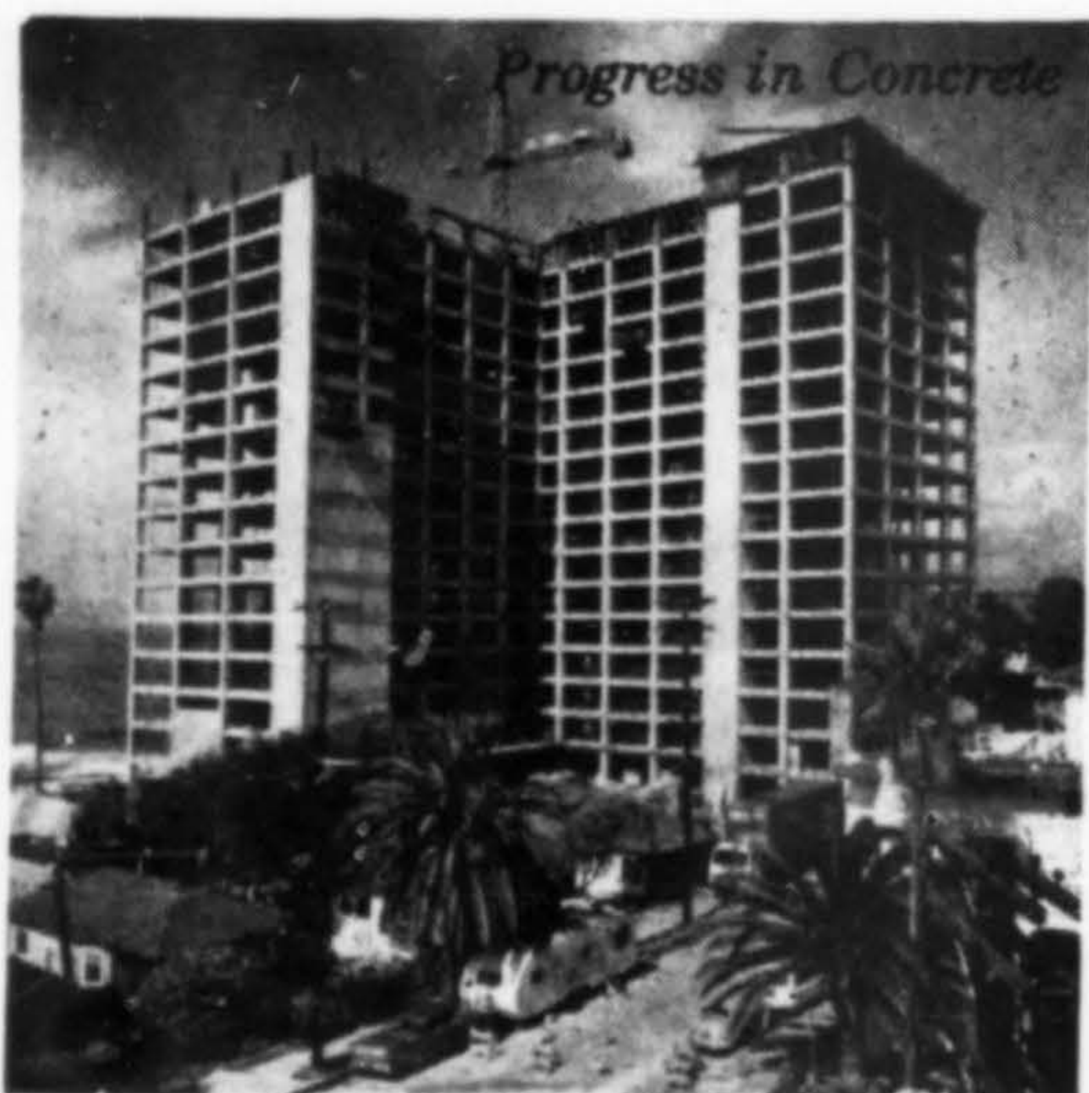
SYMONS SLAB SHORE CUTS DECK TIME FROM 5 TO 4 DAYS
