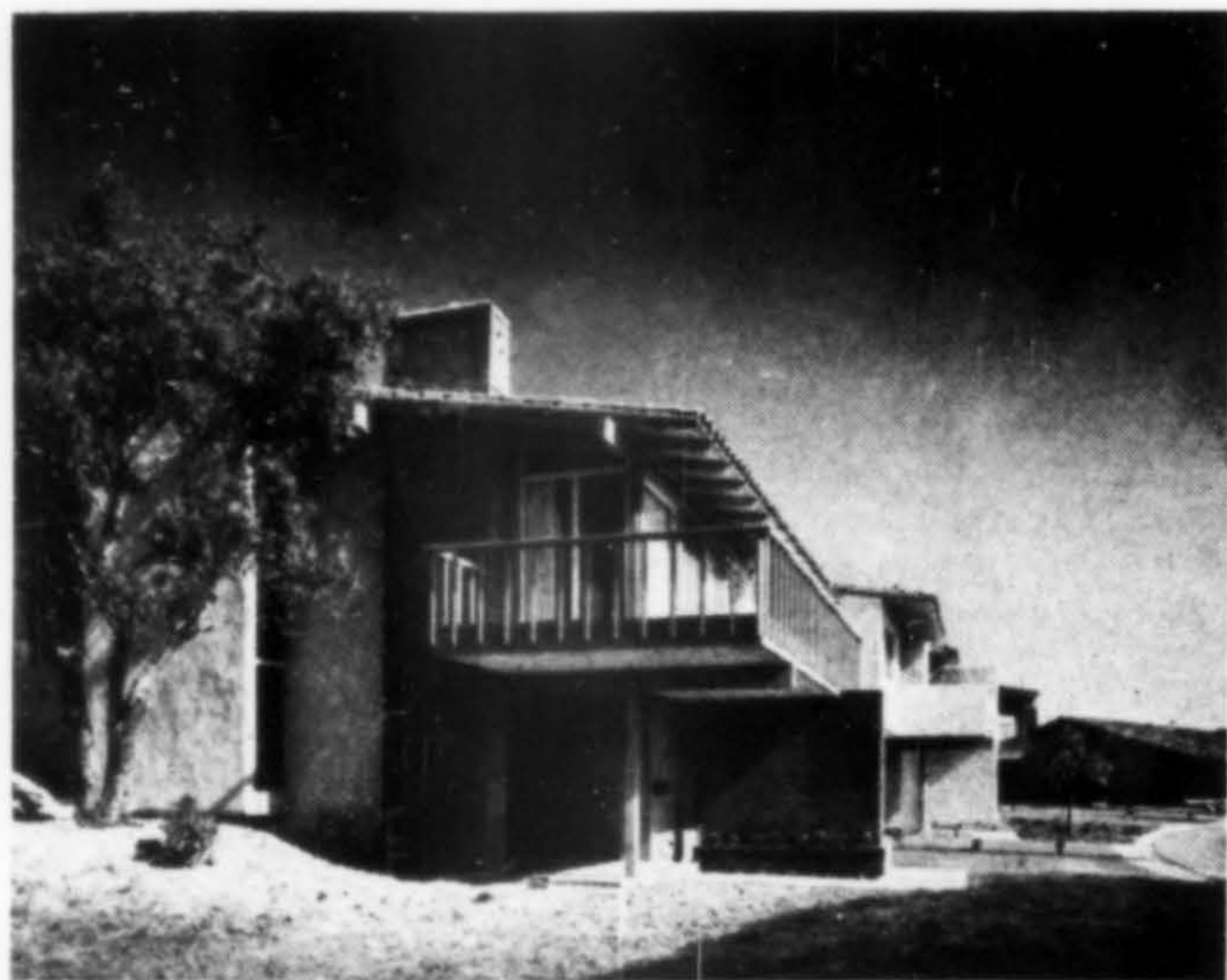
BLUFFS RESIDENTIAL DEVELOPMENT , Newport Beach, for George M. Holstein & Sons. Honor Award. Architect: Richard Leitch & Associates.
