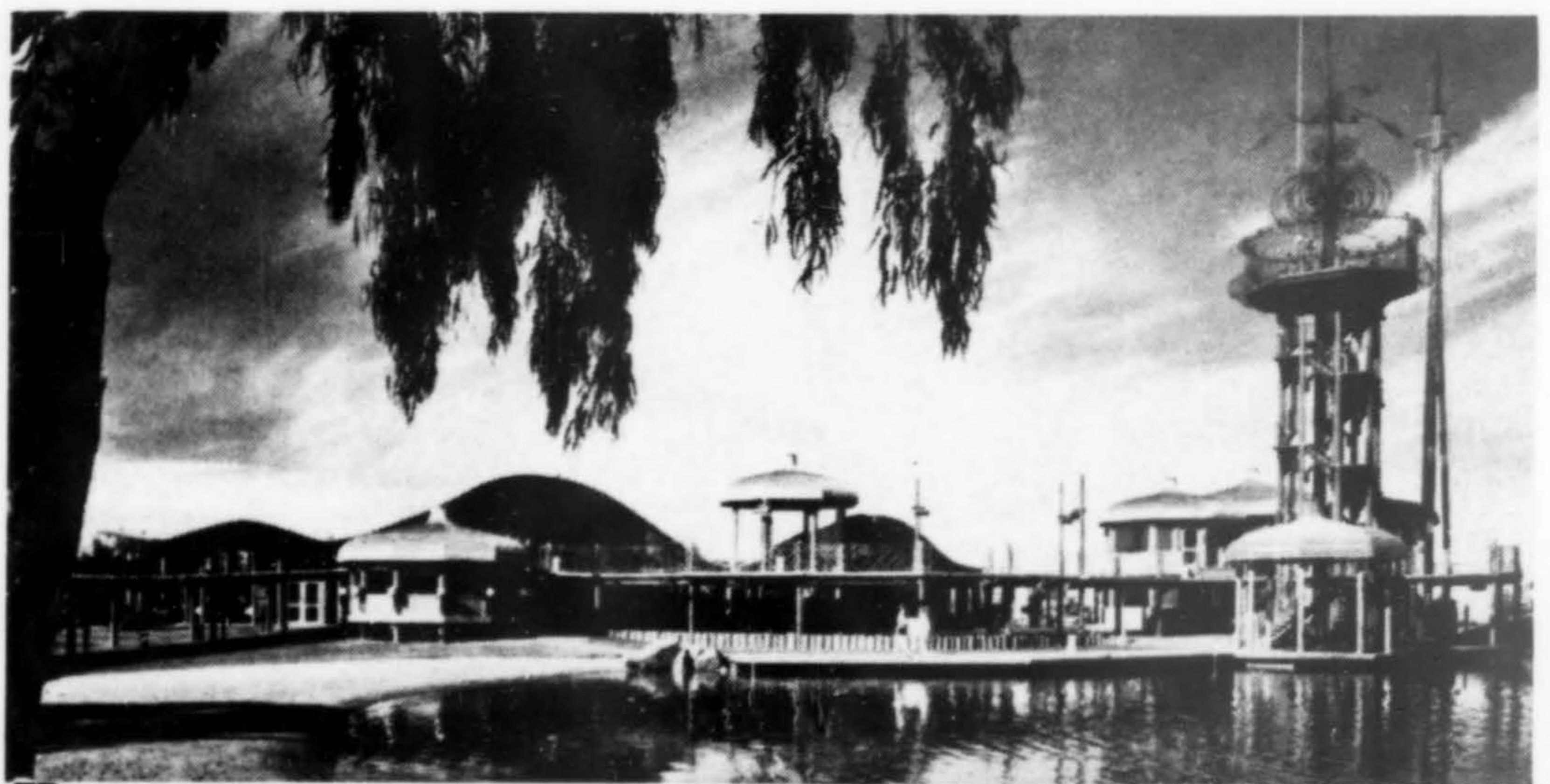
Mission Bay project at San Diego was cited by the AIA for "excellence in community architecture".
