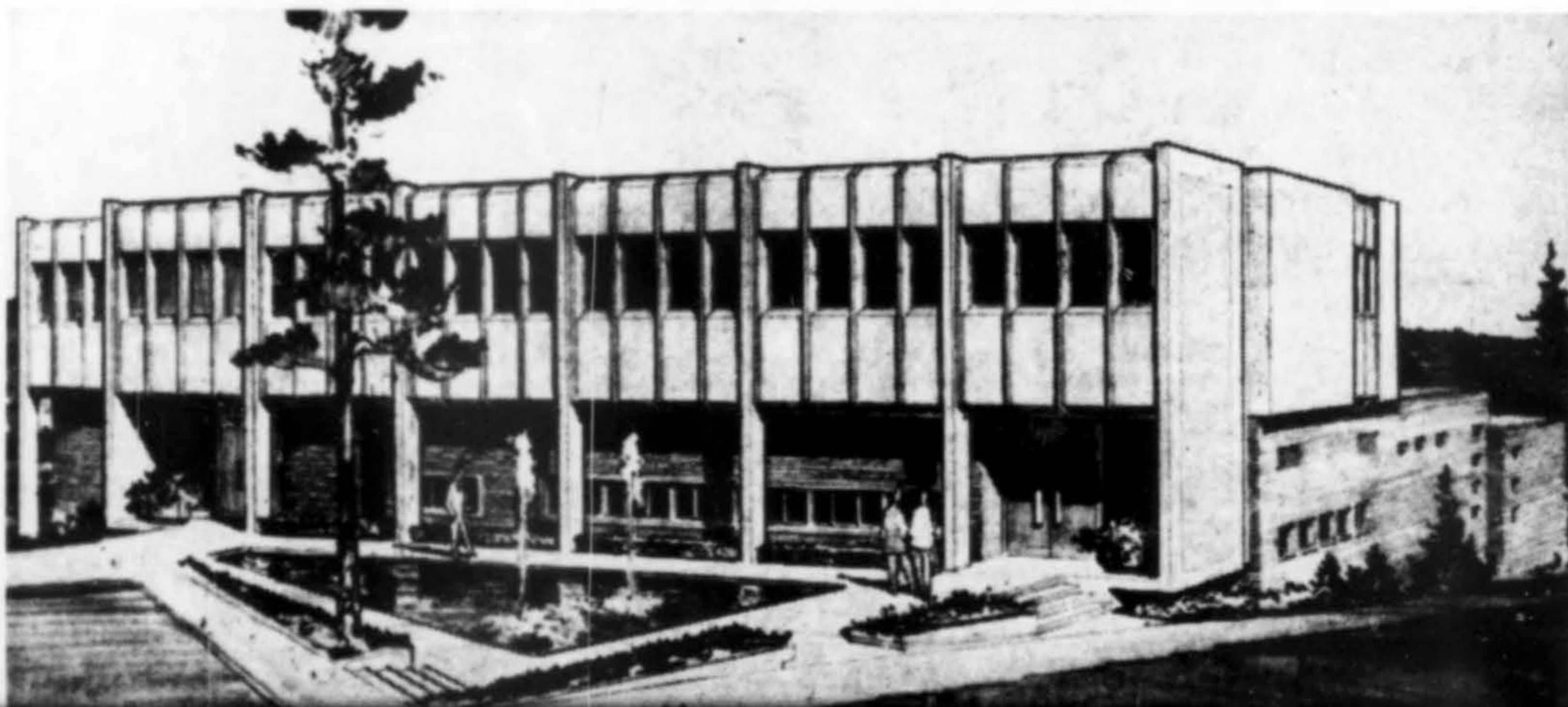
WATER RESEARCH CENTER , Washington State University, Pullman, Washington, is of structural steel and precast, prestressed concrete columns with Marblecrete and brick veneer. Included are classrooms, office and library. Cost: $186,100. Architects: Carlson & James; Lyerla & Peden, structural engineers; C & S Builders, contractor; Phil Keene, university architect.
