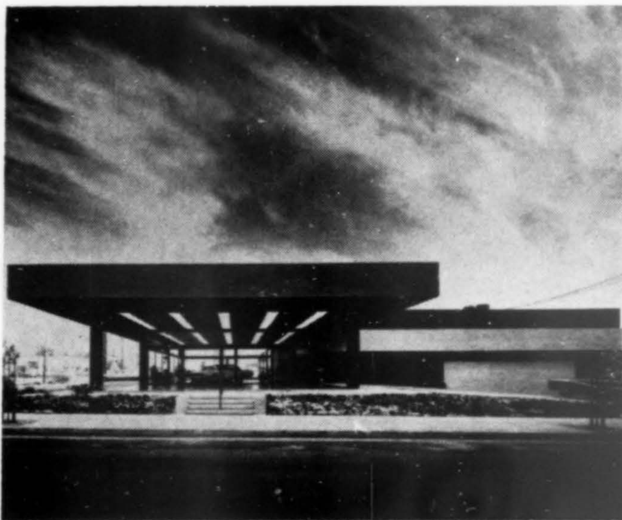
BILL HOPKINS LINCOLN-MERCURY AGENCY, Torrance. Honor Award. Daniel Dworsky & Associates, architect.
