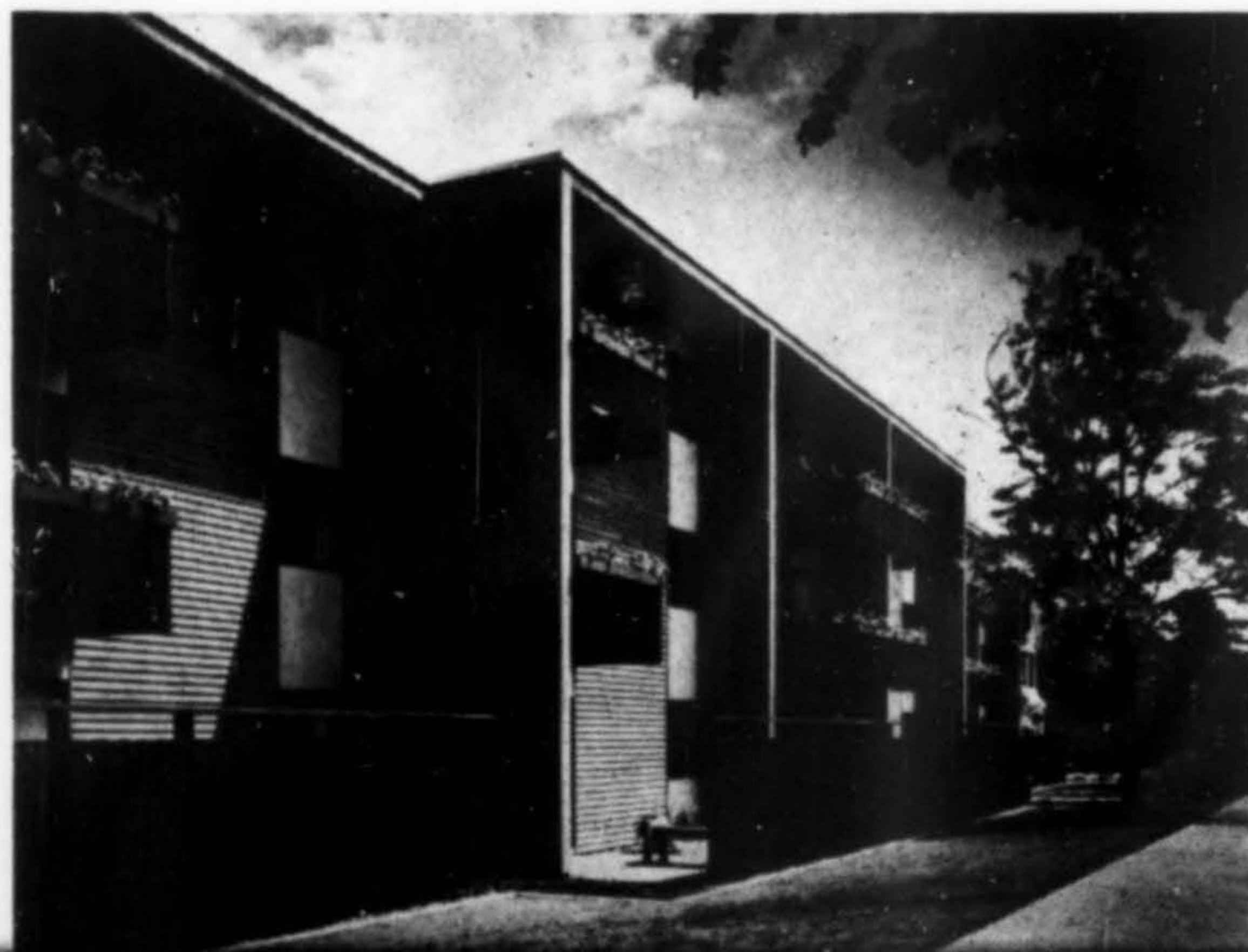
HOUSING FOR ELDERLY , 911 North K Street, Tacoma, Merit Award; Robert Billsbrough Price & Associates, architects.
