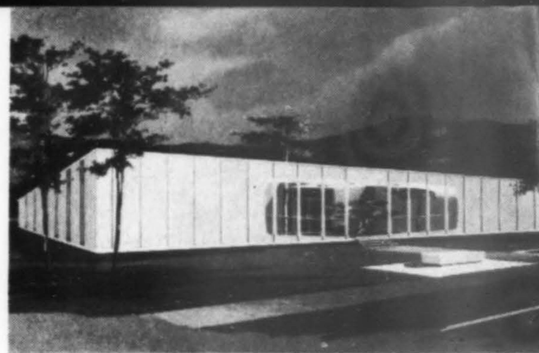
American Numismatic Association building, Colorado Springs, Colorado. Building is sited on the Colorado College campus adjacent to the Fine Arts Center and Colorado College Fine Arts School. The exterior surface is Schokbeton concrete with vertical ribs sandblasted. Architect: Carlisle B. Guy.
