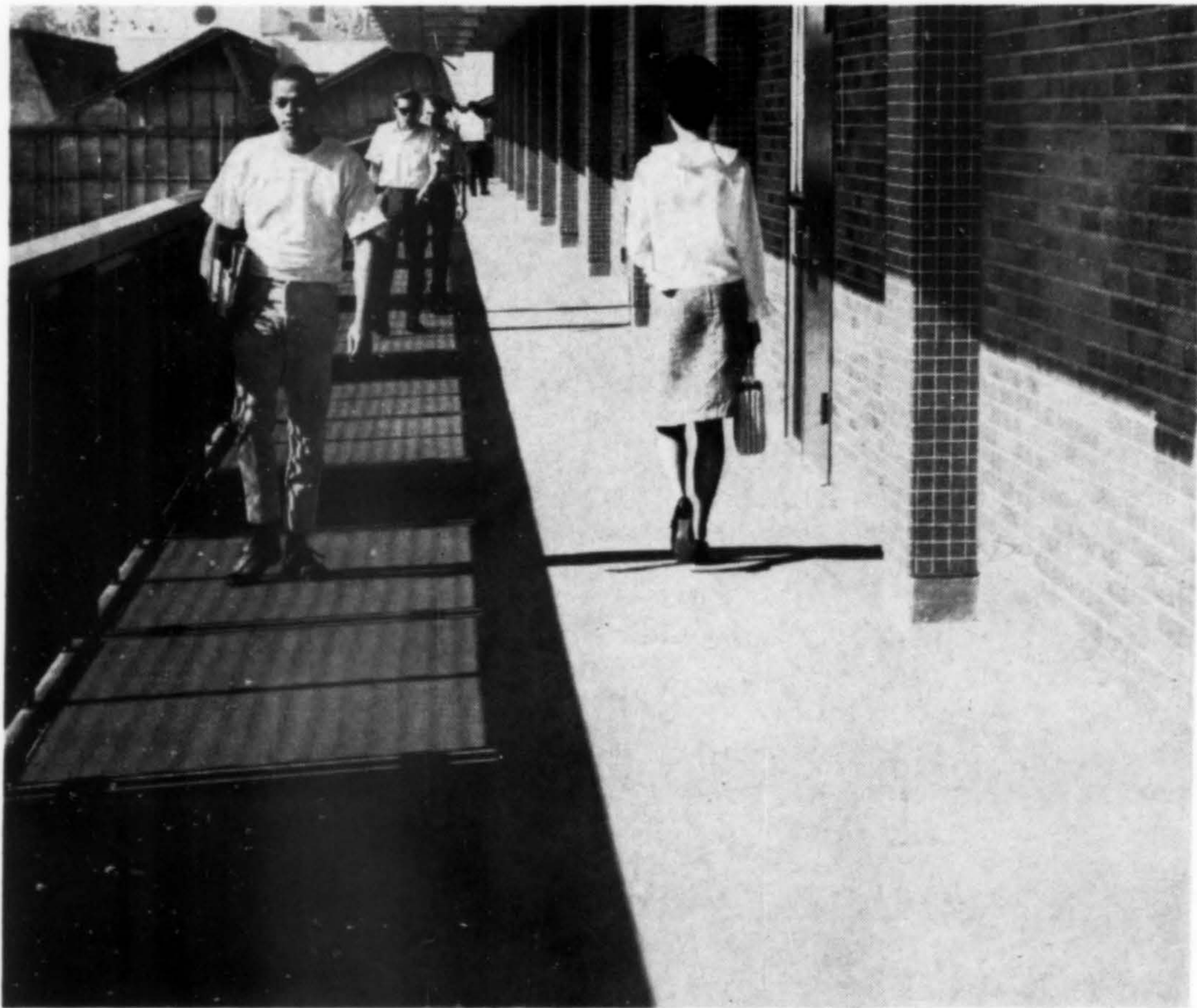
Technology Bldg., Pasadena City College, Pasadena, Calif. Architects: Allison & Ribble. Applicator: Owen Roofing Co., Los Angeles.
