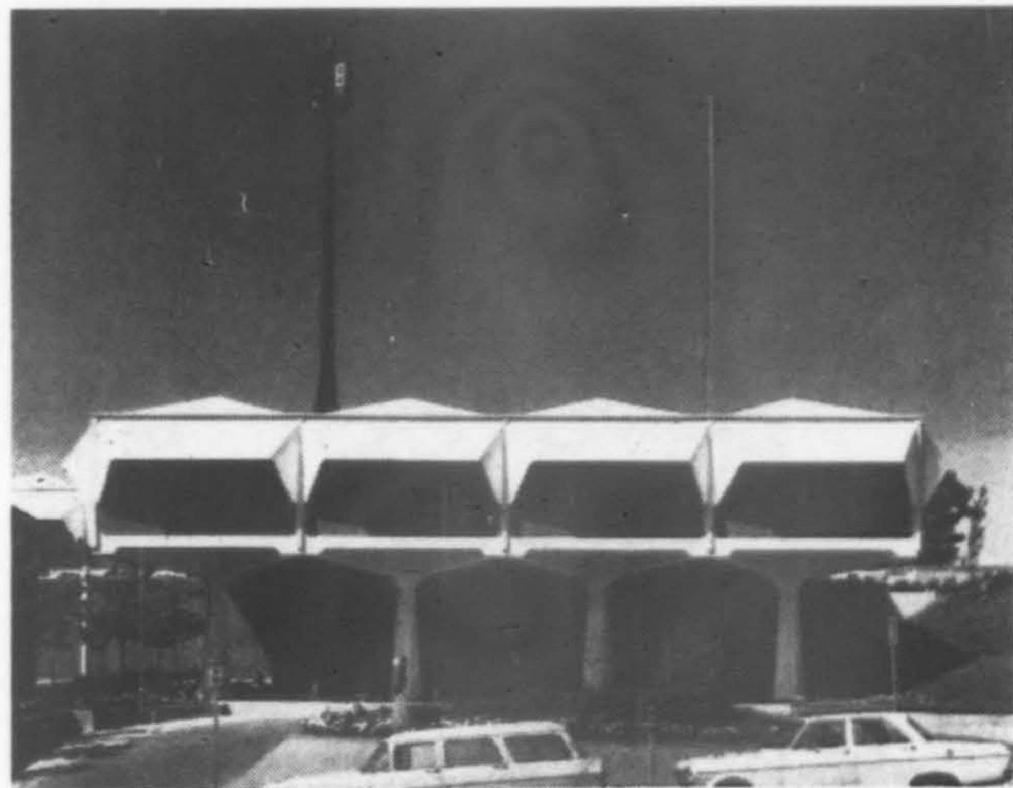
KGW RADIO & TELEVISION STATION , Portland, Oregon; Fred Bassetti & Company, architects.
