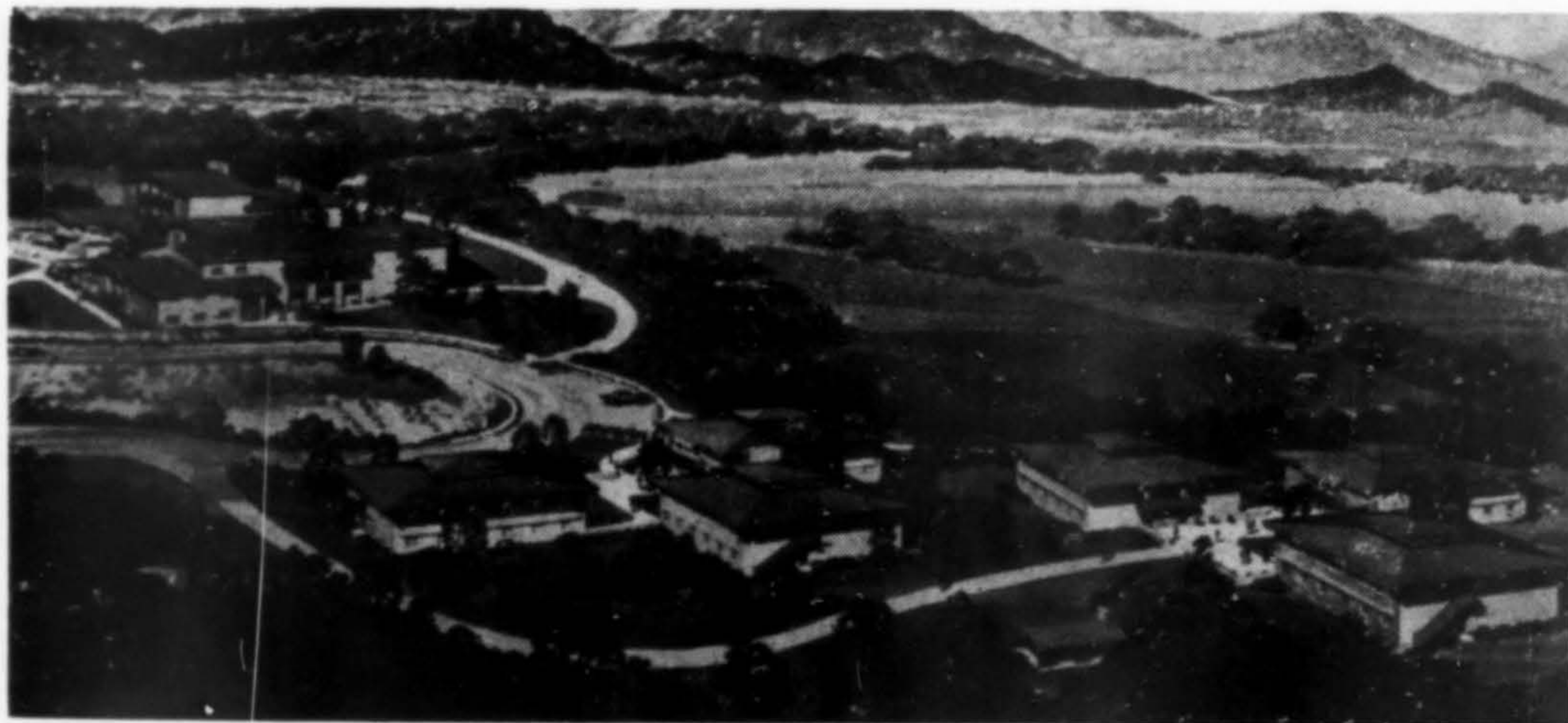
STUDENT CENTER and residence halls, Ft. Lewis College, Durango, Colorado, will provide cottage style living. The six two-story residences will house 50 students each. Construction will follow the traditional natural stone design of the present campus buildings. Cost: $1,638,000. Architect: James M. Hunter & Associates; R. W. Mier Construction Co., contractor.
