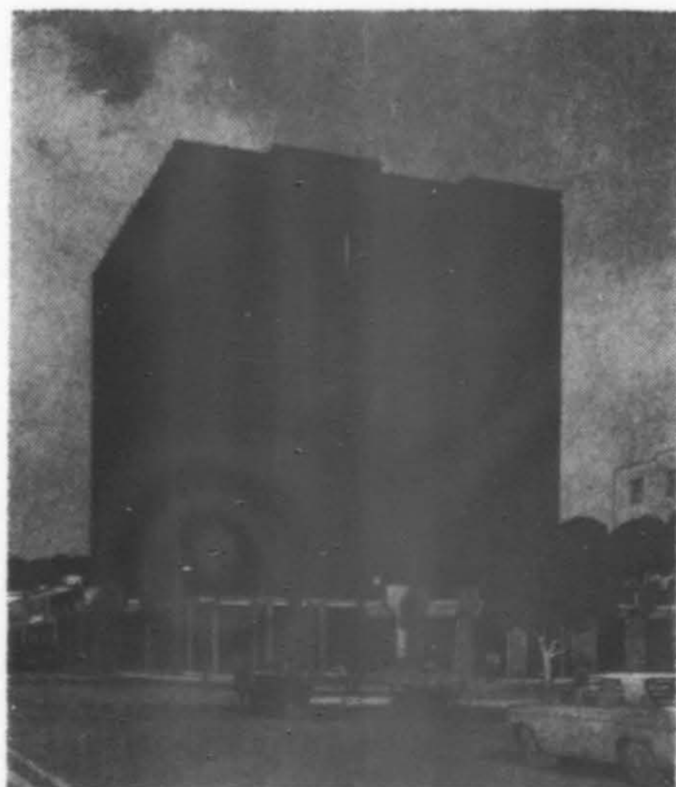
EIGHT-STORY OFFICE BUILDING , Berkeley, California, will be the largest, tallest structure built in the city proper (aside from U. of C. structures) in over 40 years. A second floor restaurant with roof garden is planned in the 55,000 sq. ft. building, located near the Rapid Transit station and the campus. Estimated cost: $1,800,000. Occupancy: February 1968. Architect: L. L. Freels & Associates.
