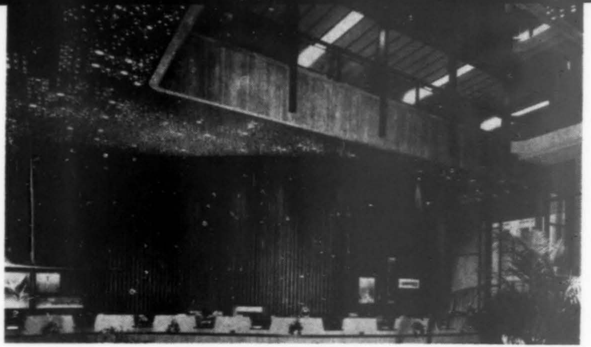
In the new Prudential Federal Savings & Loan Association building in Salt Lake City, designed by William L. Pereira & Associates, a lighted ceiling system, "Celestial," was selected to illuminate the main banking floor and part of the exterior first floor overhang. Its all-incandescent lighting sources supply the drama of the crystal chandelier, the 300-watt downlights producing approximately 75 ftc of light over the tellers areas. The viewer sees clusters of "stars" above from water-clear acrylic prisms.
