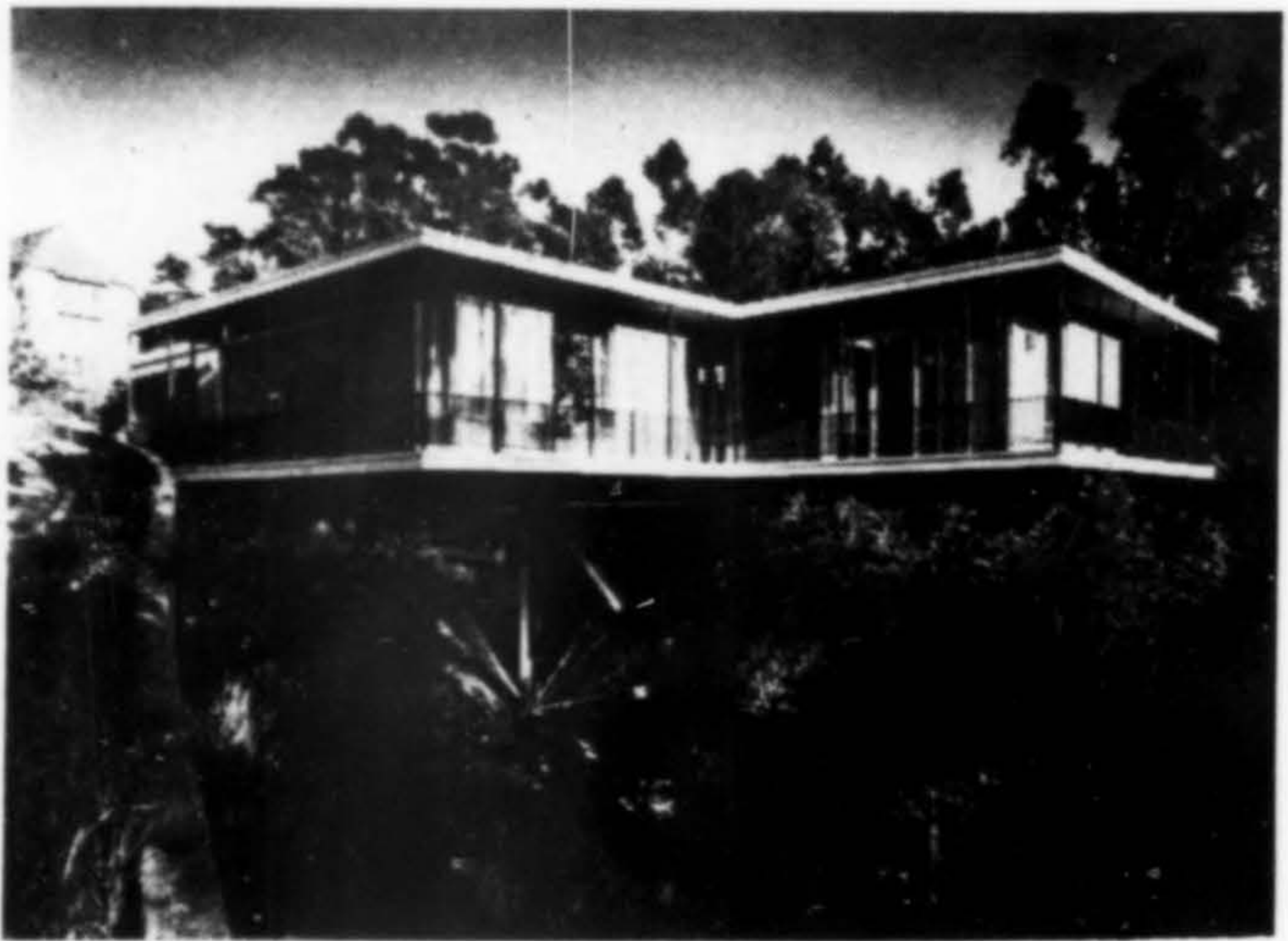
Twin residence halls at Central Washington State College, Ellensburg, Washington (top photo), won for architect Ralph H. Burkhard and engineers Anderson, Birkeland, Anderson & Mast, the top award for best engineering for high-rise or institutional construction. (Lower photo) The steel-framed house on a hillside won for Campbell & Wong & Associates, architects, the first award in best design for residential construction.
