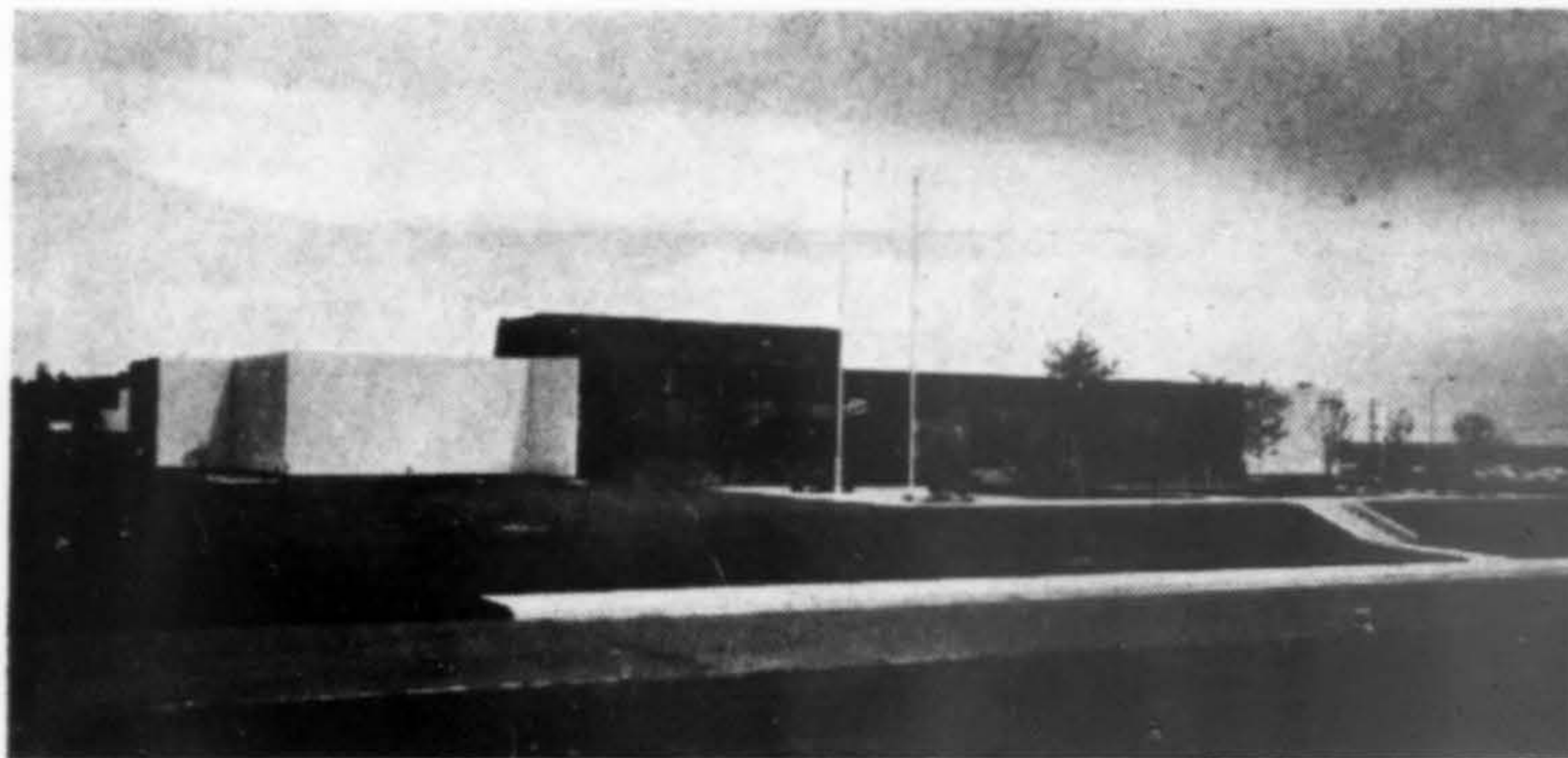
AMPEX CORPORATION , Colorado Springs, Colorado; Lusk & Wallace, architects.
