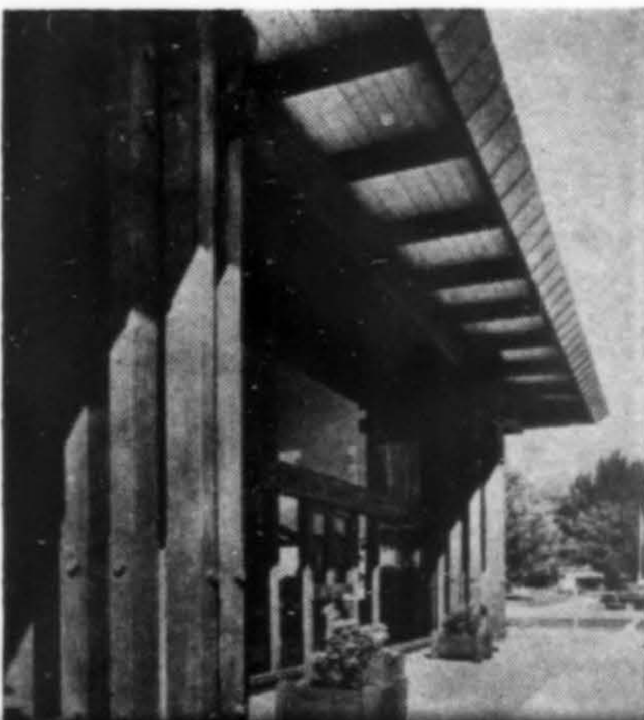
REDWOOD NATIONAL BANK , Napa, California; Neill Smith & Associates, architect.
