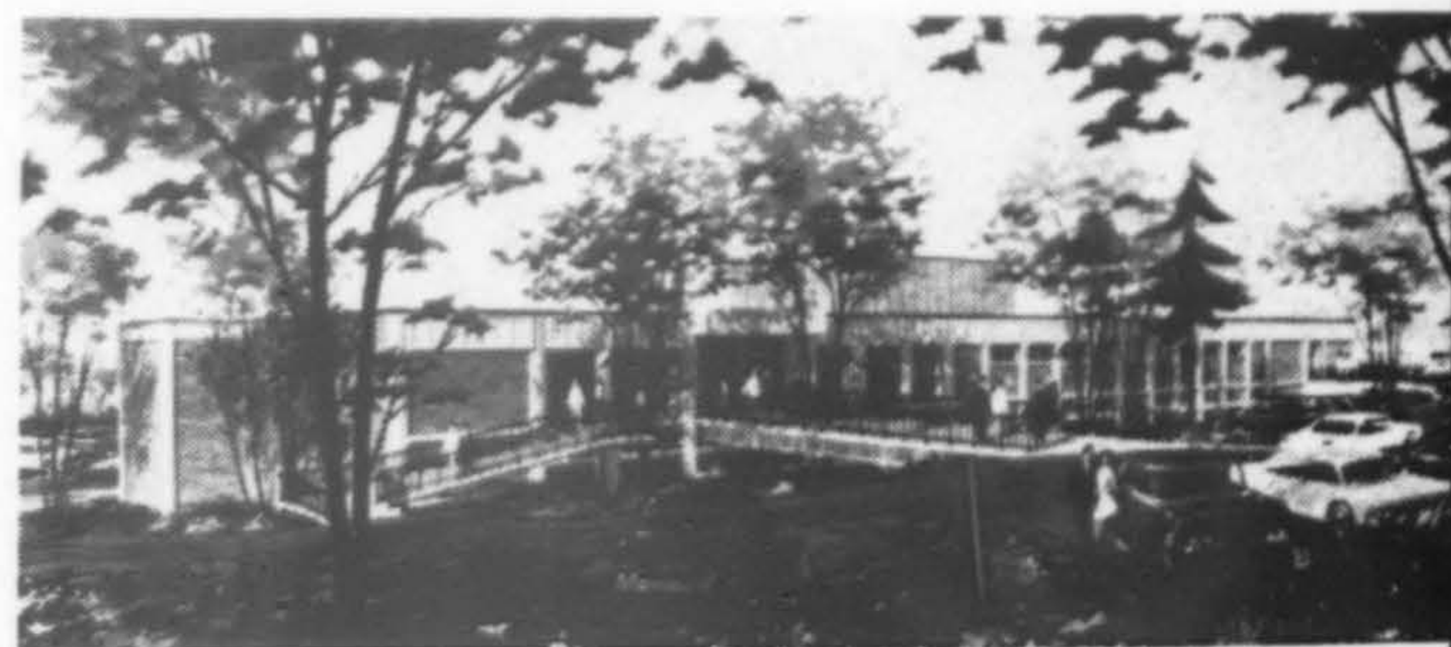
Group Health Cooperative, Renton, Washington, is a two-level reinforced concrete building, sited in a woodsy setting with a view of the valley below. Financed by a Hill-Burton grant, cost is approximately $1,000,000. Architect: George Bolotin.
