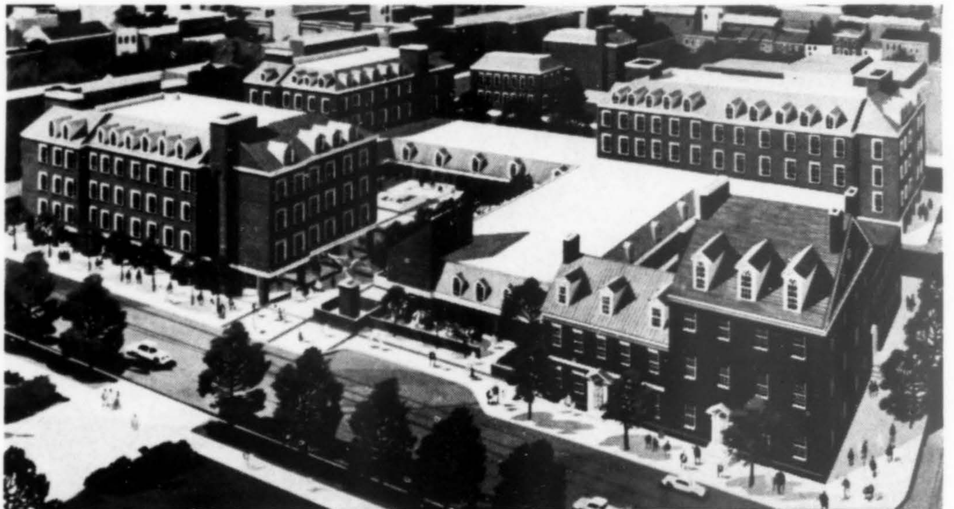
Tavern Square will provide 108,855 square feet of office space, and 63,760 square feet for retail stores. Exterior finish overall is molded brick, of an earthen color, with a rough texture that blends with the weathered look of surrounding buildings.
