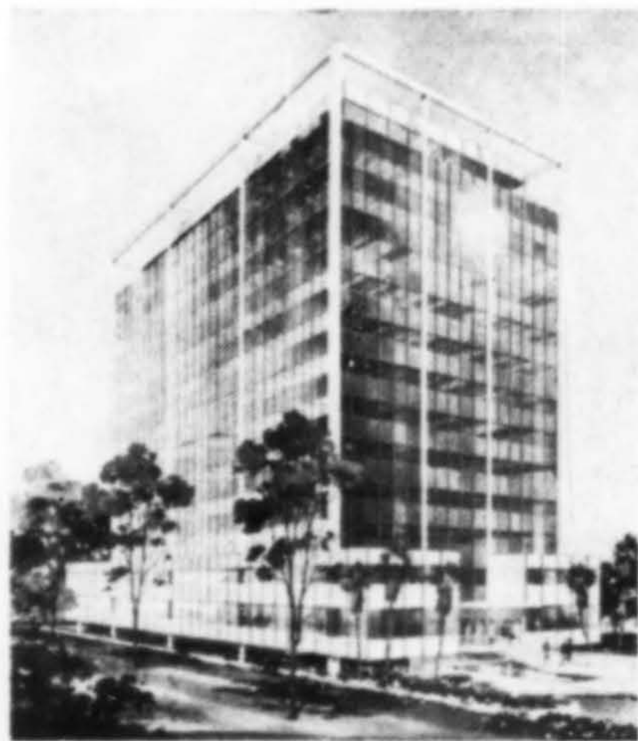
HERITAGE TOWER , a 12-story office building in Anaheim, California, will have a central concrete core with steel box columns at the corners, designed to resist major earthquake or other lateral forces. Interior space is free of columns. Estimated cost: $2,000,000. Architect: Victor Ben-Aziz; Peter Kiewit Sons' Co., contractor.
