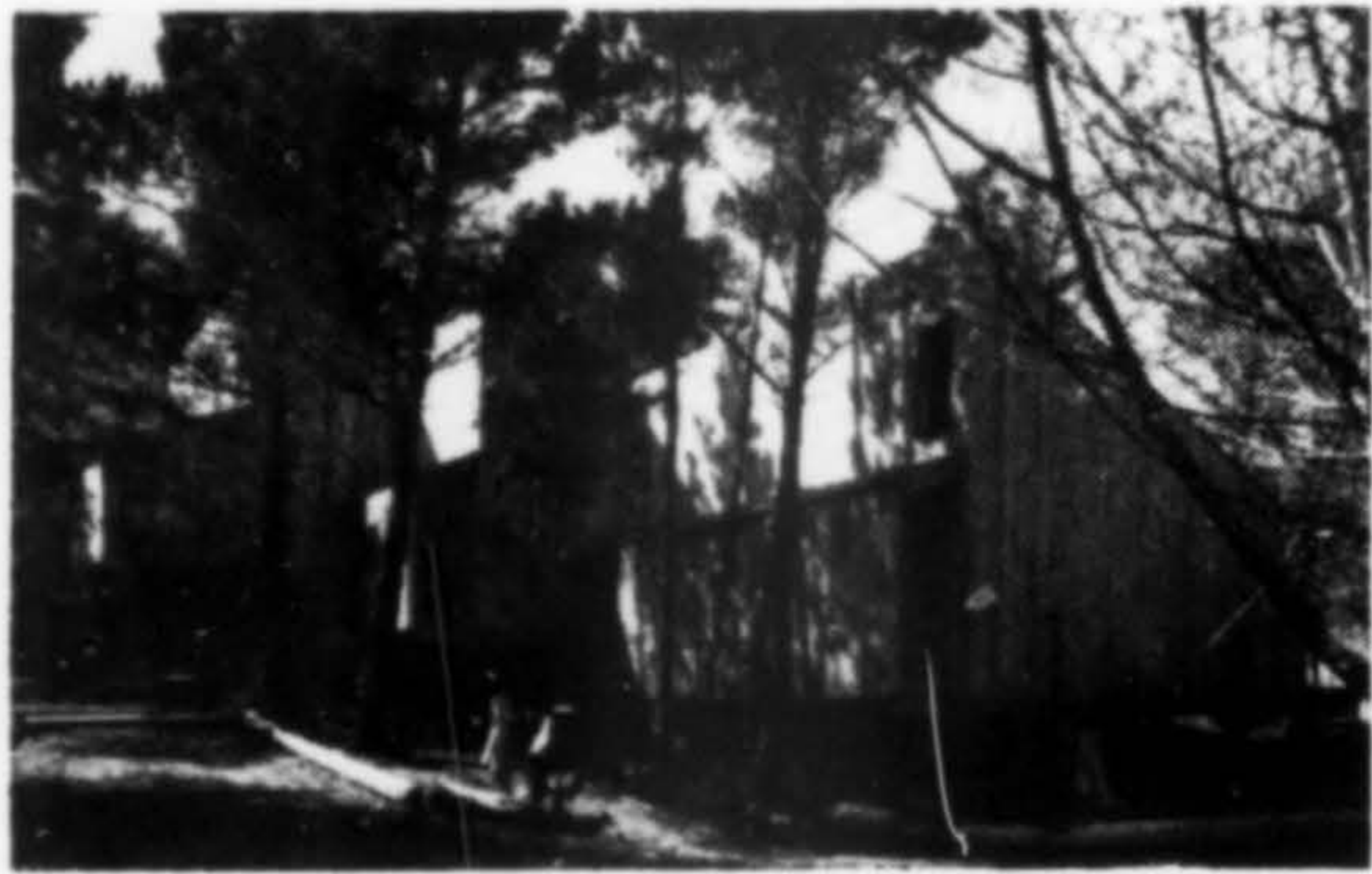
HOUSE IN THE TREES for Salishan Lodge employees, Salishan Beach, Oregon. Honor Award. Church & Shiels, architects.
