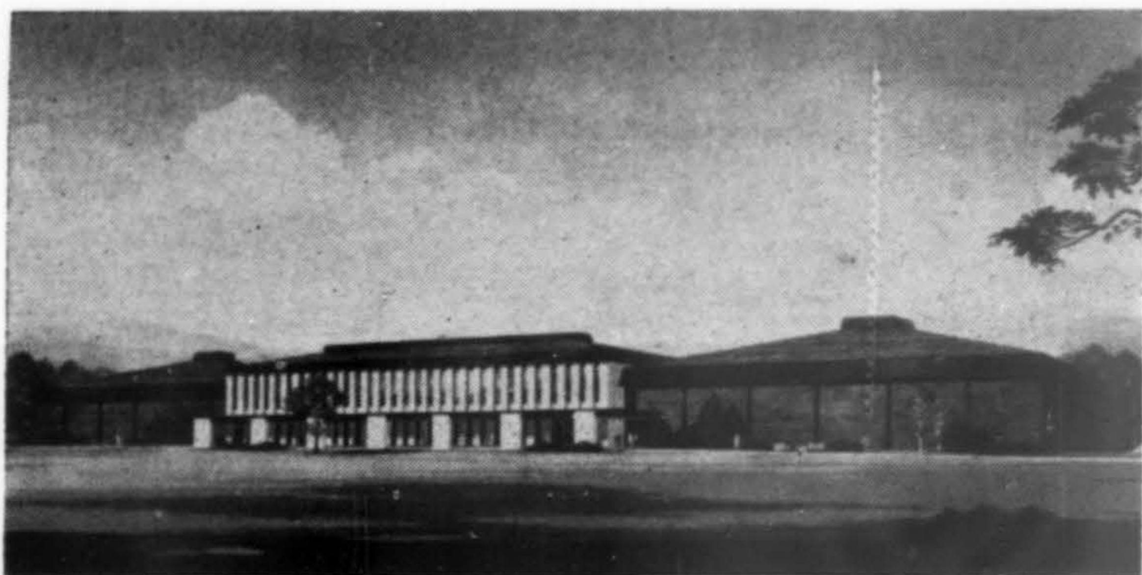
PHYSICAL EDUCATION COMPLEX , Western Montana College, Dillon, Montana, will provide a varsity basketball court, seating for 2,000, practice courts, women's gymnasium, classrooms, offices. Structure will be reinforced prestressed concrete, steel and wood roof. Estimated cost: $900,000. Architects: Eldred F. Moyle & Associates.
